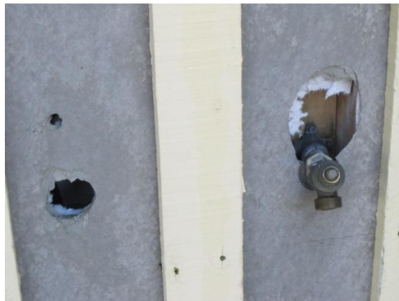
Photo 5: Holes and tap in west wall
