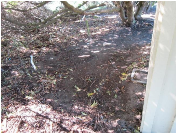
Photo 11: Soil ejecta east of building
