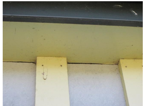
Photo 6: Gaps opening up between timber wall cladding elements
