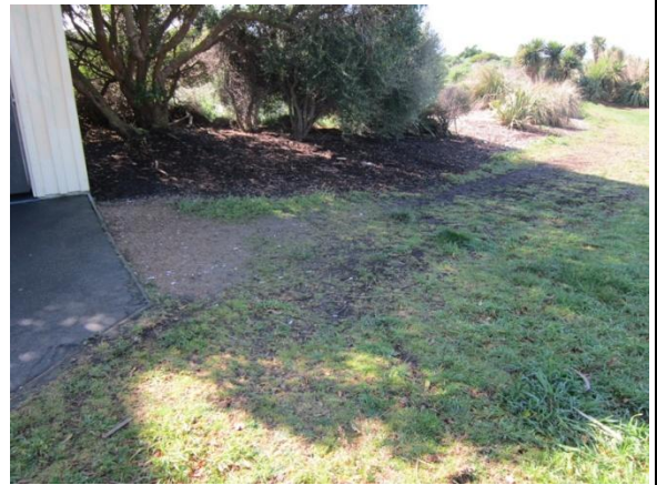
Photo 12: Cracking in the corner of the asphalt west of the building
