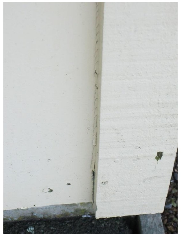
Photo 8: Gaps opening up between timber wall cladding elements
