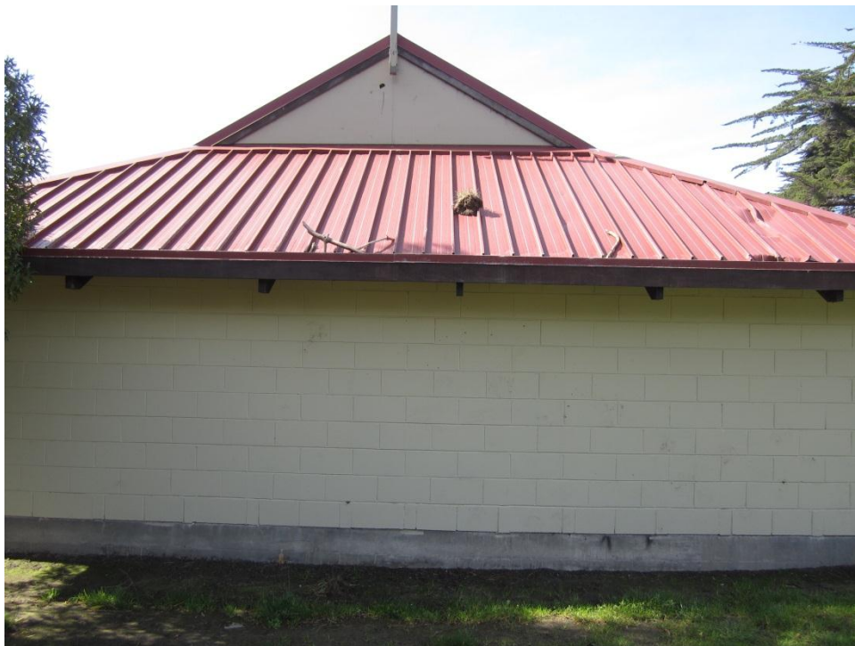
Photograph 5 External concrete masonry wall on north-eastern side of building
