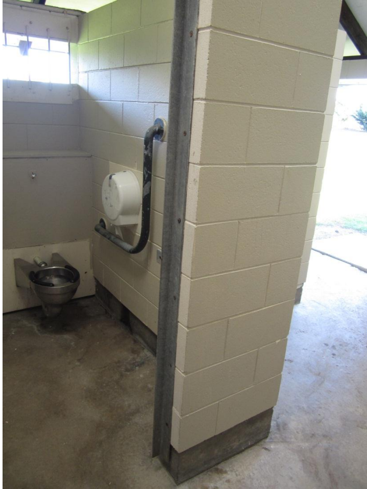
Photograph 3 Internal concrete masonry wall
