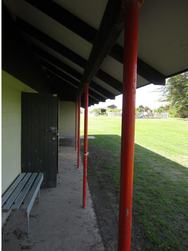
Photograph 7 Steel posts supporting beam and roof trusses
