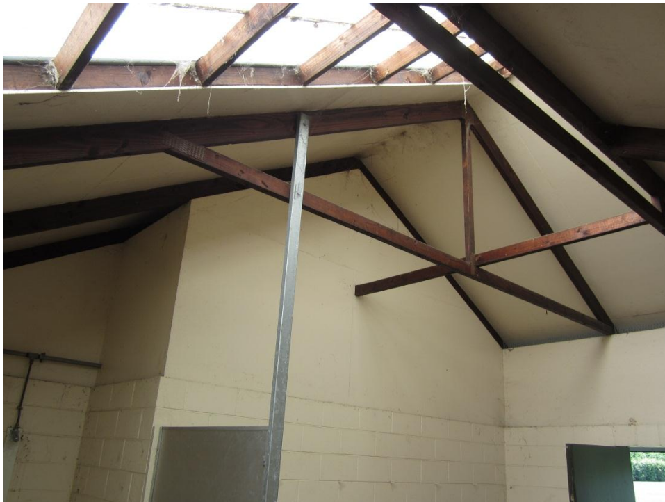
Photograph 8 Vaulted truss
