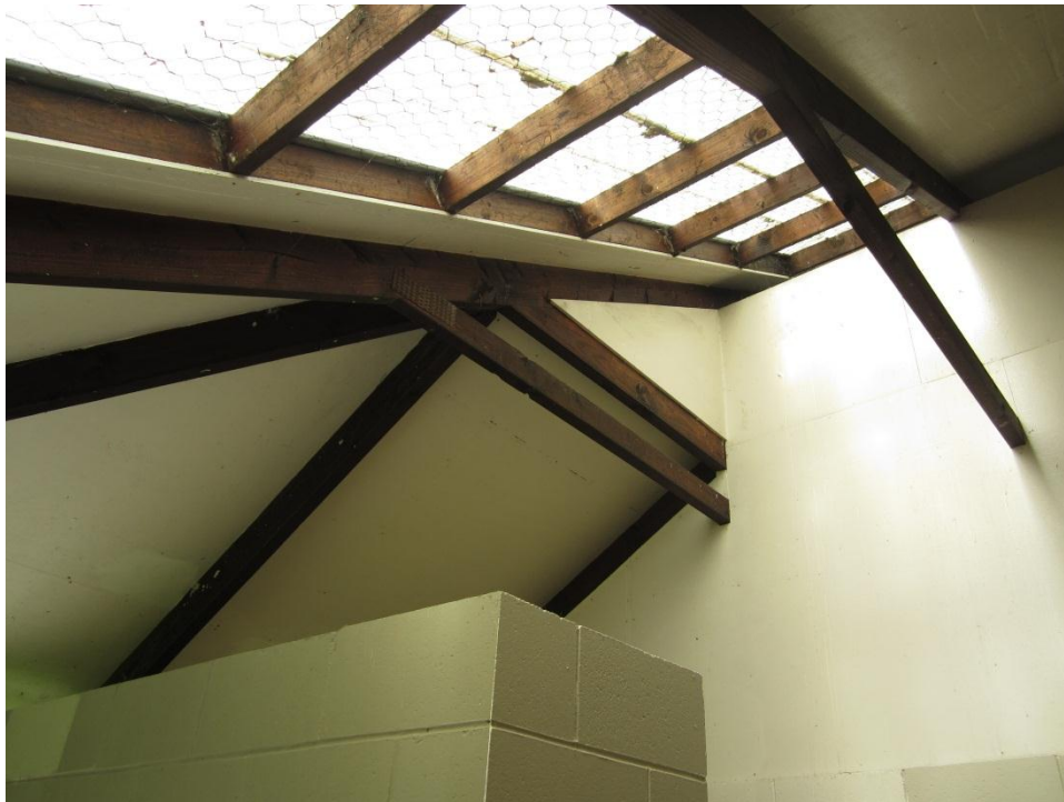
Photograph 4 Unrestrained top edge of internal concrete masonry partition walls
