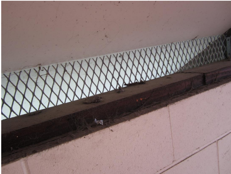
Photograph 9 Hardboard lining to underside of roof purlins
