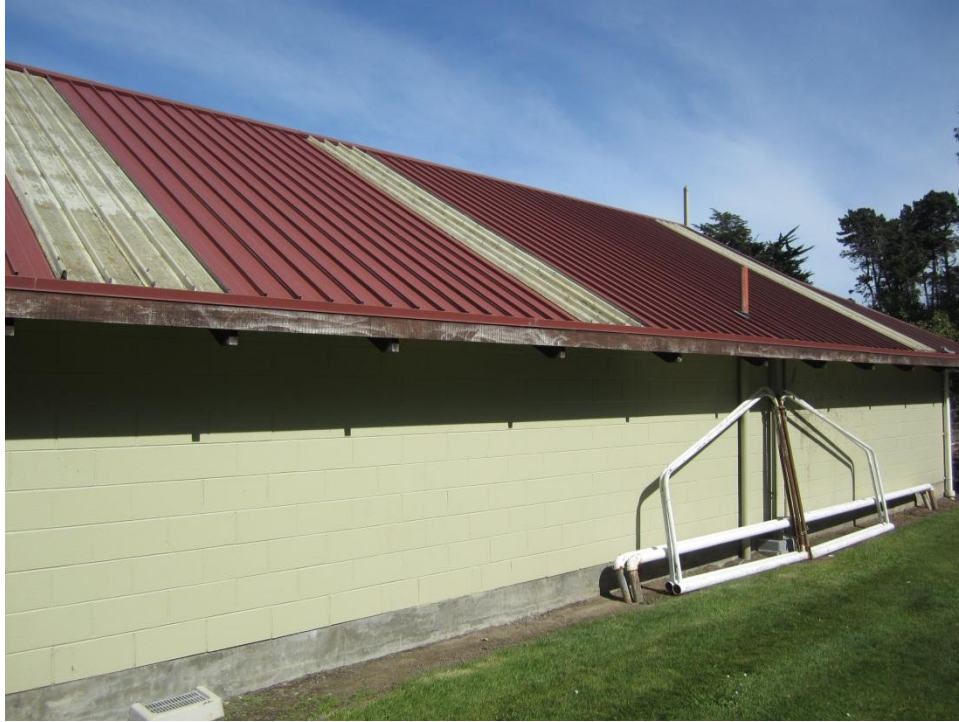
Photograph 5 External concrete masonry wall on north-eastern side of building
