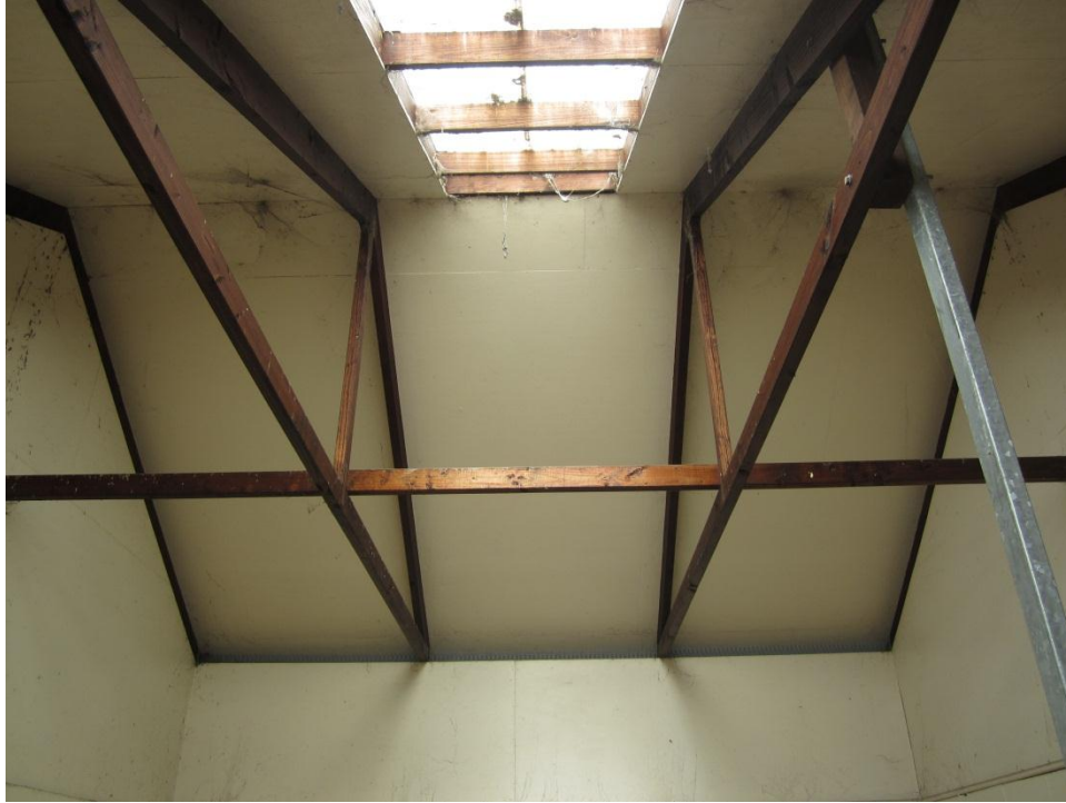
Photograph 9 Hardboard lining to underside of roof purlins
