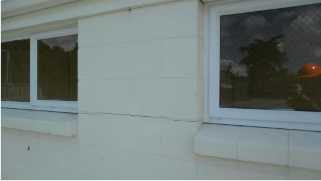
Photo 9: Cracking to reinforced masonry wall at extension area
