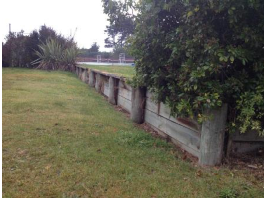
Photo 1: Leaning retaining wall located 7m at north face of the building
