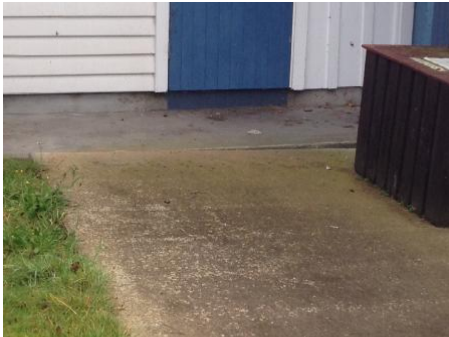
Photo 2: Uneven external concrete pavement
