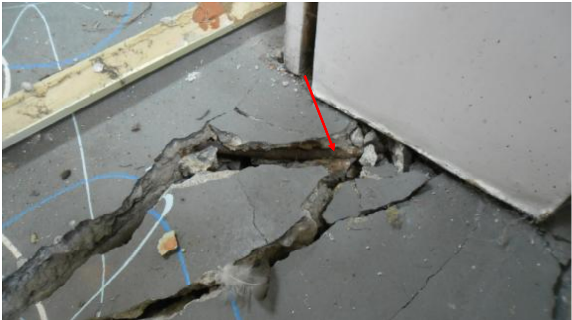
Photo 12: Cracking to concrete floor with exposed reinforcement
