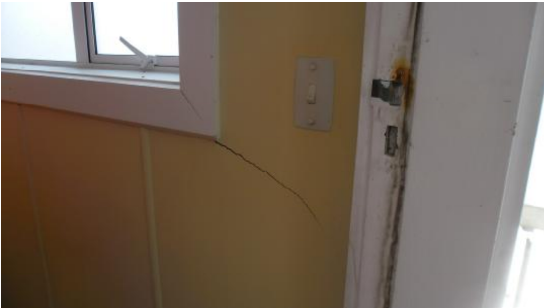
Photo 10: Cracking to non-structural wall lining
