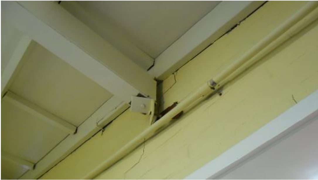
Photo 11: Roof timber connection damage
