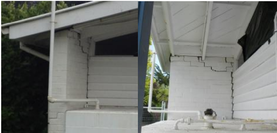
Photo 8: Typical cracking to unreinforced masonry wall
