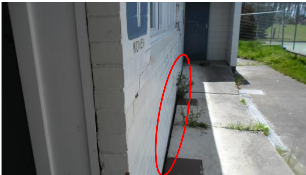
Photo 4: Separation between external pavement and foundation wall
