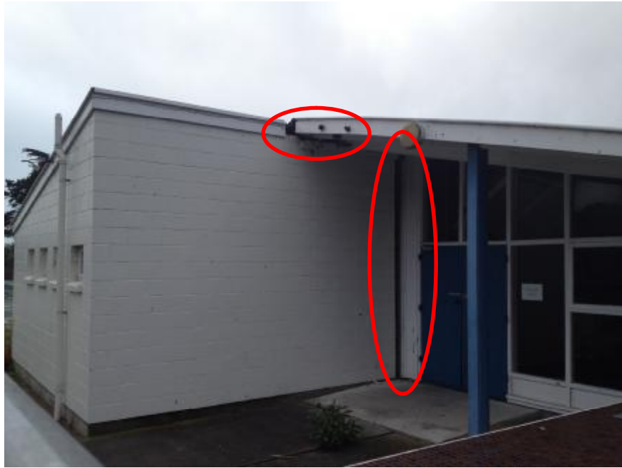
Photo 5: Separation between original and extension area
