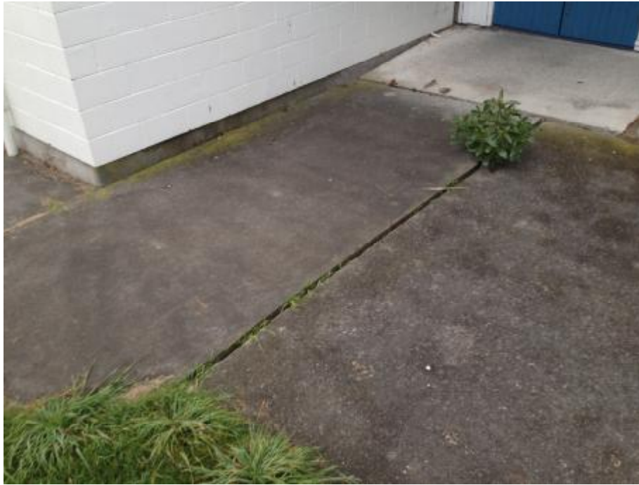
Photo 3: Widened construction joint of external concrete pavement
