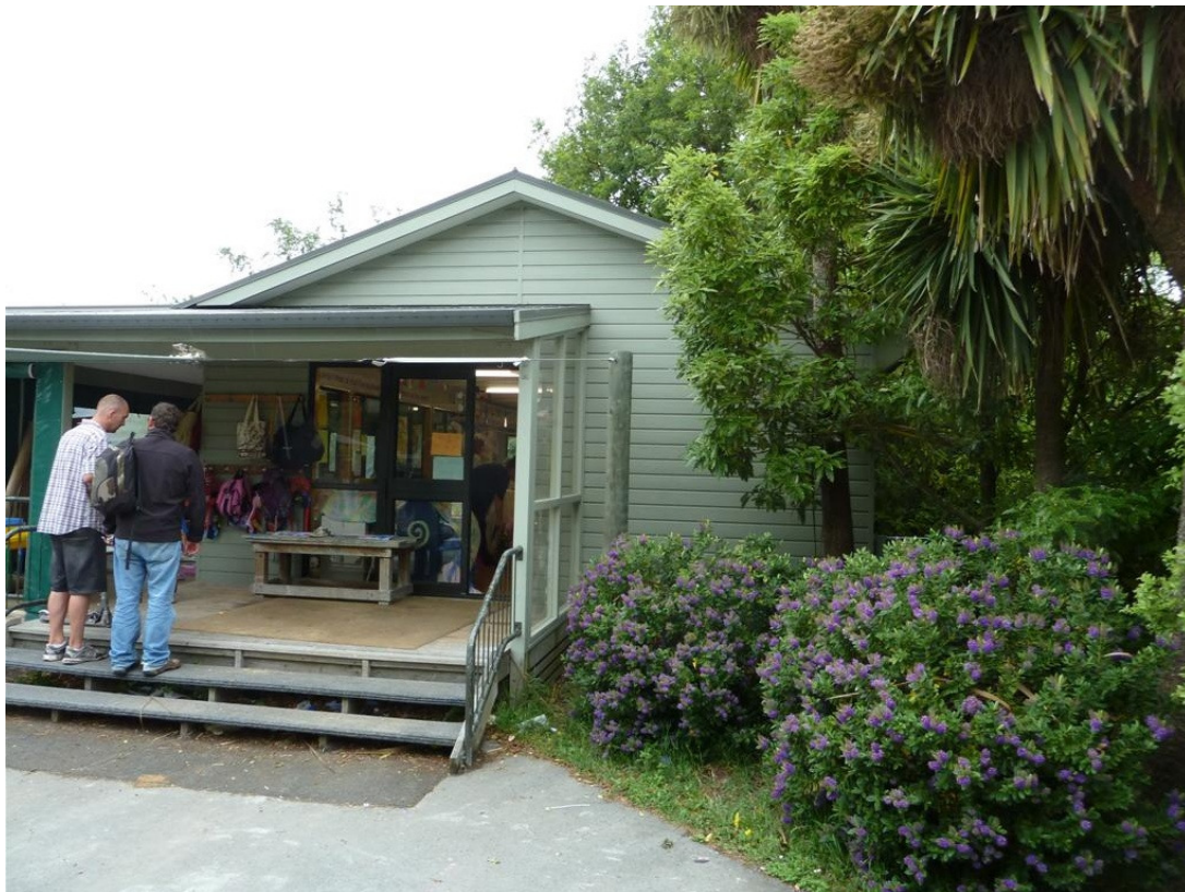
Photo 2 – North-west elevation of building
