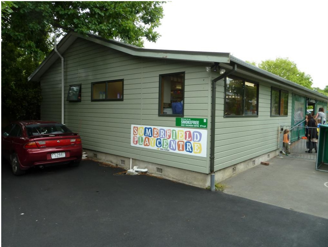
Photo 1 – South-east elevation of building
