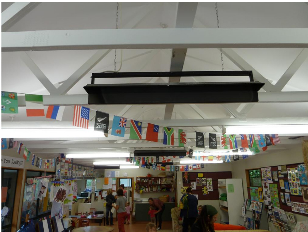
Photo 4 – Exposed truss arrangement in the main play room of the building
