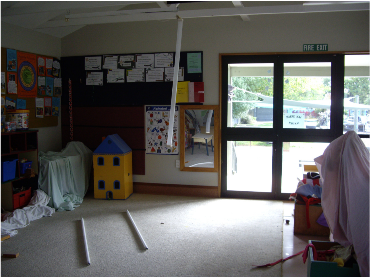
Photo 7 – Internal or overhead lights hanging loose or fallen in the building
