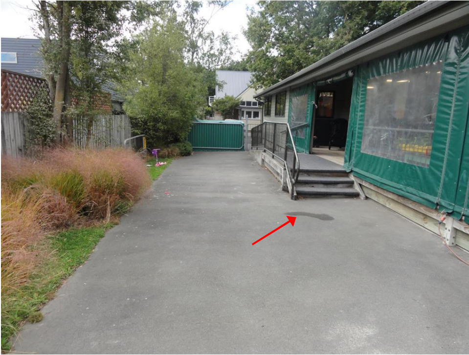
Photo 3: Localised settlement of asphalt (<10mm).
