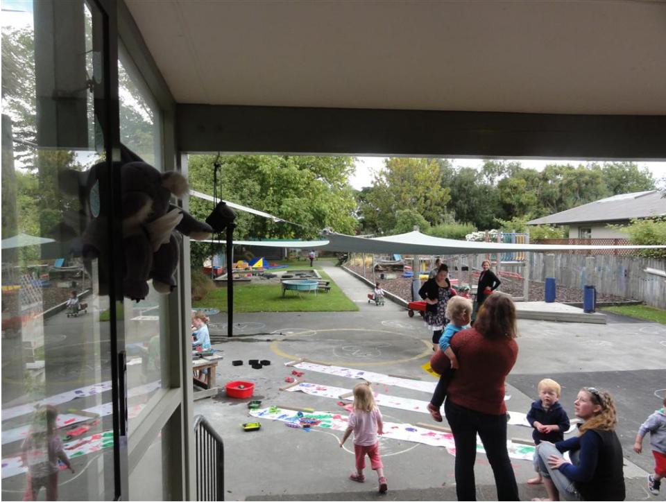
Photo 5: View from rear of building, note uneven asphalt and newly paved areas.
