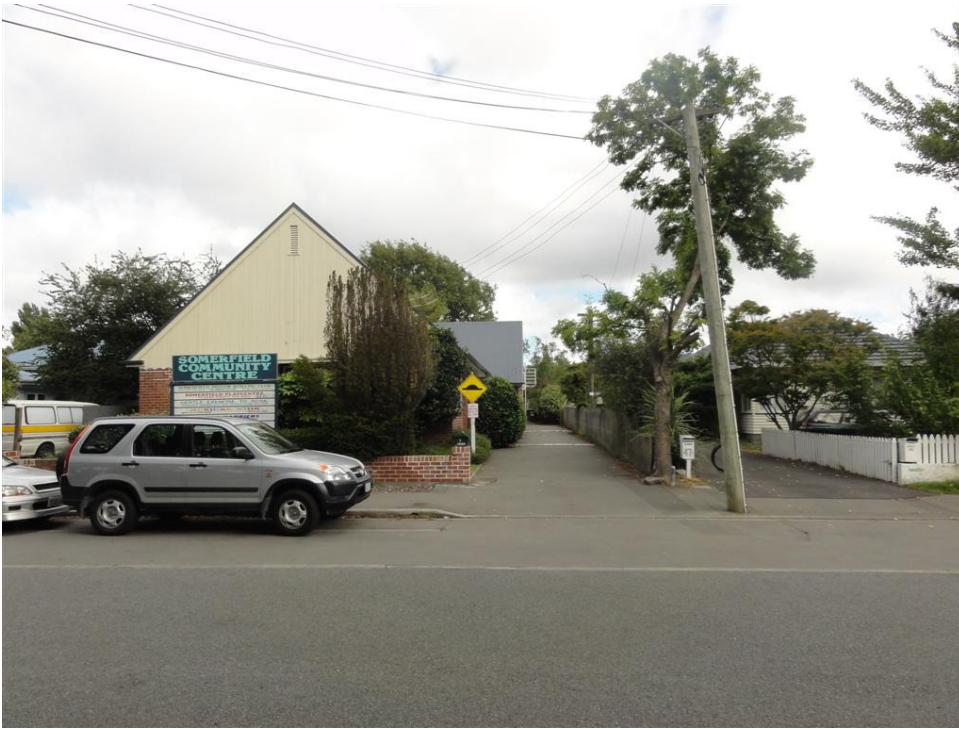
Photo 1: Street elevation, Somerfield Community Centre, 47 Studholme St.
