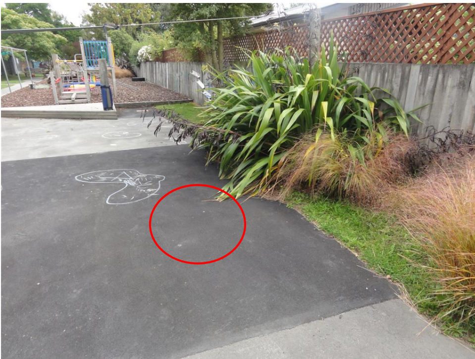
Photo 4: Approximate location of liquefaction on site (0.25m 2 ), note new asphalt.
