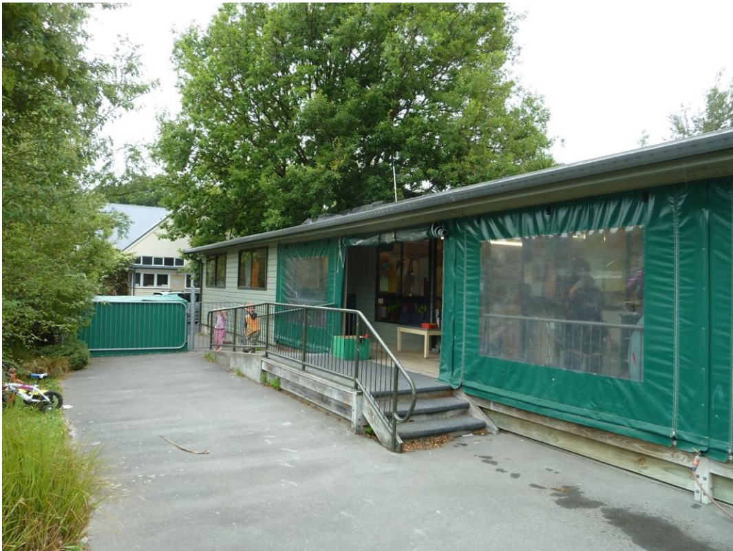
Photo 3 – North-east elevation of building
