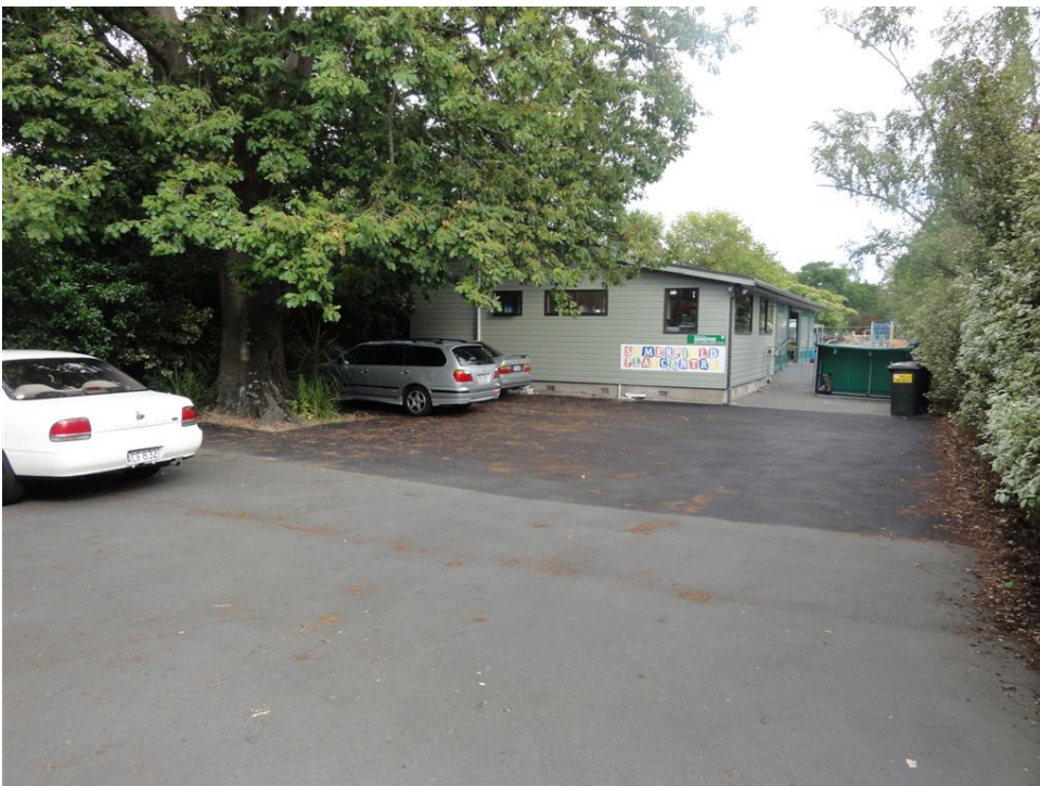
Photo 2: Playcentre down driveway, behind community centre. Note new asphalt.
