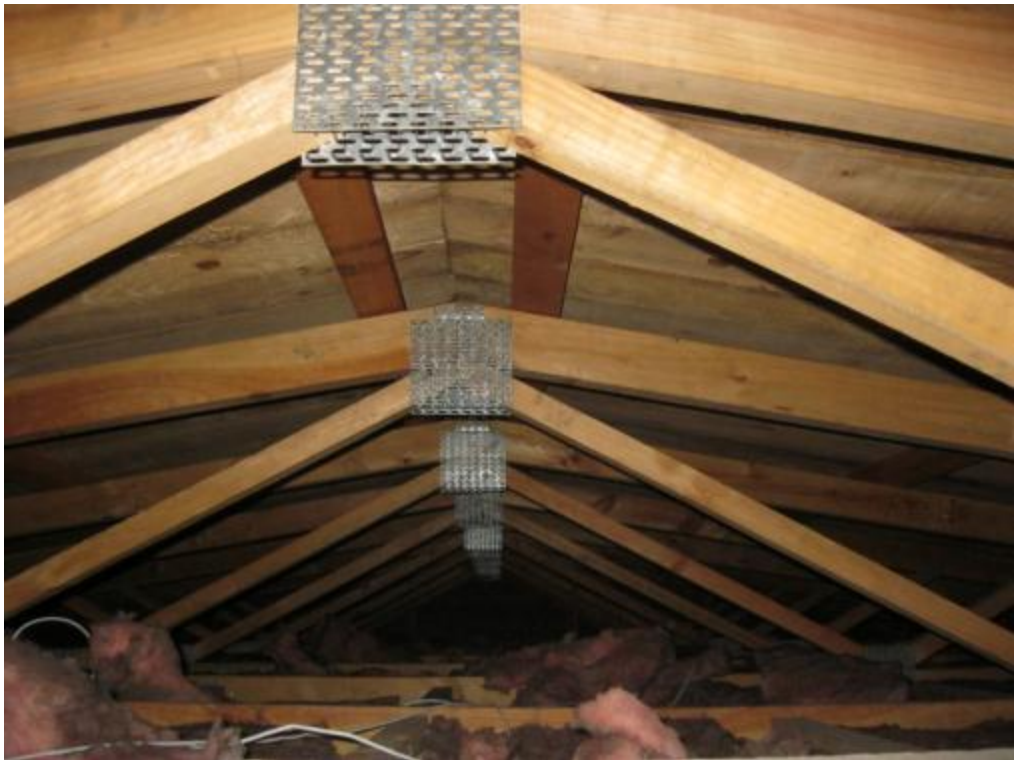
Photograph 12: Timber truss roof in section four with timber sarking
