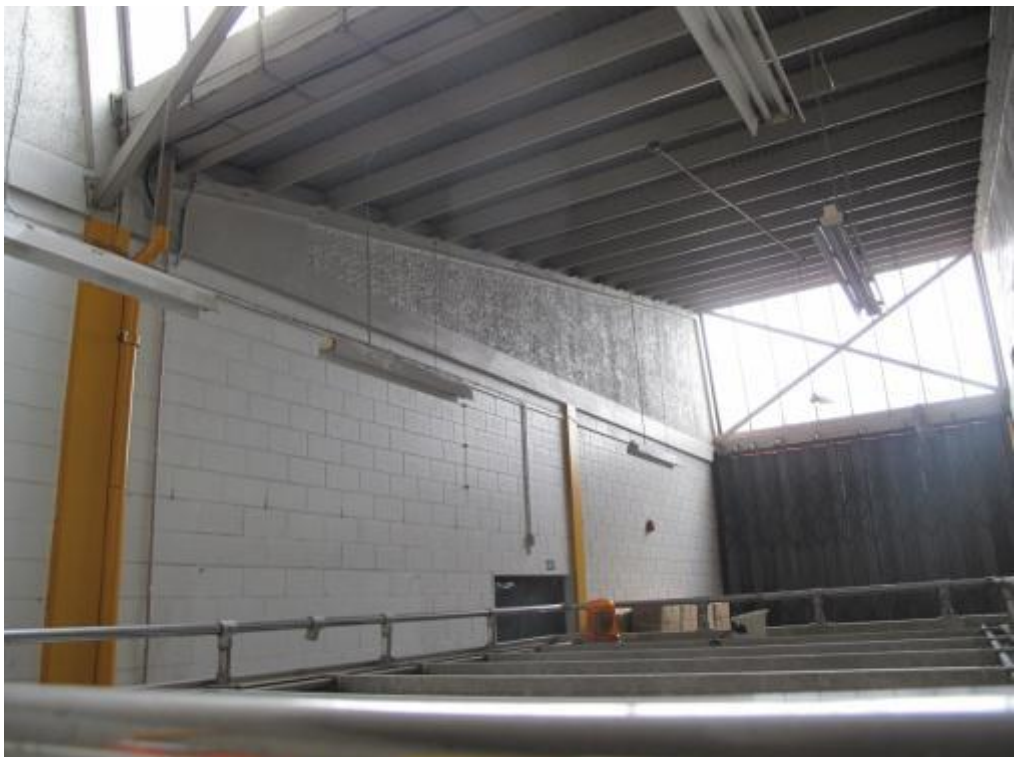
Photograph 10: Section three has SHS diagonal sections acting as compression/tension members to transfer load, no strap bracing is present
