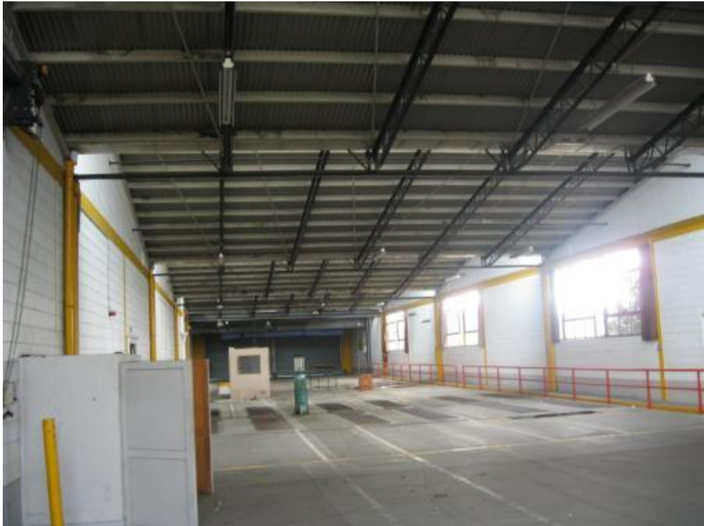
Photograph 5: Interior structure of Section two showing concrete frame structure with infill masonry
