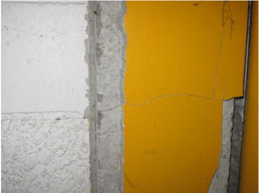
Photograph 11: Cracking and spalling of concrete at column base
