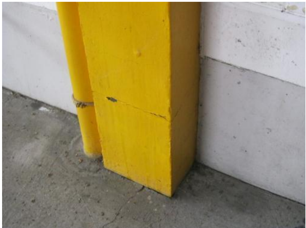
Photograph 8: Cracking at the base of the column indicates bending and movement
