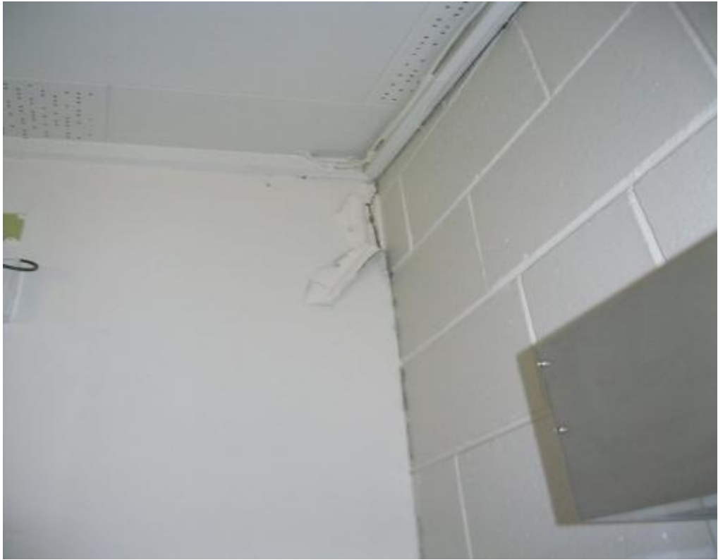
Photograph 3: Separation between masonry blockwork and timber framed walls to Section one
