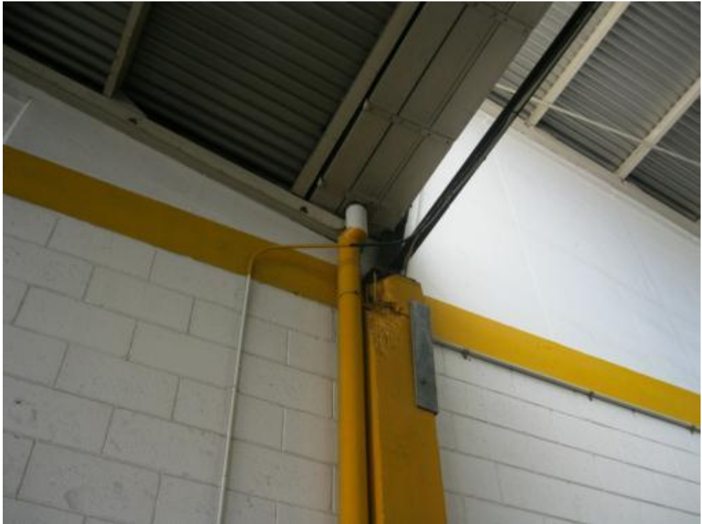
Photograph 7: Cracking and spalling of the concrete has occurred at the connection between the roof steel beams and the top of the concrete column
