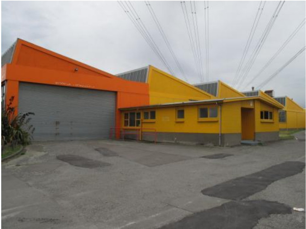
Photograph 1: East elevation showing Sections one and two
