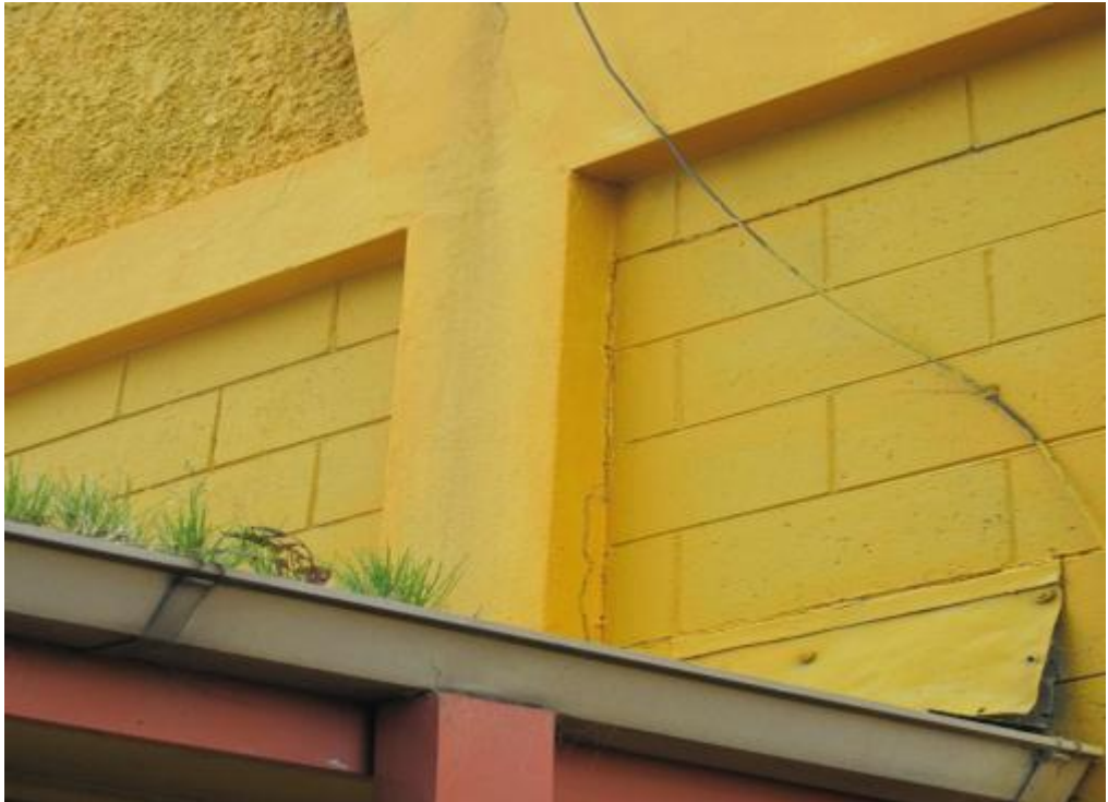
Photograph 9: Externally cracking is evident to the concrete column and masonry blockwork
