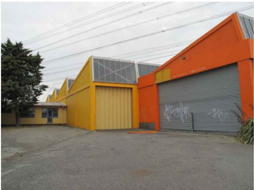
Photograph 2: South elevation showing Sections two, three and four
