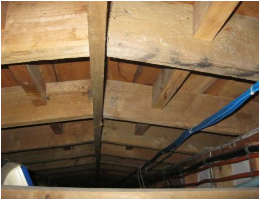
Photograph 4: Timber framed roof with timber sarking to Section one
