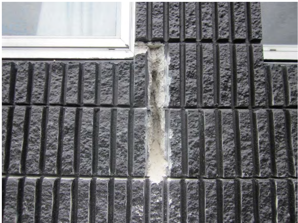
Photograph 29 Opening up works at crack location below concrete masonry column. No reinforcement was observed.
