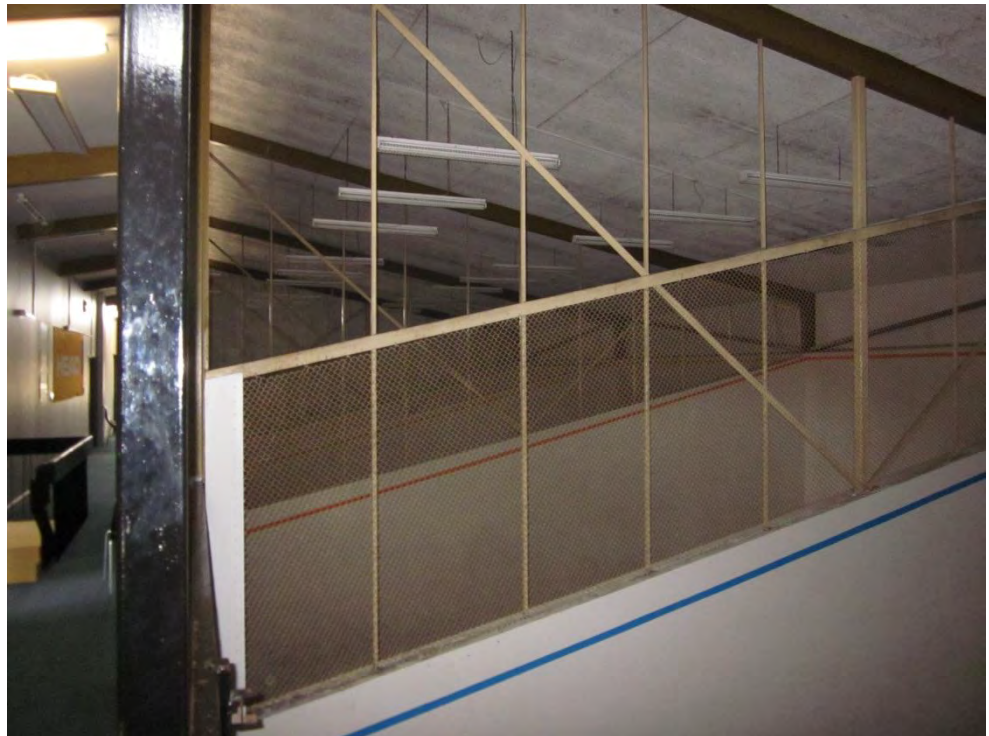
Photograph 25 Bracing in each portal frame bay with masonry infill
