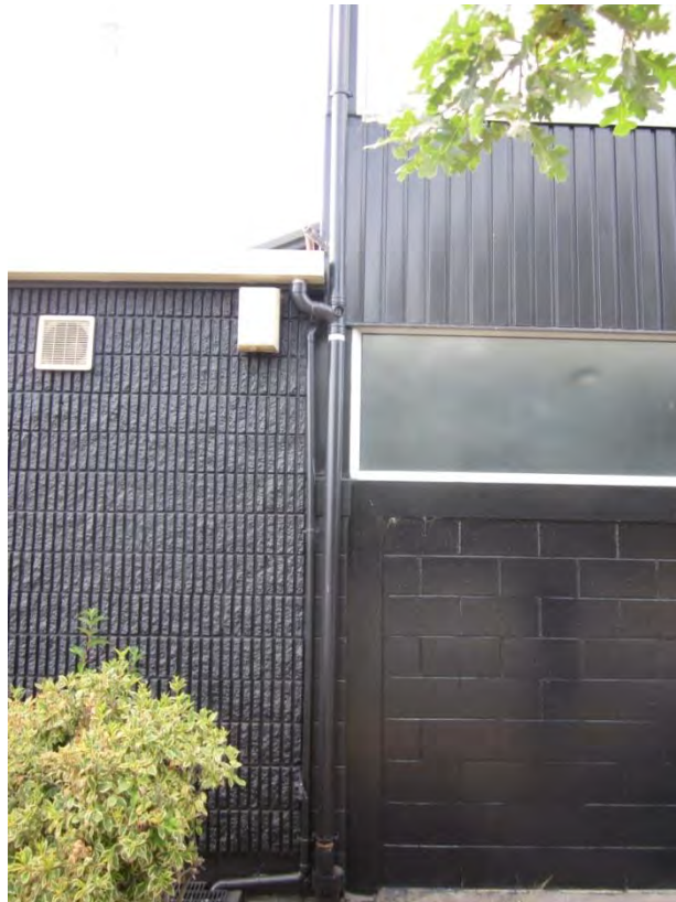
Photograph 7 Connection between original structure and subsequent addition
