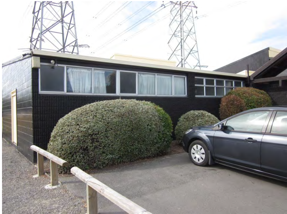
Photograph 2 View from the north of the administration area
