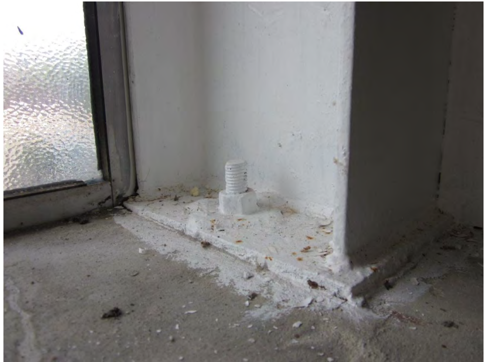
Photograph 24 Steel portal frame base connection
