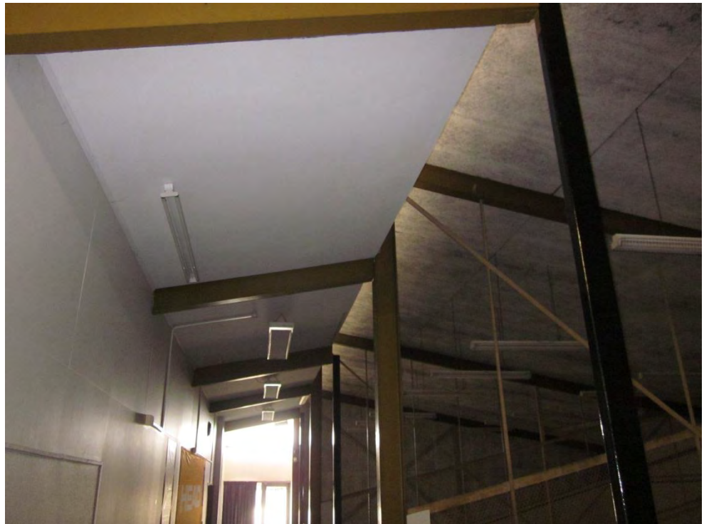
Photograph 27 Rafter to portal frame connections
