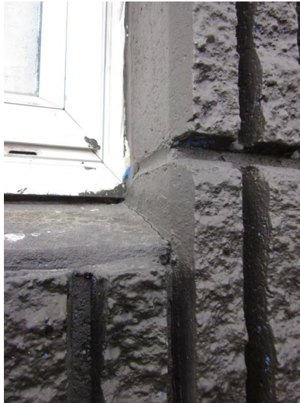
Photograph 5 Cracking at the edge of the window between the column and concrete masonry wall on the front face of the building
