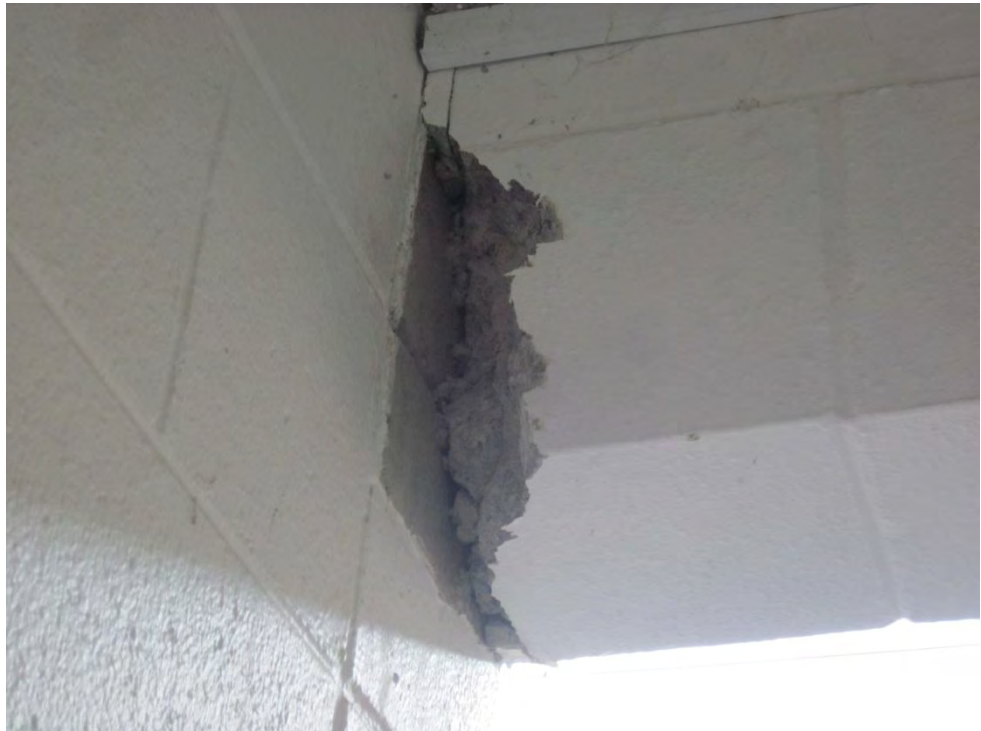
Photograph 31 Opening up works undertaken at location of cracking around connection between original structure and addition. No reinforcement was observed.
