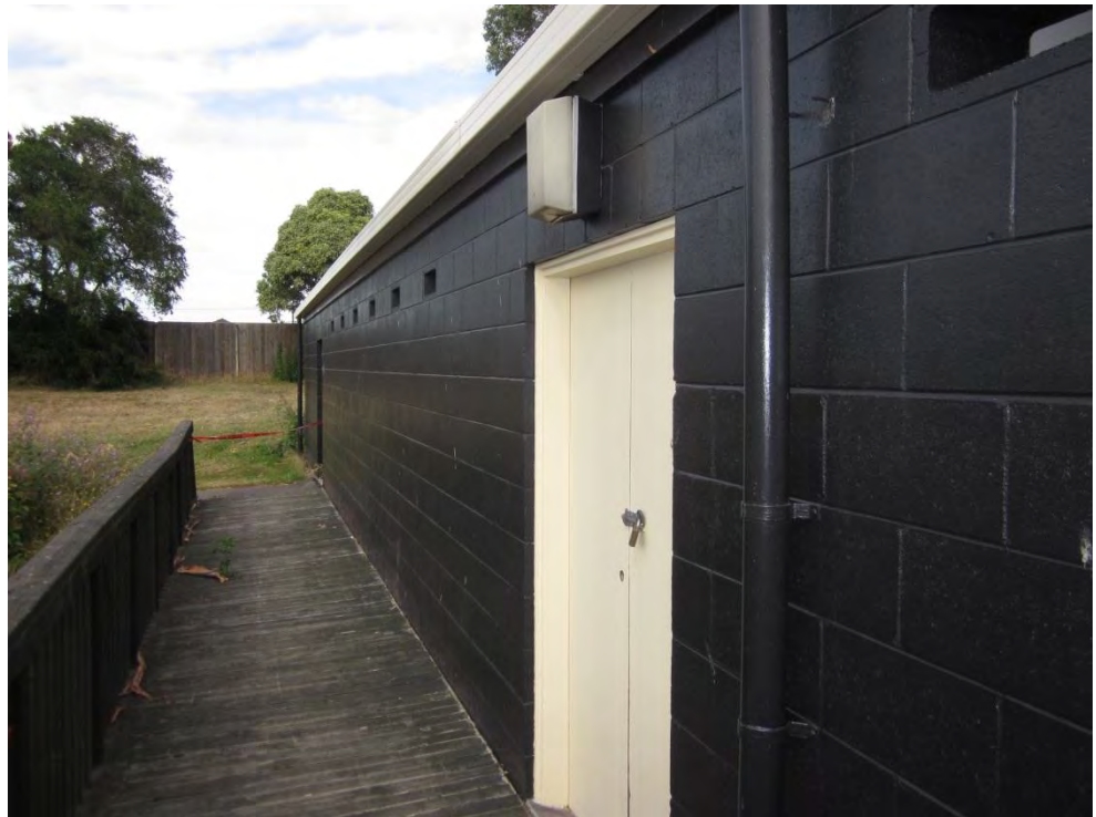
Photograph 11 Timber deck and changing rooms at rear of building
