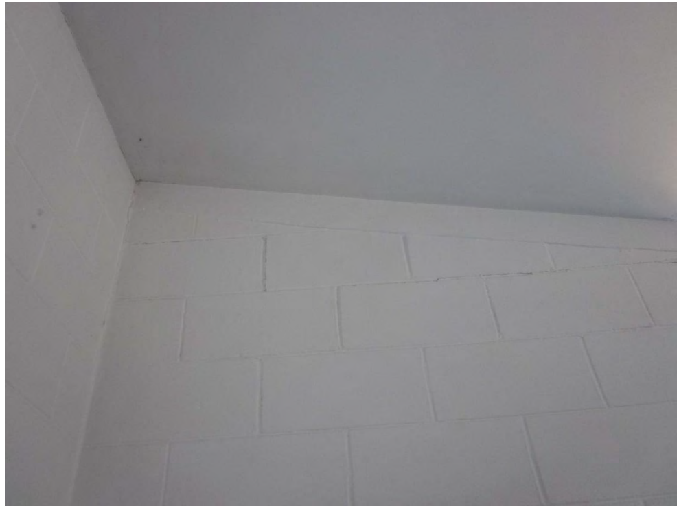
Photograph 26 Cracking on the south-western wall of second story
