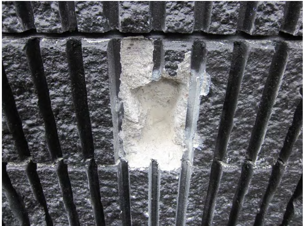
Photograph 28 Opening up works at crack location on left side of front face of the building. No reinforcement was observed.
