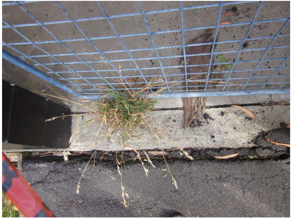
Photograph 12 Cracking of asphalt footpath where ground appears to have slumped
