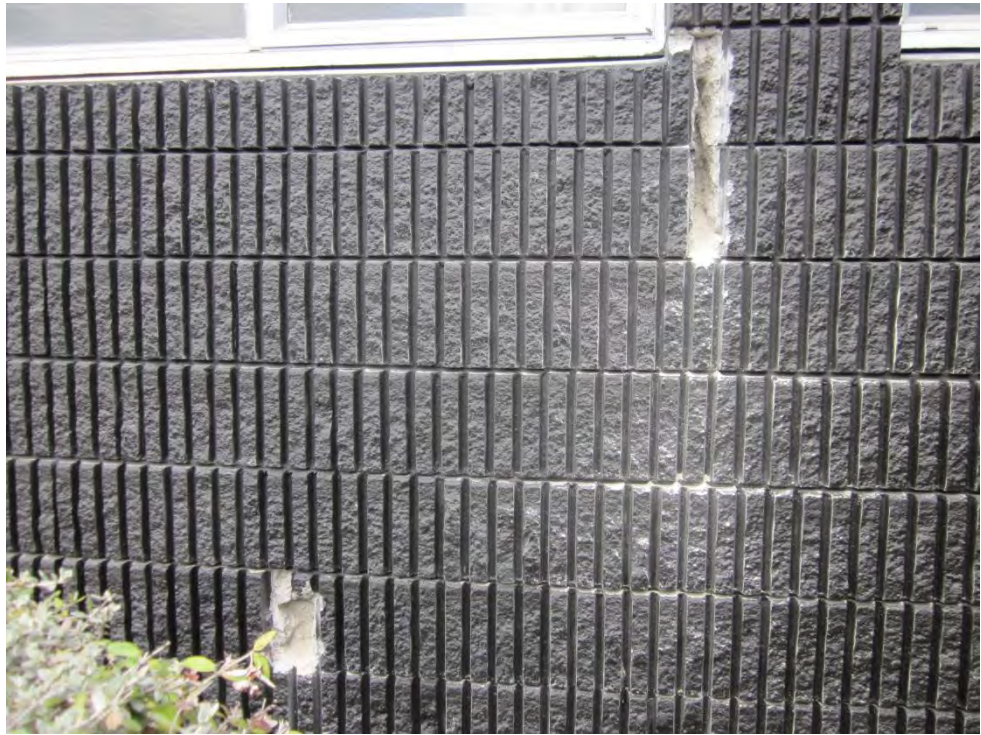
Photograph 30 View of external opening up works undertaken
