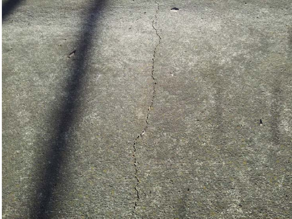
■ Figure 8 - Cracking in external concrete slab
