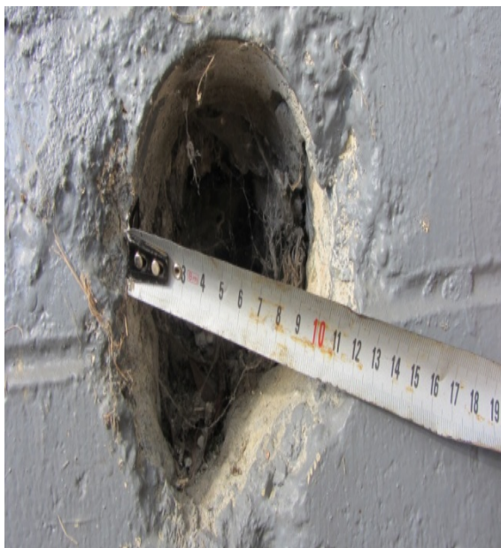
Photo 15: Close up view of 100mm diameter hole
