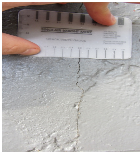
Photo 16: Close up view of vertical crack
