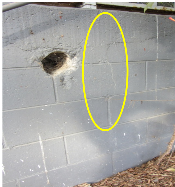
Photo 14: Masonry retaining wall with 100mm diameter hole, and vertical crack alongside.
