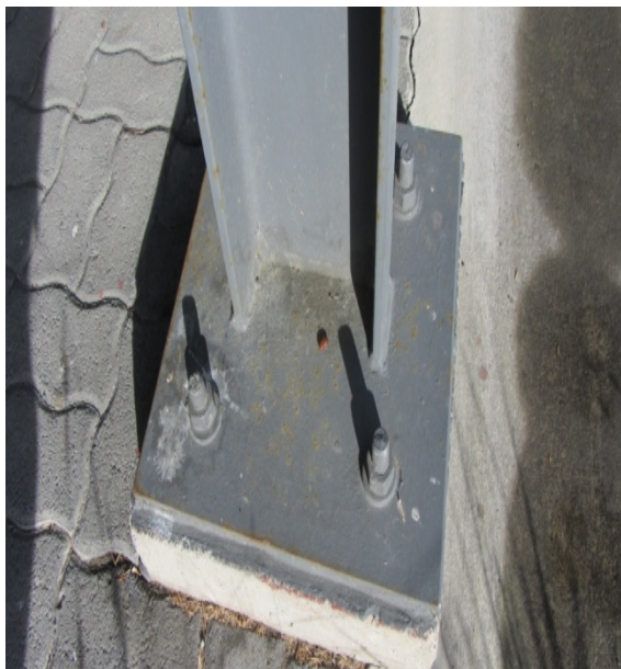
Photo 13: Close up view of foundation pad connection
