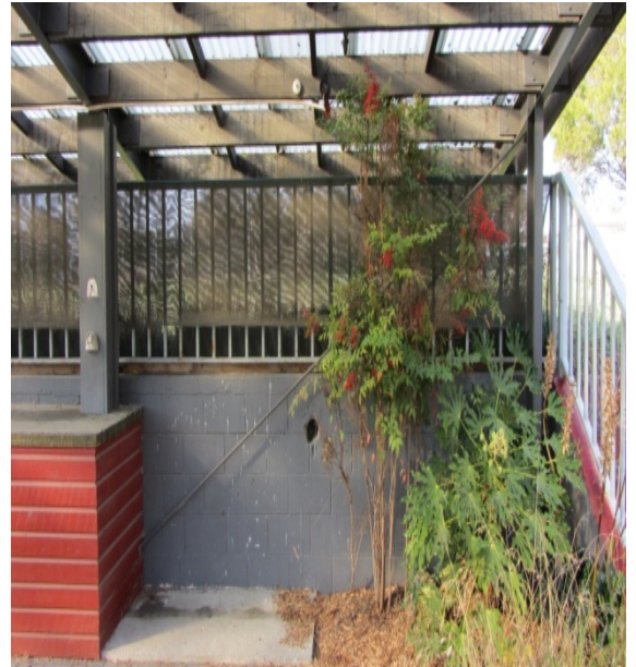
Photo 6: North elevation, close up view of west
