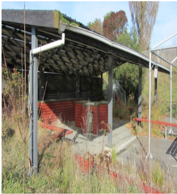
Photo 9: View along north elevation
