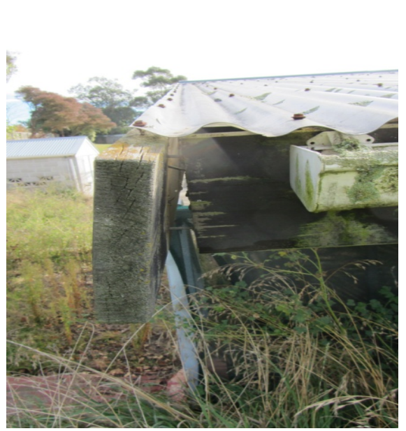
Photo 18: loose timber connection in roof framing
