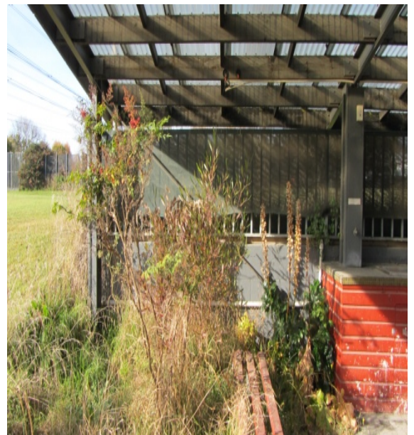
Photo 8: North elevation, close up of east bay
