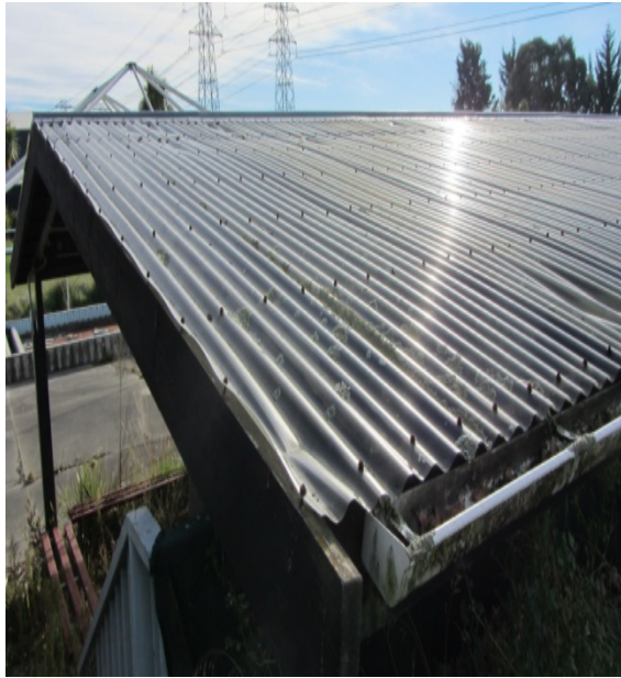
Photo 17: View of translucent roof cladding.
