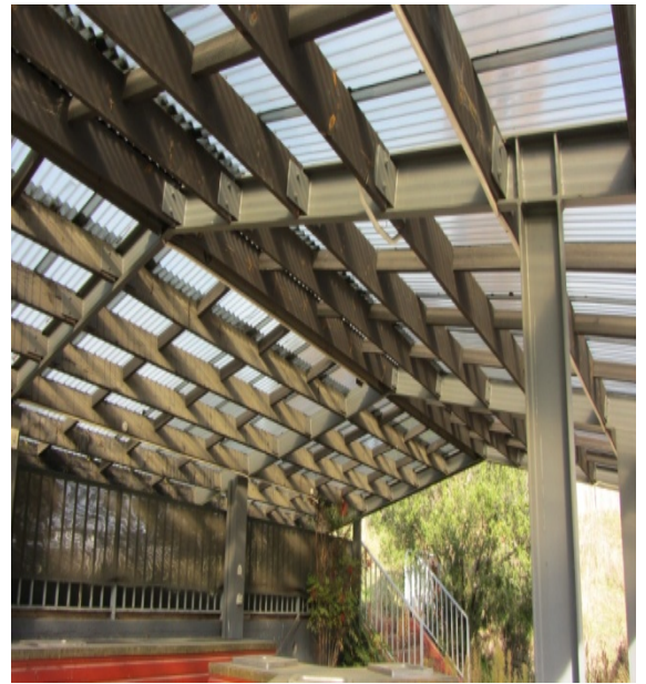
Photo 10: View of roof framing
