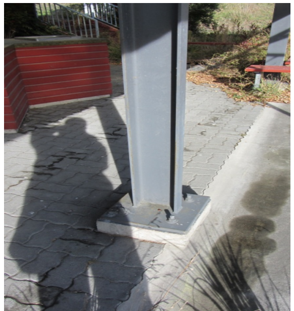
Photo 12: Foundation pad connection
