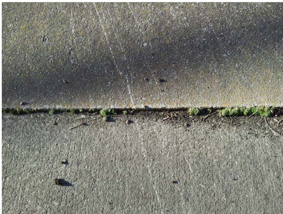
■ Figure 9 – Observed differential settlement of external concrete slabs
