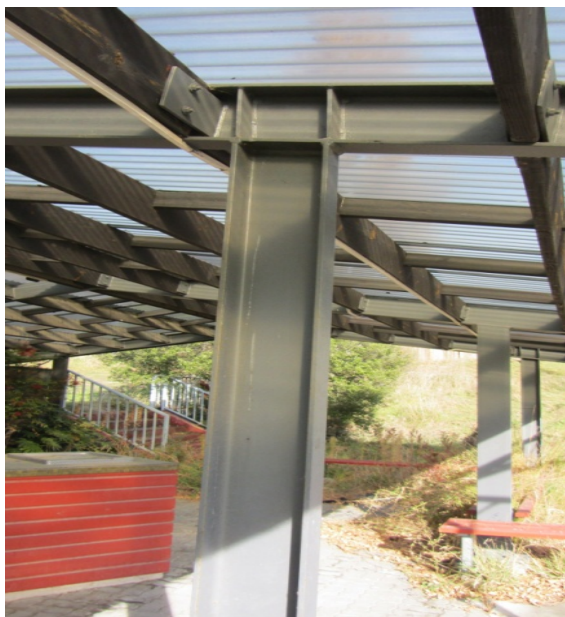
Photo 11: Steel column and rafter connection
