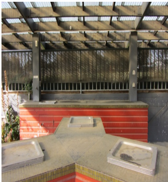
Photo 7: North elevation, close up view middle bay
