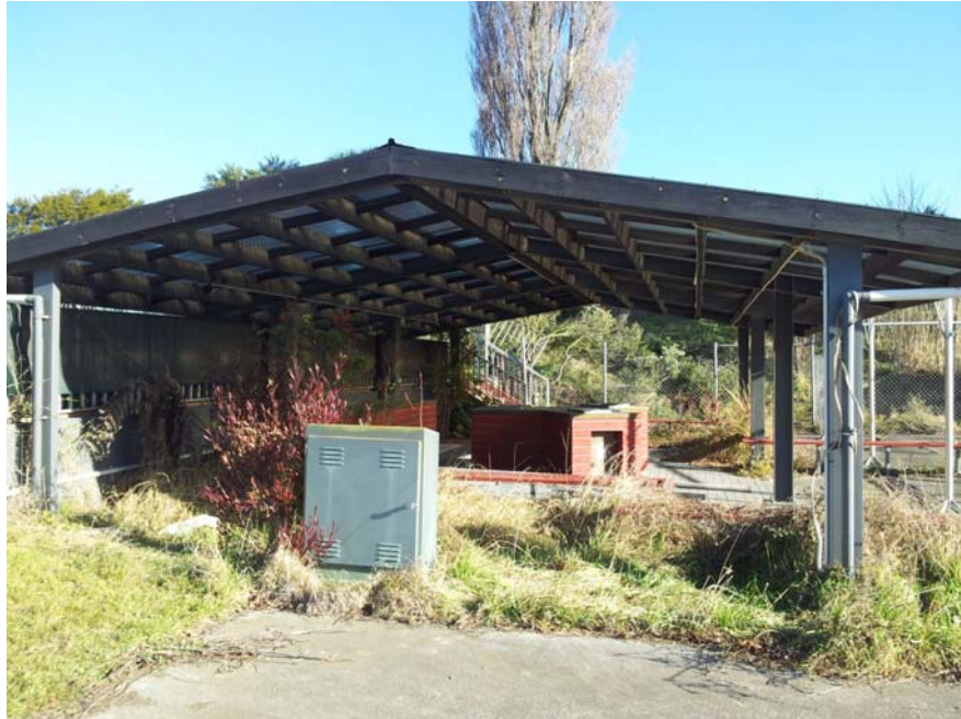
■ Figure 6 - Overview of the structure (eastern elevation)
