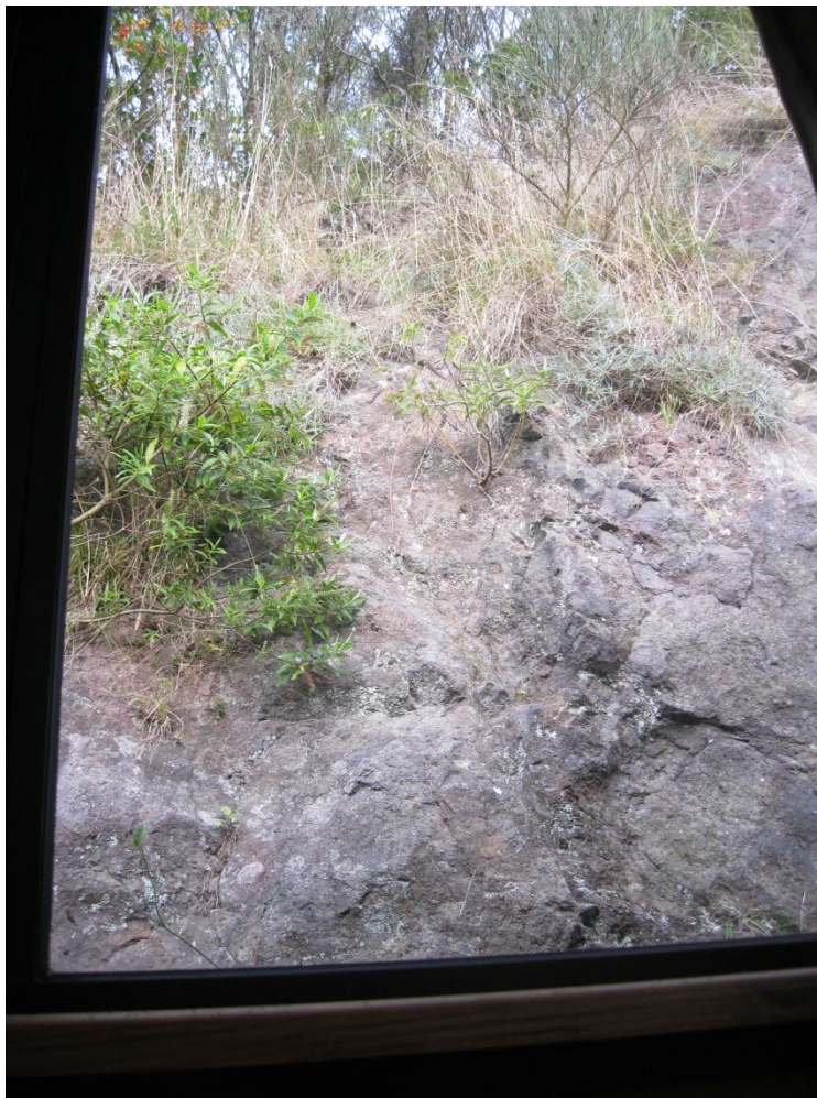
Photograph 4 View of cut face from interior.
