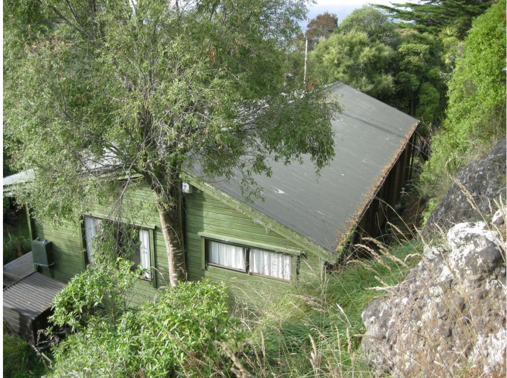
Photograph 3 View from slope above(Potential rockfall hazard in foreground).
