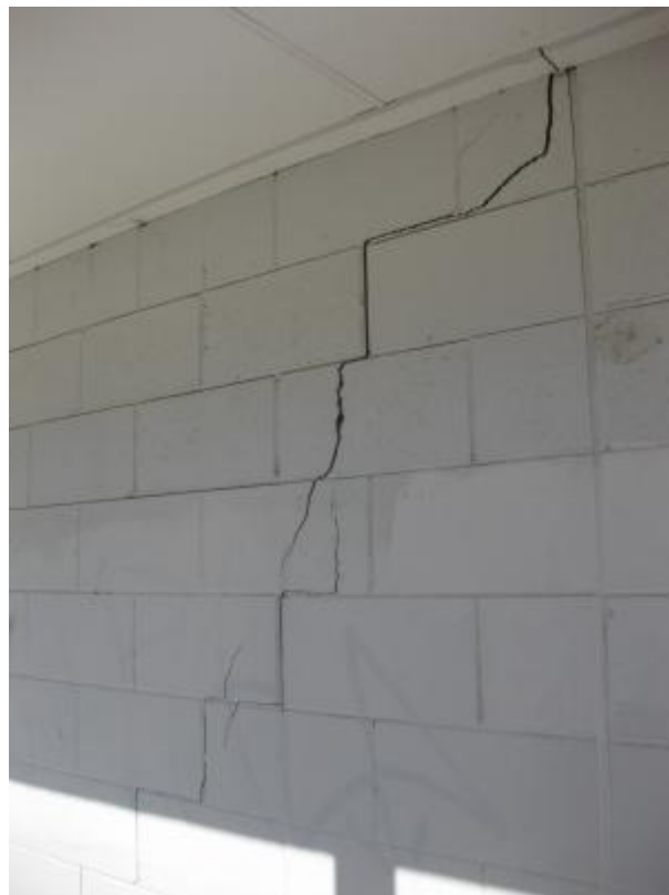
Photo 6: Crack in the front wall
