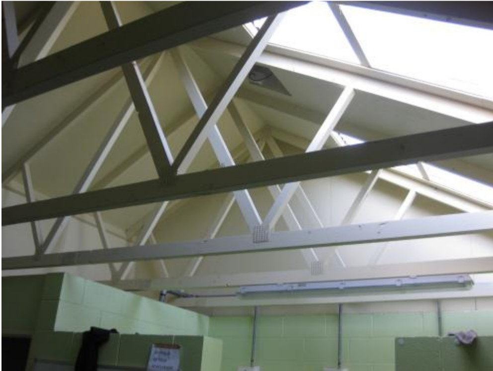
Photo 9: Roof truss and lining
