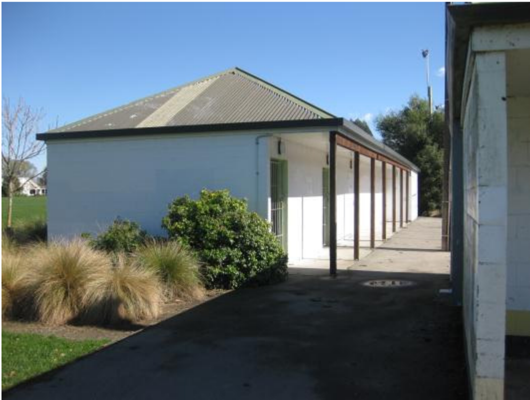
Photo 1: View of the building from east
