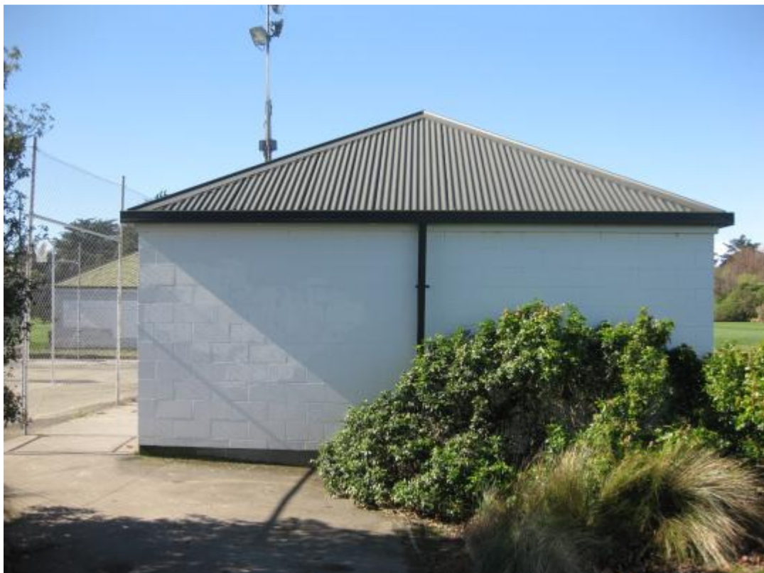
Photo 4: View of the building from west
