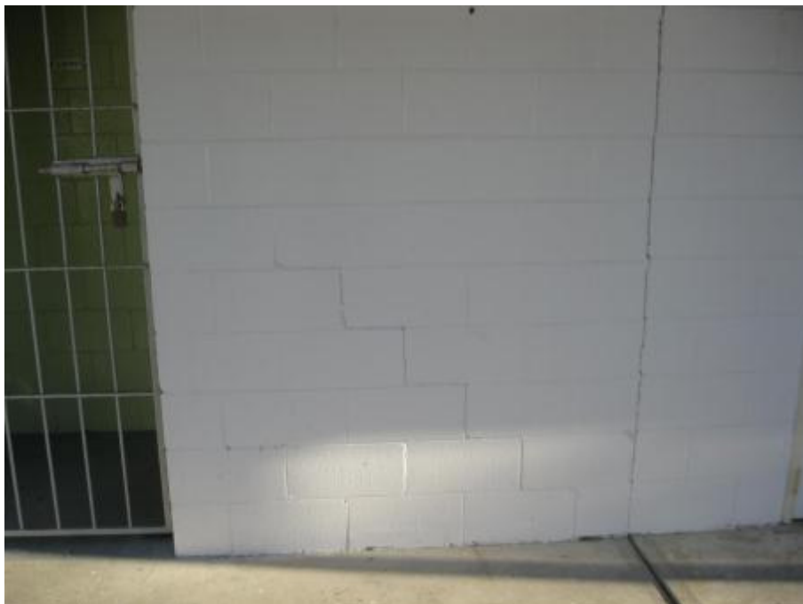
Photo 8: Diagonal crack in the front wall
