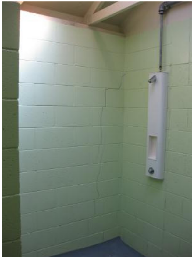
Photo 10: Diagonal crack in the back side wall from inside
