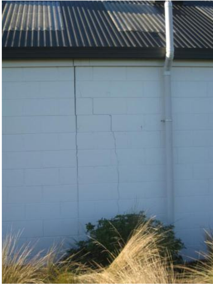
Photo 7: Crack in the rear wall
