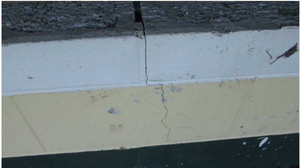
Cracking to blockwork.
