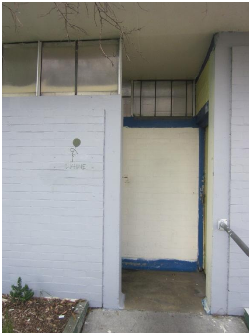
Photo 11: Entrance to womens toilet
