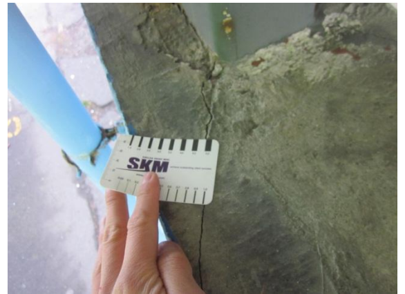
Photo 18: View of RHS column northwest corner (3) showing 1mm crack
