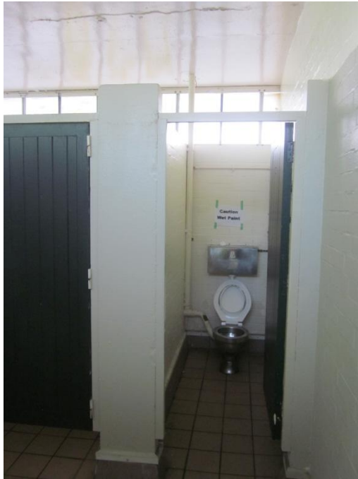
Photo 9: Interior of mens toilet (3)
