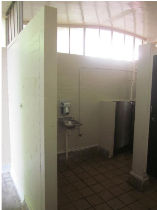
Photo 7: Interior of mens toilet (1)
