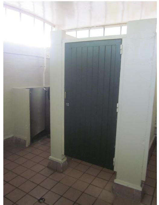
Photo 8: Interior of mens toilet (2)
