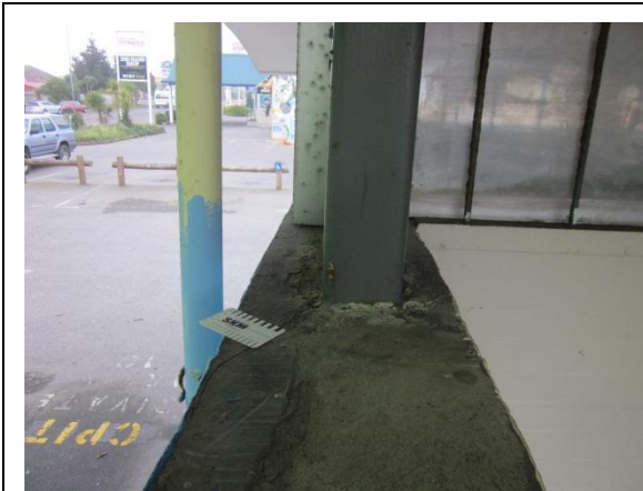
Photo 17: View of RHS column northwest corner (2)
