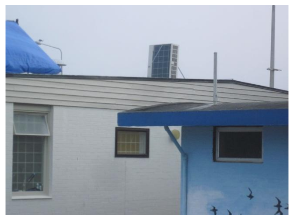
Photo 22: View of roof
