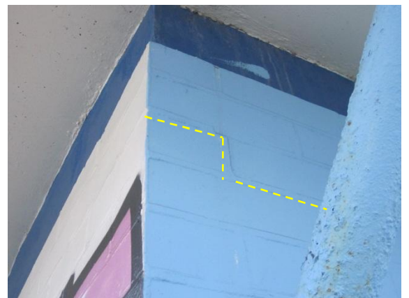
Photo 20: Close up view from photo 19 showing minor step cracks
