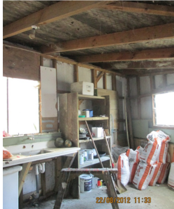
View of the opposite end of the northeast wall.
