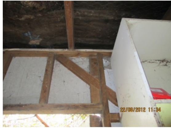
Timber bracing along the northeast end wall.
