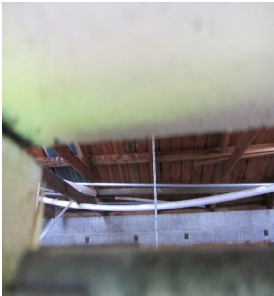
Photo 3: Internal view of shed
