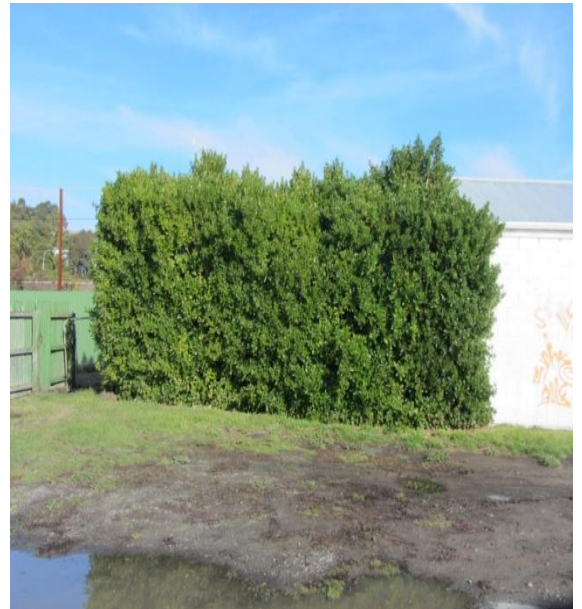
Photo 4: East Elevation (building is behind the hedges)
