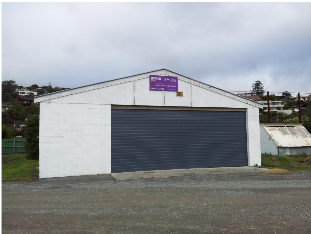
■ Figure 8 Overview of the double garage (PRK_1409_BLDG_008) referred to as "rescue boat shed" in the council files drawing
