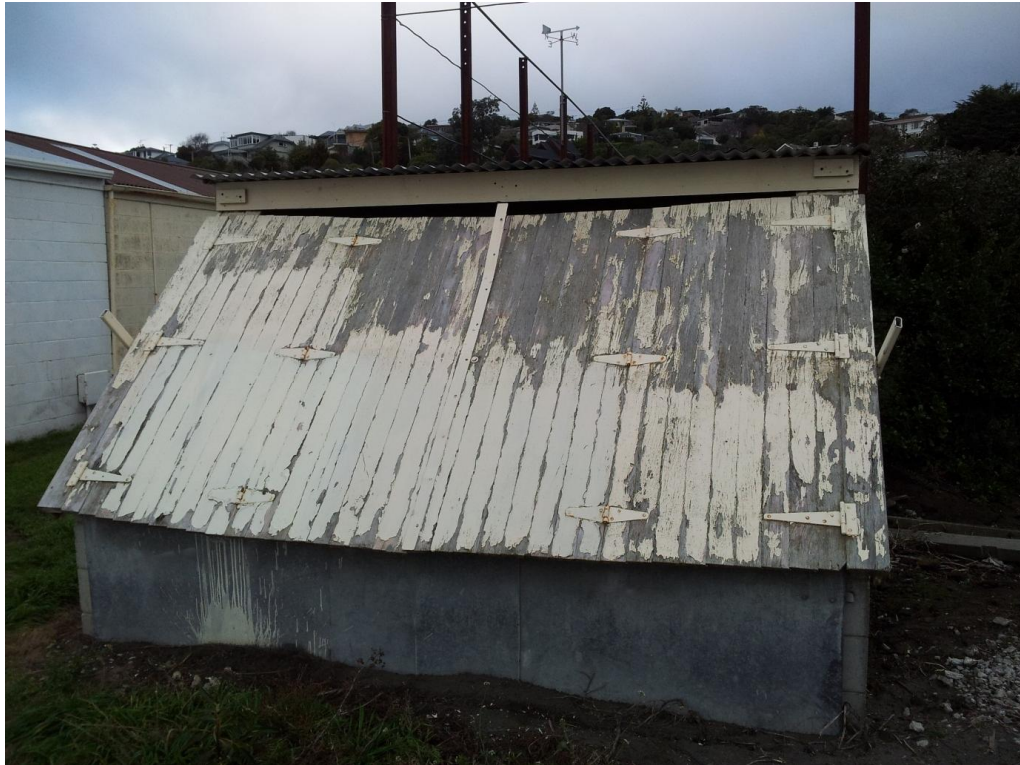
■ Figure 7 Overview of the storage shed (PRK_1409_BLDG_007)
