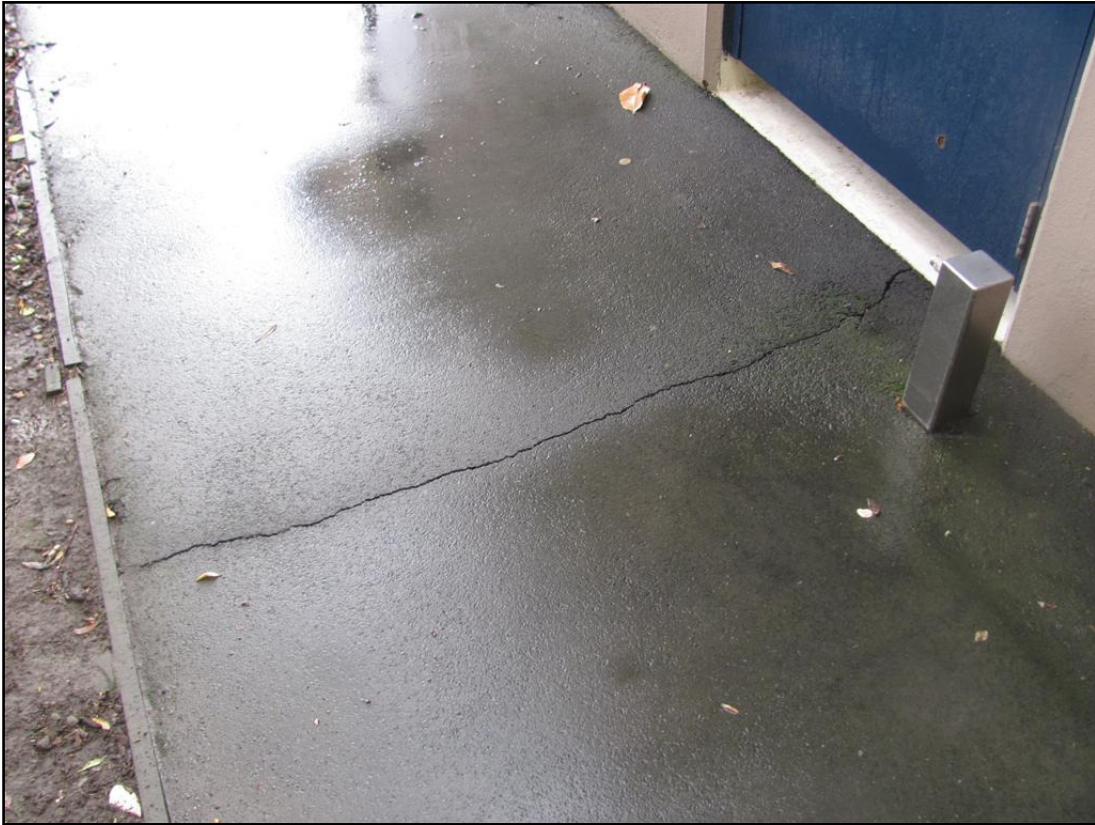
Photograph 11: View of the 5mm wide crack in the asphalt pavement located midway along the south facing side of the toilet block.
