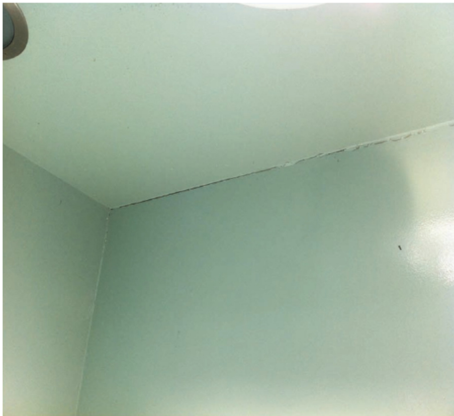
Cracking where the wall meets the ceiling in the southeast corner toilet
