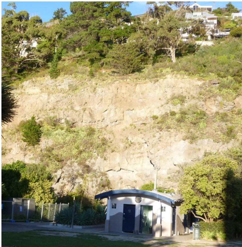
Rock face behind toilet facility
