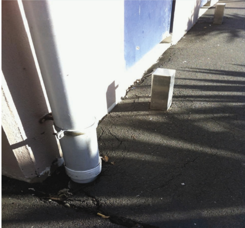
Separation between building foundation and footpath on the east side about 10-20mm
