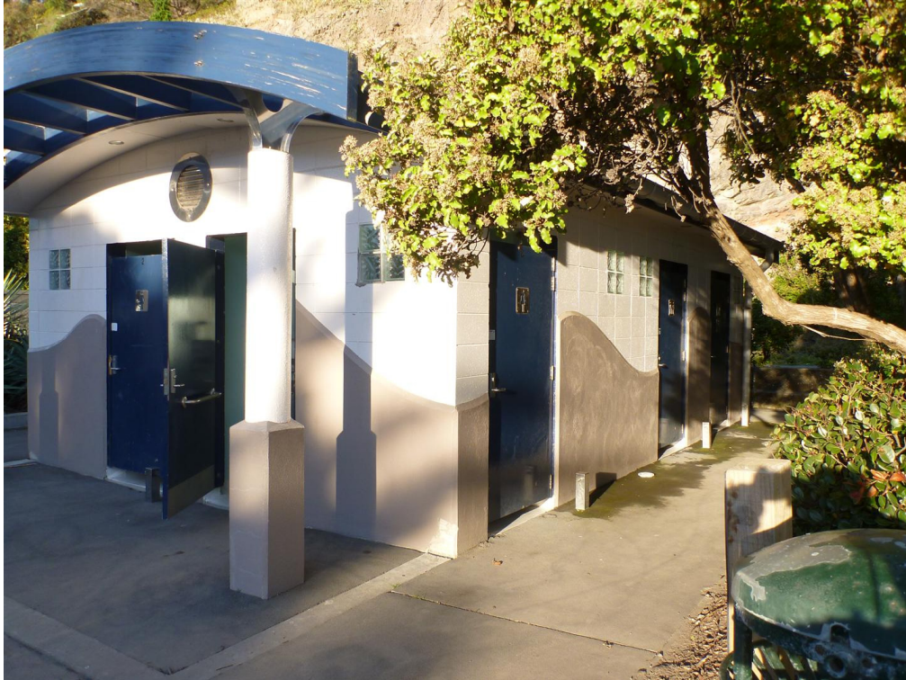
Front side (Note columns on separate foundation than building)
