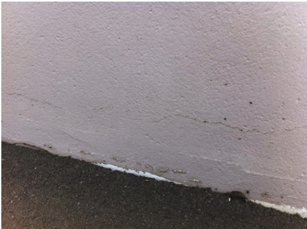
Hairline cracking at east side wall 1m long
