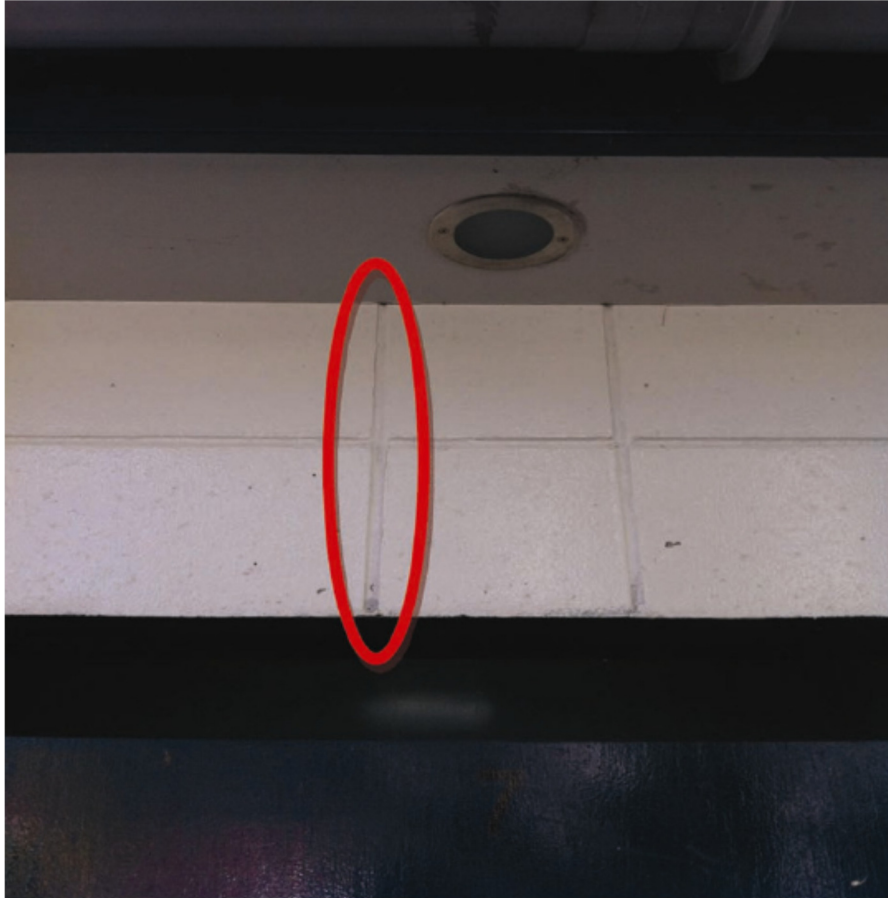
Cracking in mortar joint above door at midpoint on west wall
