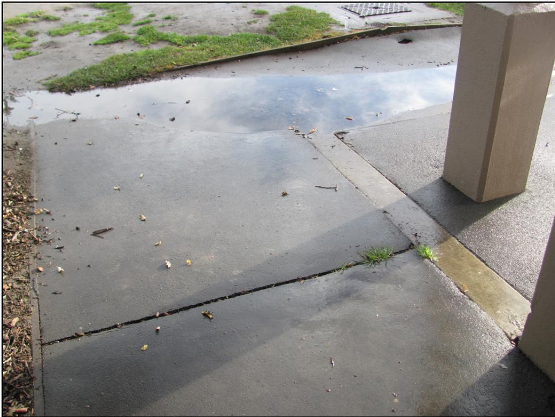
Photograph 8: View of 20mm wide crack in asphalt pavement located by the southwest corner of the toilet block.
