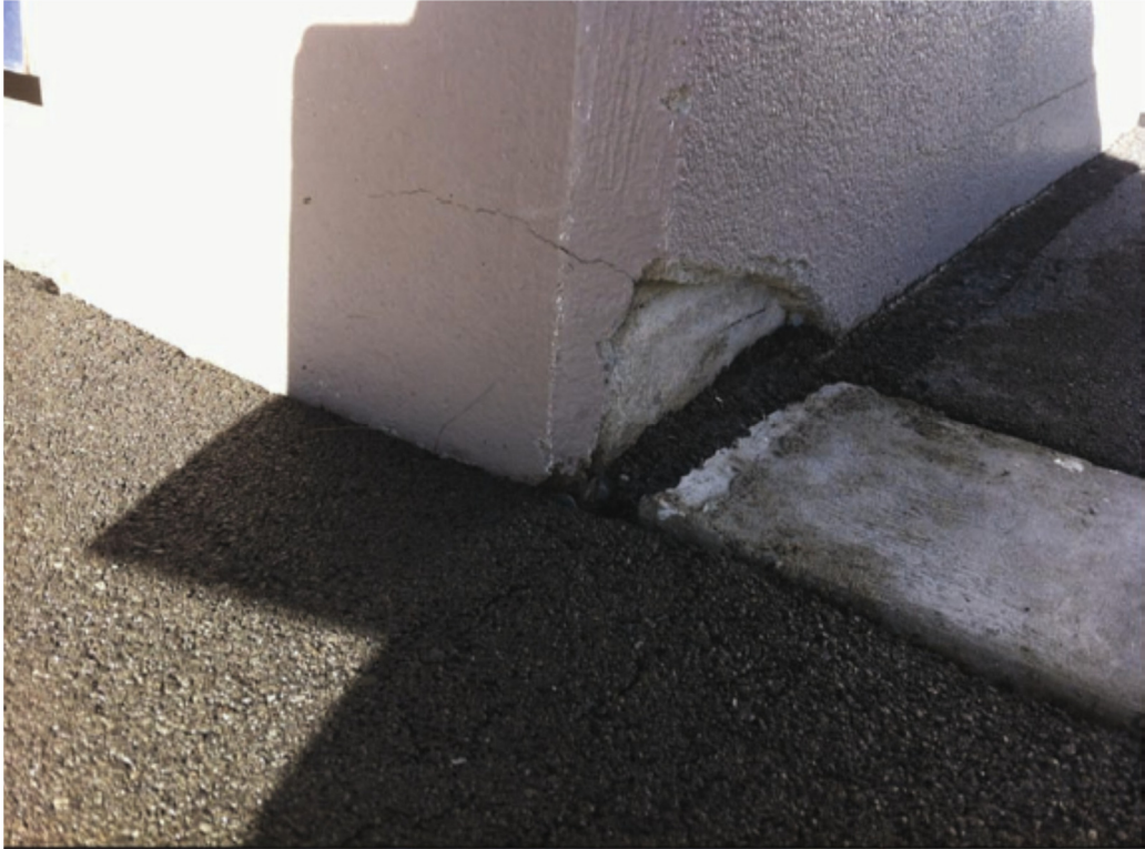
Hairline cracking and break away at the southeast corner
