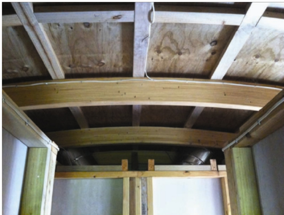
Roof structure in the service corridor
