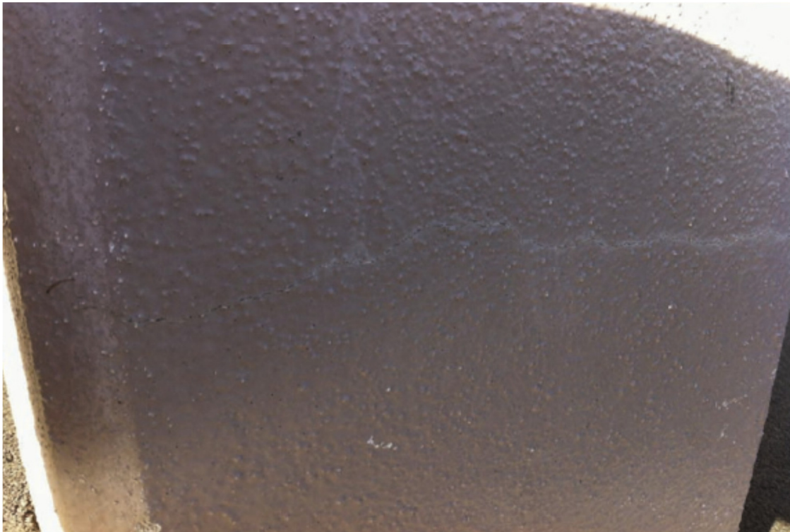
Hairline cracking on the southeast corner column
