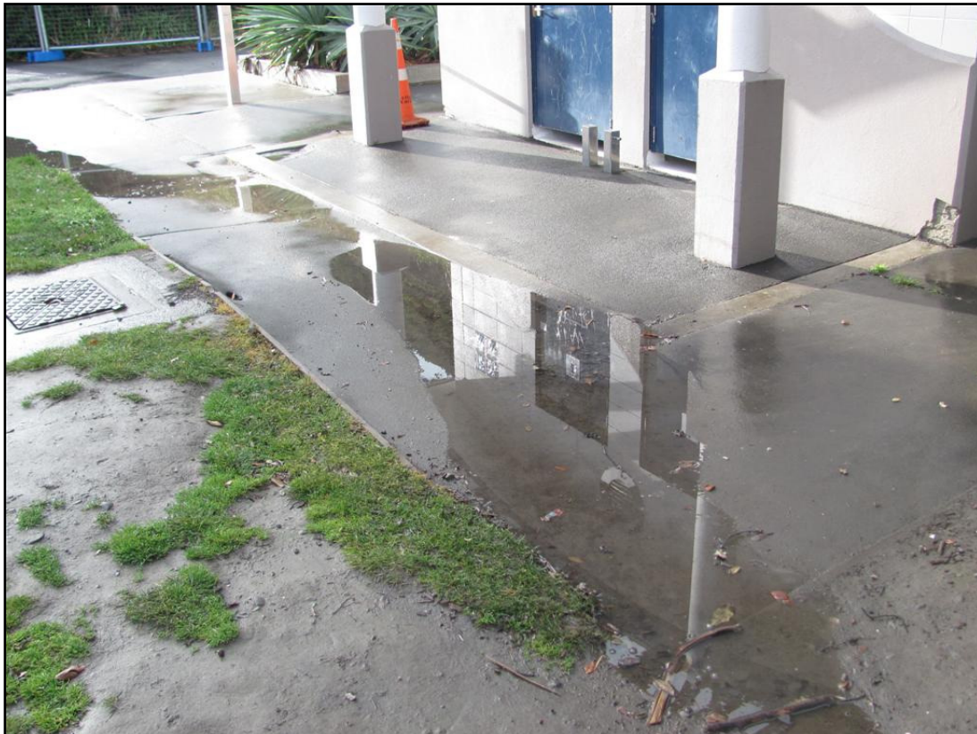
Photograph 4: View of the subsidence bowl in the asphalt pavement on the southwest corner of the toilet block.
