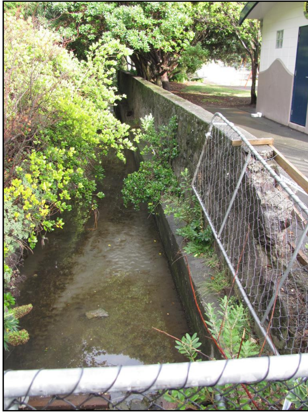
Photograph 7: View of the open drain located to the east of the toilet block.
