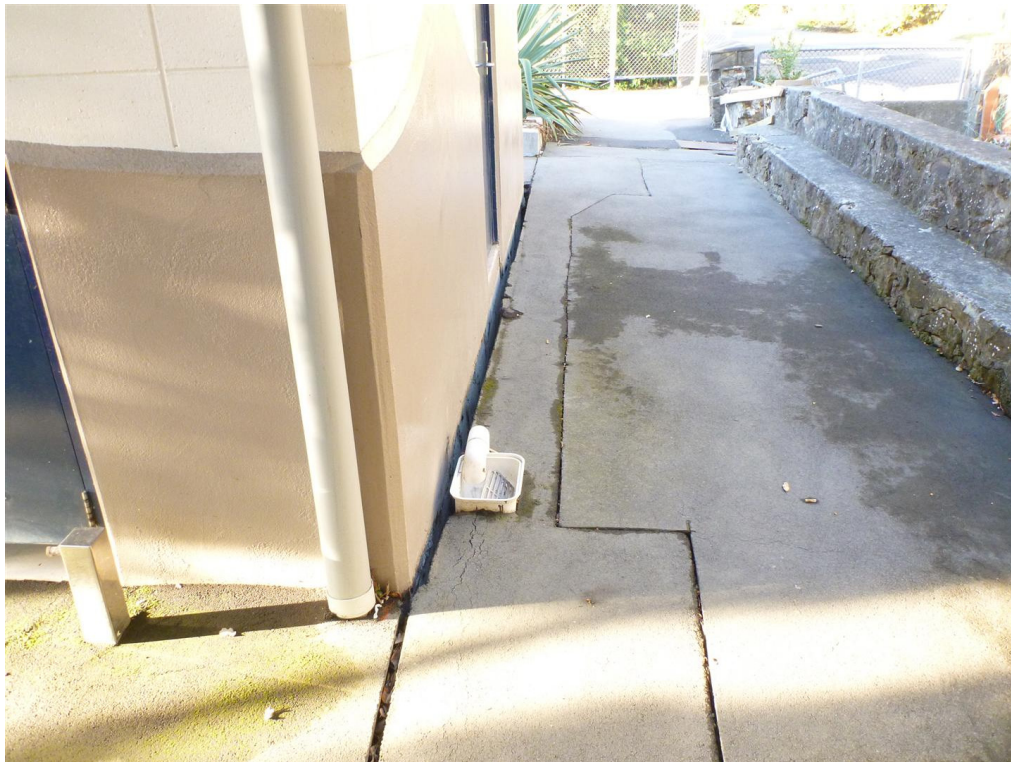
Rear (east) wall (Note the displacement of the building relative to surrounding slab)
