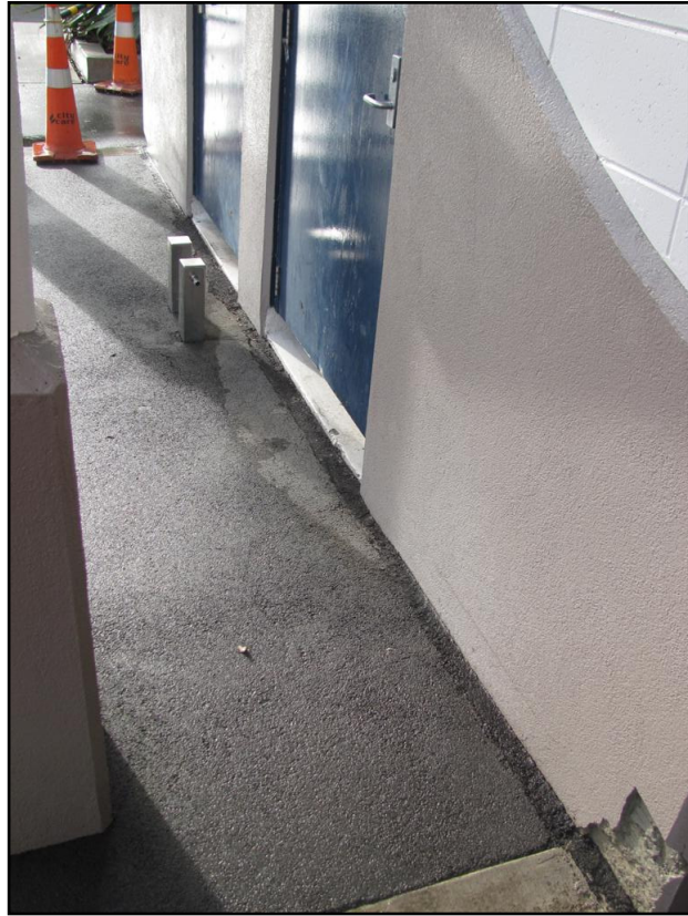
Photograph 5: View of horizontal separation of asphalt pavement from western edge of the toilet block footings (in-filled at time of site visit).
