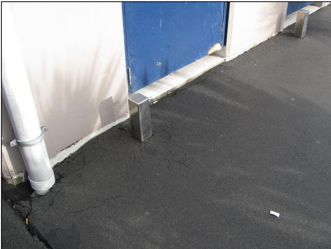
Photograph 12: View of between 20mm and 80mm of settlement of asphalt pavement along the northeast corner of the toilet block
