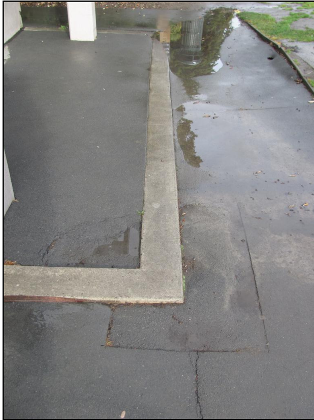
Photograph 9: View of View of 5mm wide crack in asphalt pavement located by the northwest corner of the toilet block.
