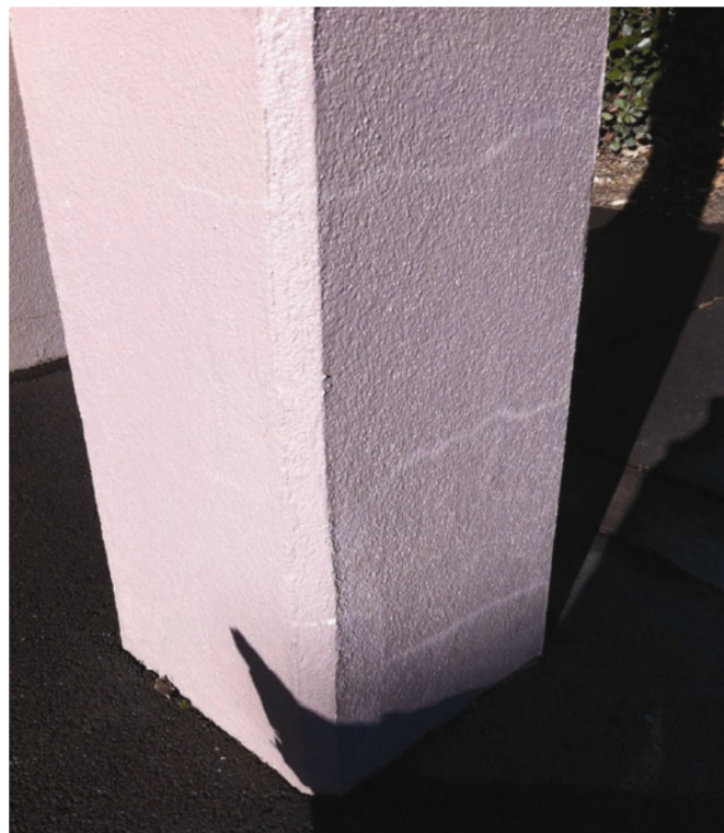
Hairline cracking on the southwest corner column
