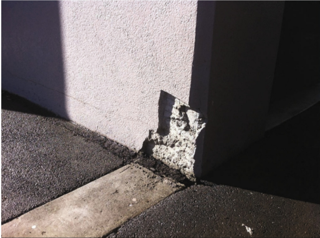
Hairline cracking and breakaway at the southwest corner
