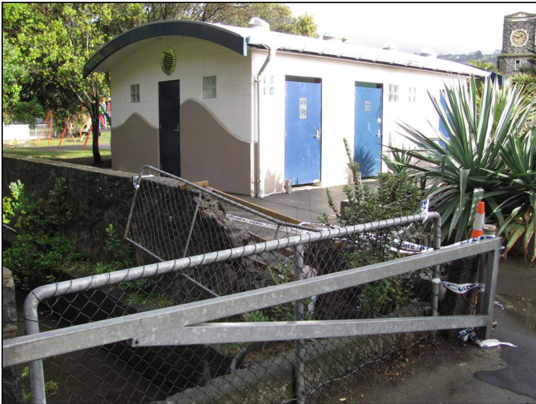
Photograph 2: View of east facing side of the toilet block
