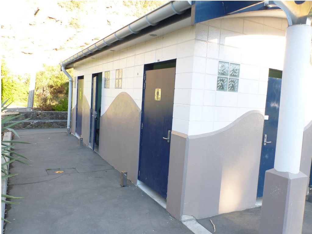
Right (north) wall (Note slab cracks. Note central CMU wall pier much stiffer)
