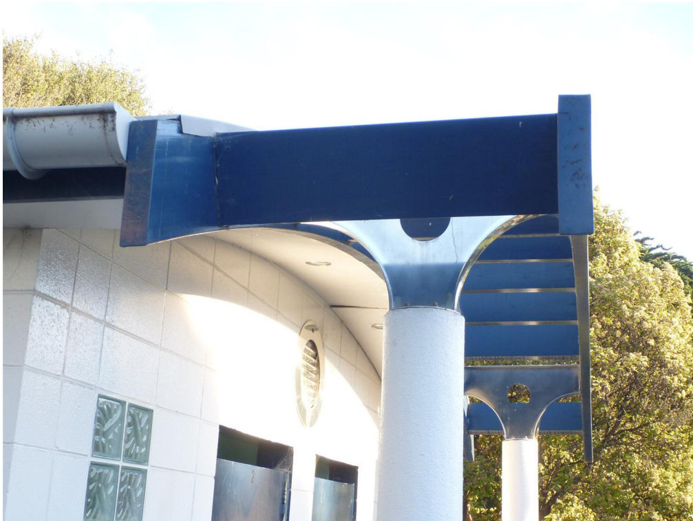
Front view showing column attachment and ceiling deformation
