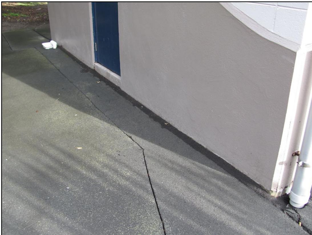
Photograph 6: View of horizontal separation of asphalt pavement from eastern edge of the toilet block footings (in-filled at time of site visit).
