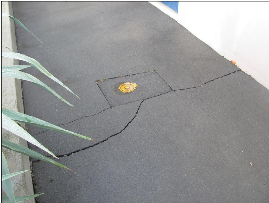
Photograph 10: View of the 10mm wide crack in the asphalt pavement located midway along the north facing side of the toilet block.
