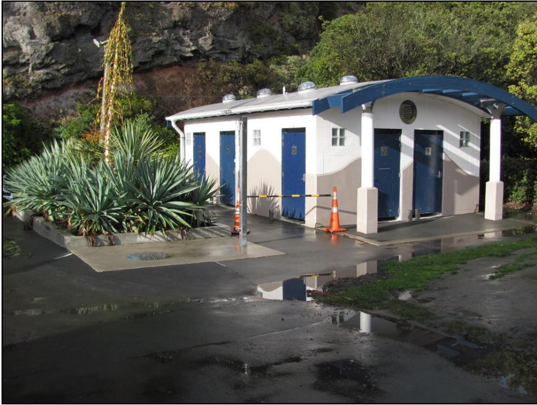
Photograph 1: View of North facing side of the toilet block
