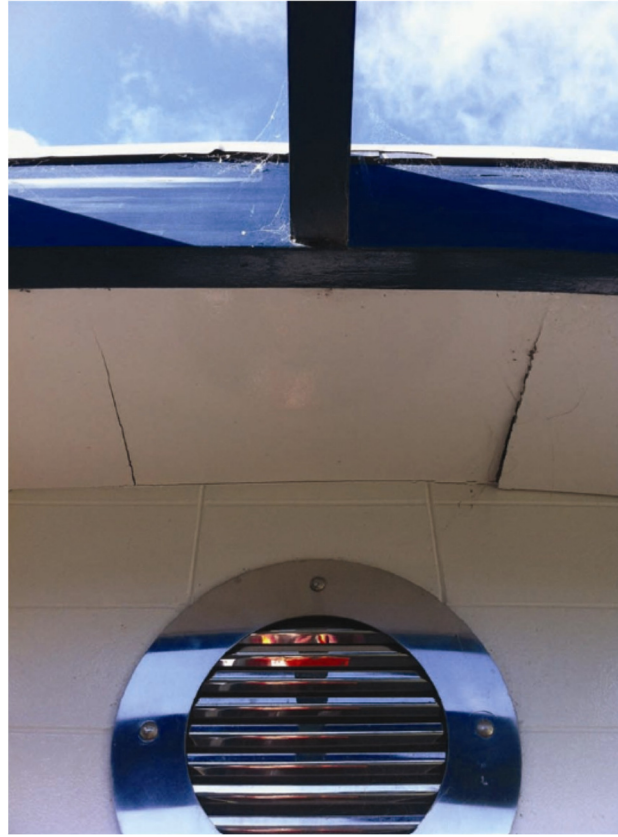
Movement in the eave on the south end
