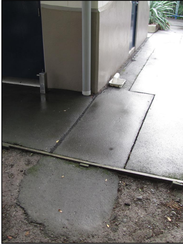
Photograph 13: View of the 20mm wide opening of asphalt pavement along eastern edge of the toilet block (possible trench to buried services).
