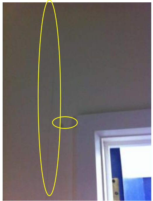
Photo 64: Vertical hairline Crack at wall Lining Joint Next to East Wall Door and Horizontal Crack Radiating out from Corner of Door in the First Aid Room
