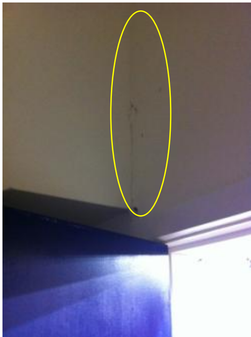
Photo 61: Close up of Photo 60
