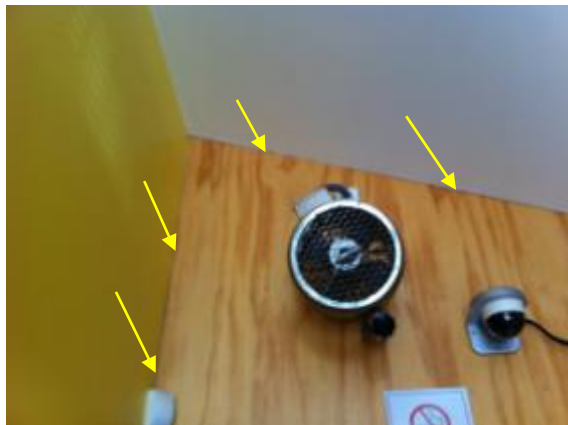
Photo 41: Hairline Cracking Between Ply and Plasterboard Lining Joints
