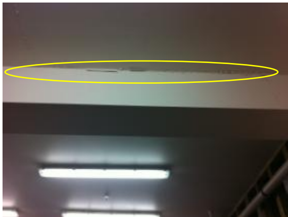
Photo 57: Close up of Photo 56
