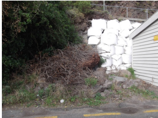
Photo 3 – Sand bags supporting dry stacked boulder wall that collapsed behind historic boat shed. Wall to right is still standing.
