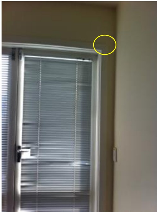
Photo 81: Mitre Joints on Window and Door architraves in the Kitchen have Opened up
