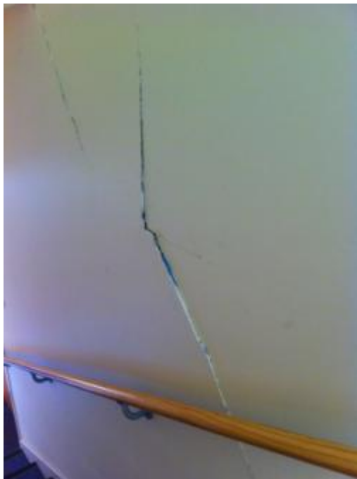
Photo 71: Close up of Cracking on SouthWall
