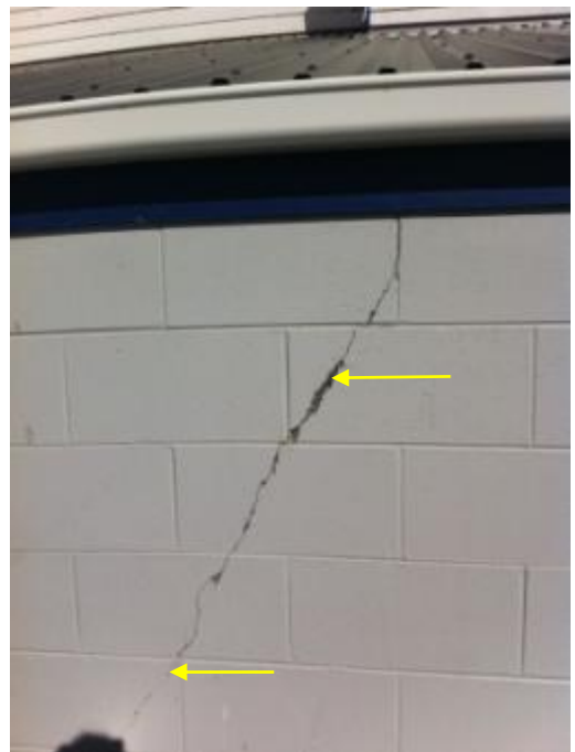
Photo 12: Diagonal Cracking to North Wall Blocks
