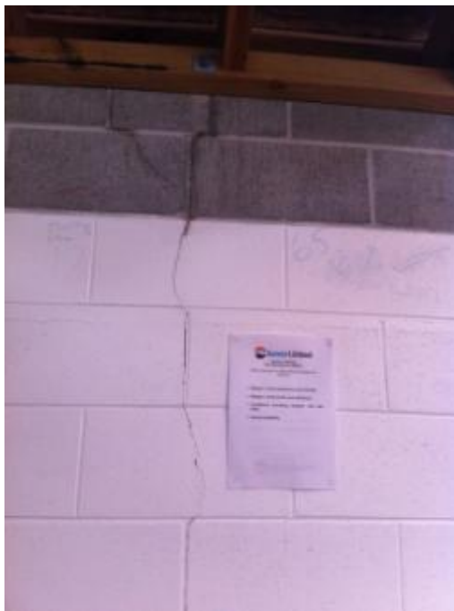
Photo 45: Internal Cracking of Northern Block Wall
