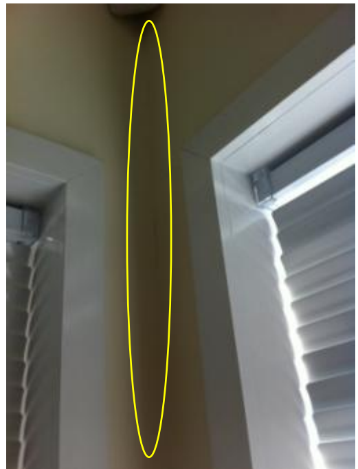
Photo 84: Hairline Cracking in SW Corner of Kitchen
