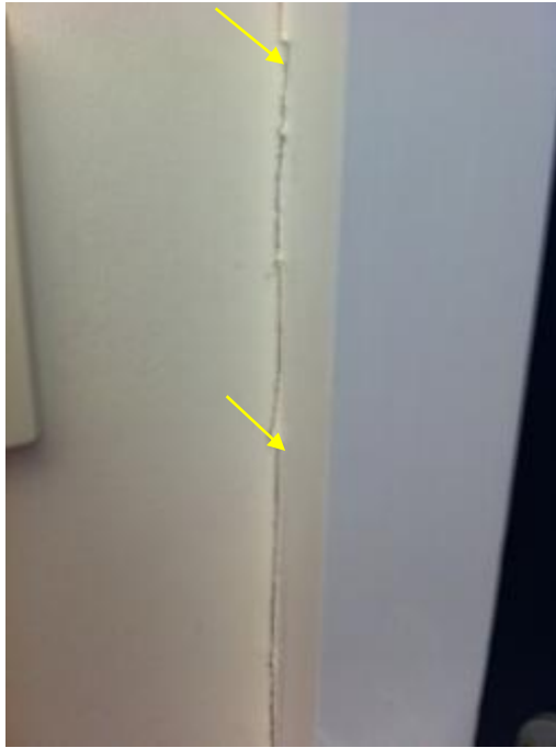
Photo 101: Close up of Photo 100
