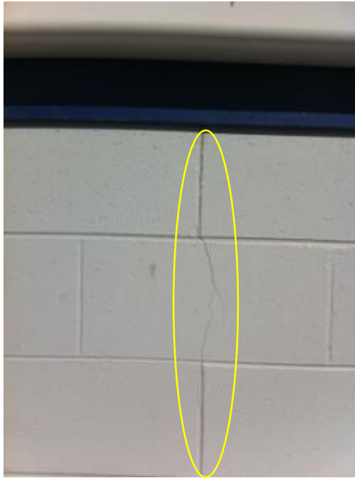
Photo 5: Vertical Cracking to North Wall Blocks
