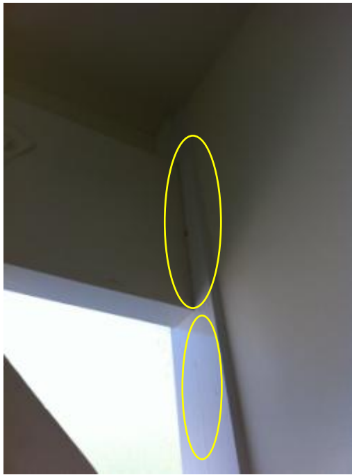
Photo 97: Cracking Present to Window Architrave in SE corner of South Stair
