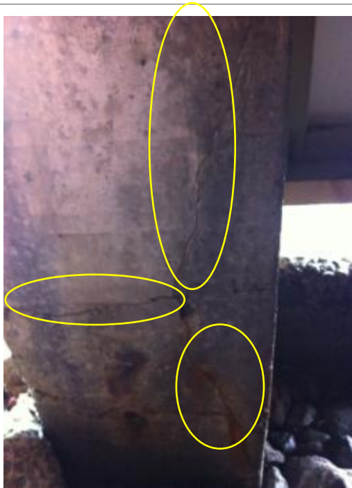
Photo 37: Cracking and Spalling to Concrete Pile
