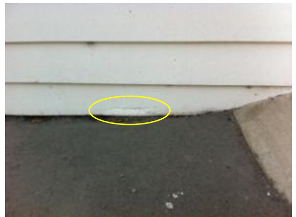
Photo 28: Cracking and Splitting of Weatherboard near SE Corner
