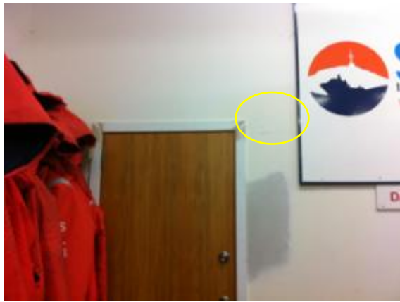
Photo 51: Cracking in Wall Lining above Door near NE Corner of Main Boat Shed
