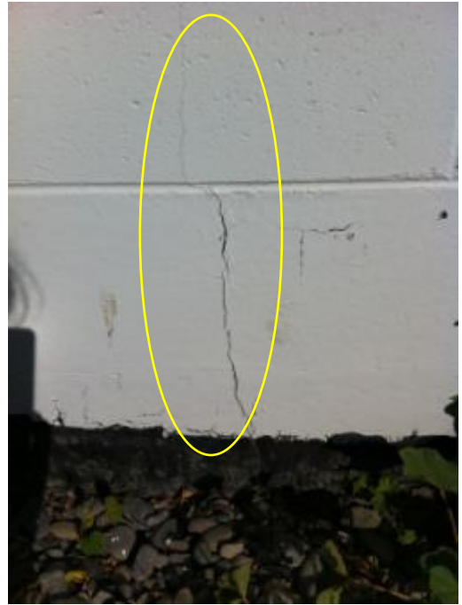
Photo 6: Cracking Continuing through Concrete Foundation
