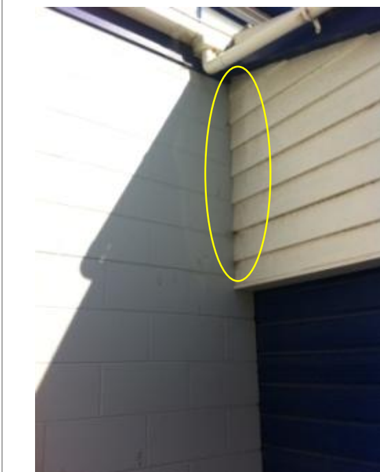
Photo 23: Hairline Cracking Between Timber Cladding and Block Wall Joint
