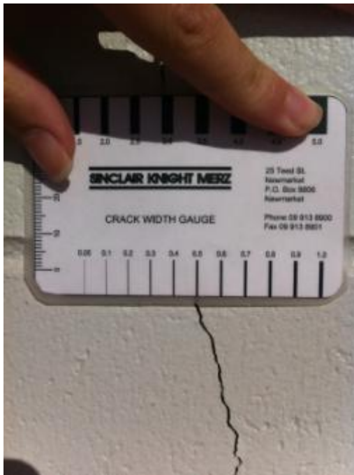
Photo 7: Close up of North Wall Crack
