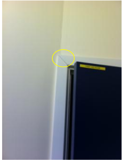
Photo 102: Mitre Joints in First aid Room Door architrave have Opened up
