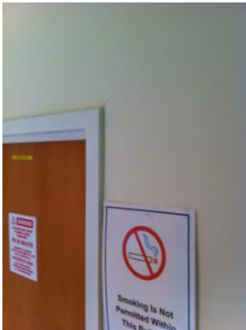
Photo 67: Cracking Between Wall Lining and Main Boat Shed Door Architraves
