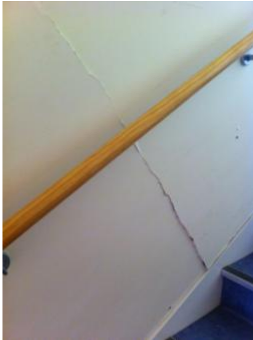
Photo 69: Severe Cracking to Wall Lining on the SouthWall (Bottom of Cracking)
