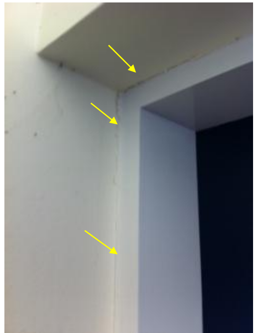
Photo 100: Cracking around East Exit Door
