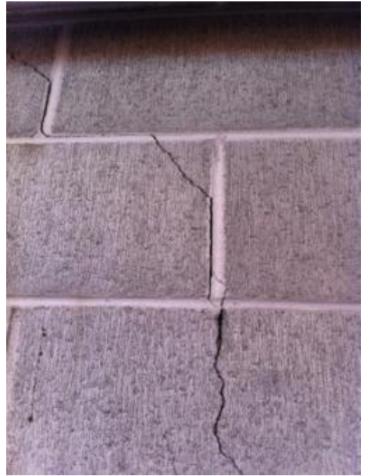
Photo 44: Internal Cracking of Northern Block Wall
