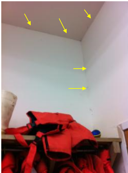
Photo 53: Hairline Cracking at Lining Joints in the NE Corner of Main Boat Shed
