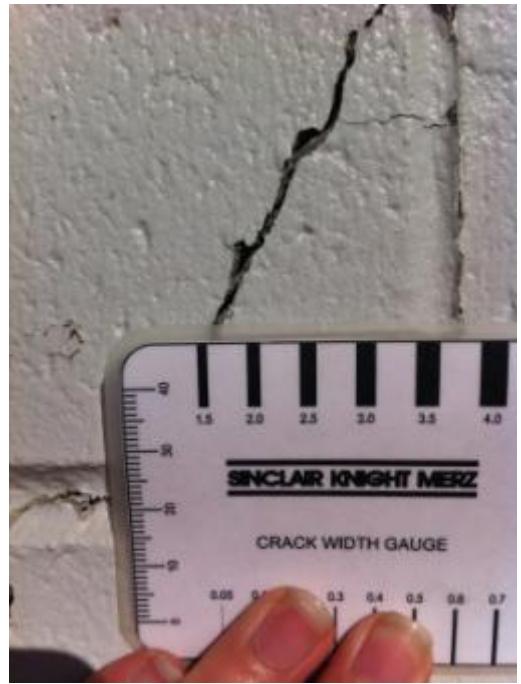
Photo 14: Close up Of Diagonal Cracking
