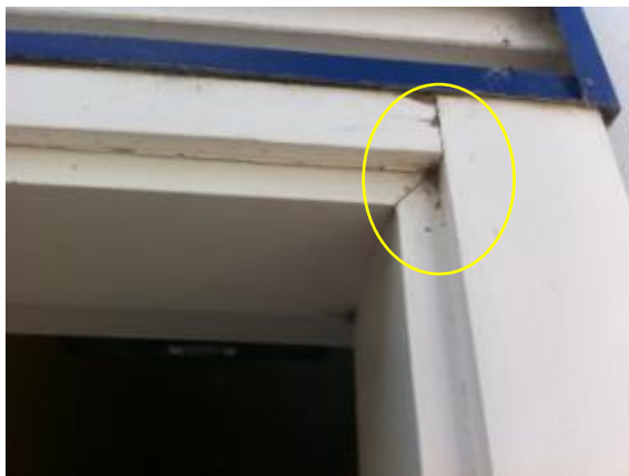
Photo 27: Timber Door Frame and Architrave Joints have Opened up
