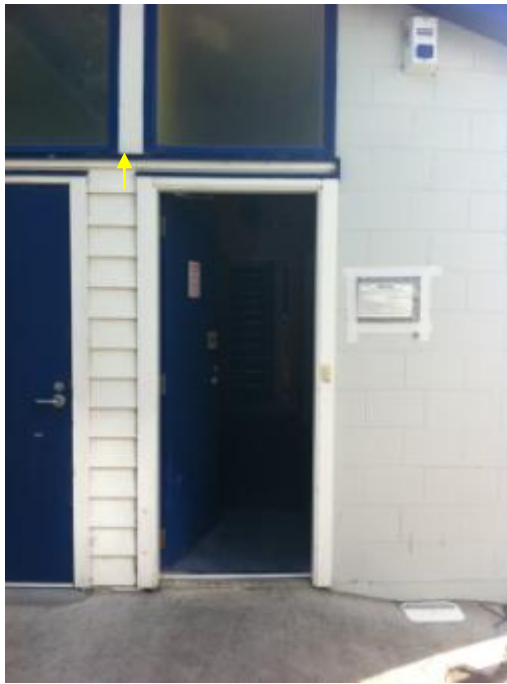
Photo 25: Opening up of Joints in Weatherboards
