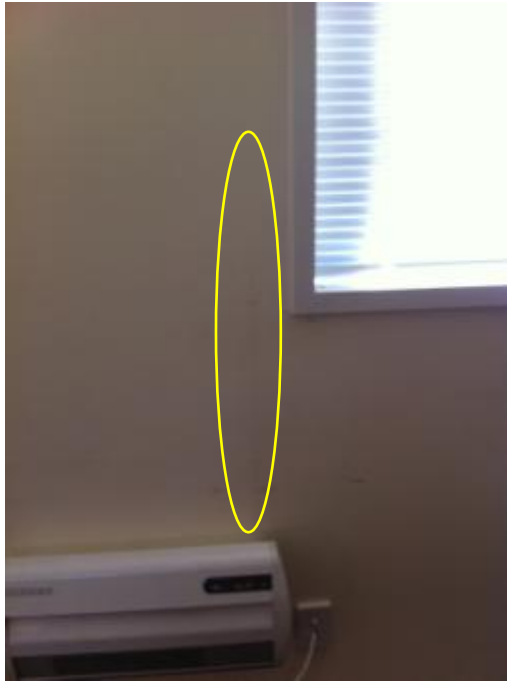
Photo 89: Vertical Hairline Crack on North Wall of L1 Main Room
