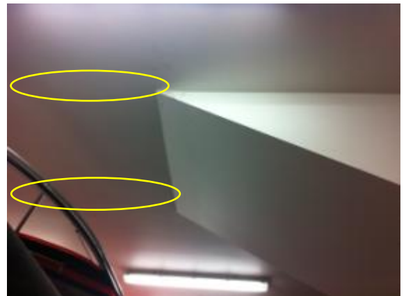
Photo 58: Hairline Cracking at Ceiling Lining Joints
