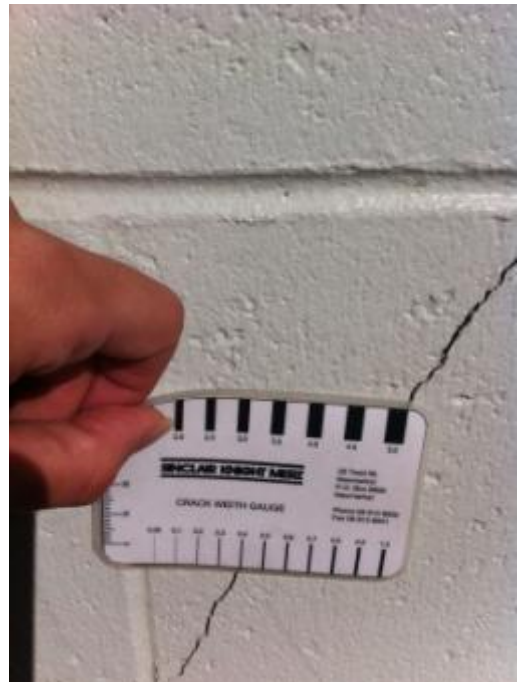
Photo 16: Close up of Photo 17
