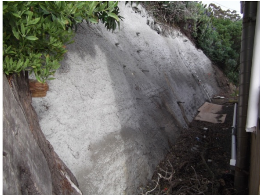
Photo 1 – Shotcrete wall behind jet boat shed.
