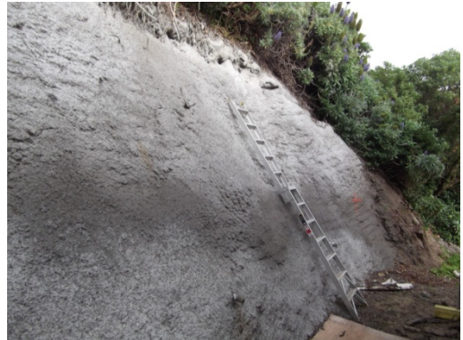
Photo 2 – Shotcrete wall behind jet boat shed
