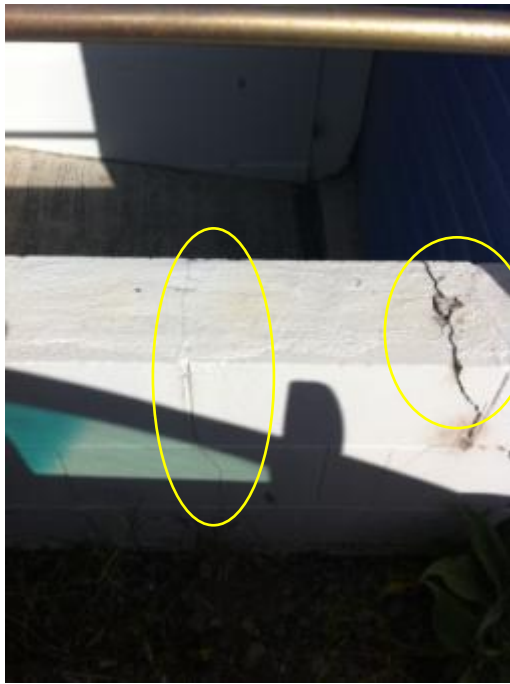
Photo 17: Cracking to Block Wall Balustrade
