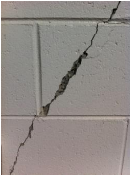
Photo 13: Close up Of Diagonal Cracking
