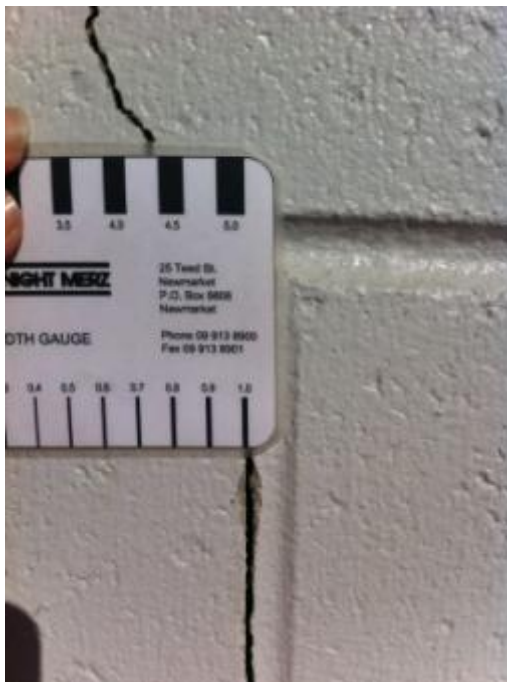
Photo 11: Close up of North Wall Cracking
