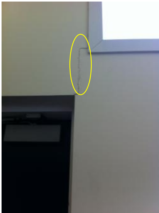
Photo 99: Cracking above East Exit Door in West Stair
