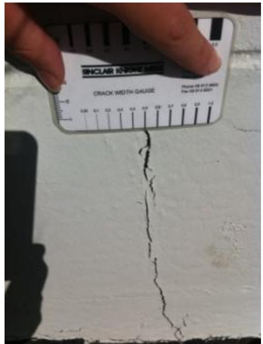
Photo 8: Close up of Foundation Crack
