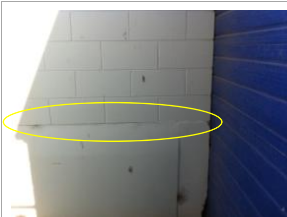
Photo 21: Hairline Cracking Along Block Wall and Concrete wall Joint
