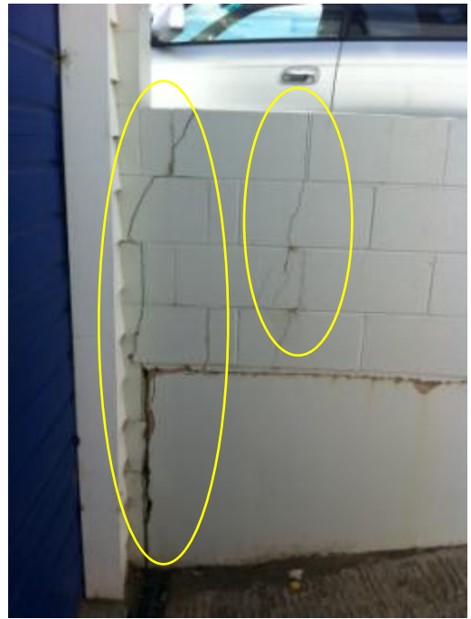
Photo 18: Cracking to Block Wall Balustrade
