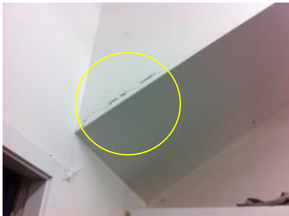
Photo 49: Cracking to Stair Wall Lining Joints near East Wall in Main Boat Shed
