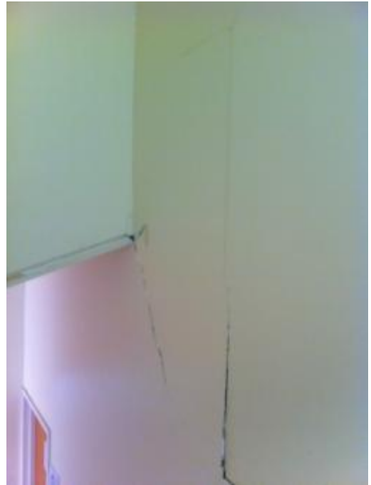
Photo 70: Severe Cracking to Wall Lining on the South Wall (Top of Cracking)
