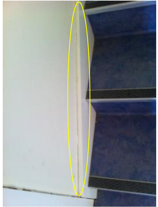
Photo 66: Cracking Between Timber Stair Skirting and Wall Lining Joint in Eastern Stairwell
