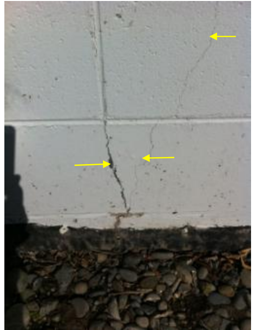
Photo 10: Cracking to Concrete Foundation
