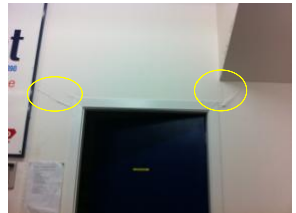
Photo 50: Diagonal Cracking to Wall Lining above First Aid Room Door
