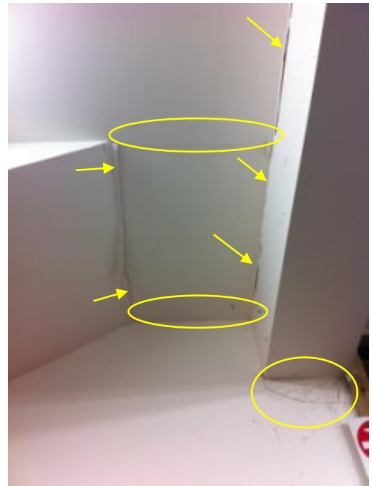
Photo 48: Close up of Cracking to Linings on Southern Wall of Main Boat Shed
