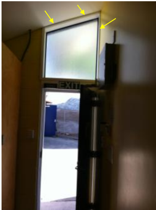
Photo 39: Cracking present Between South Wall Window architrave and Linings
