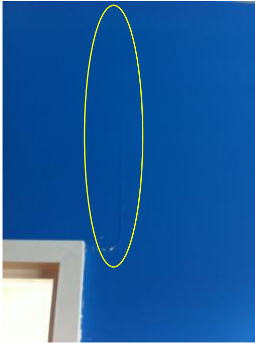
Photo 77: Vertical Hairline Crack at Wall Lining Joint above Door in the Communications Room
