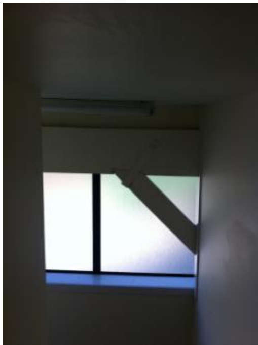
Photo 95: Cracking around Timber Brace in South Stair
