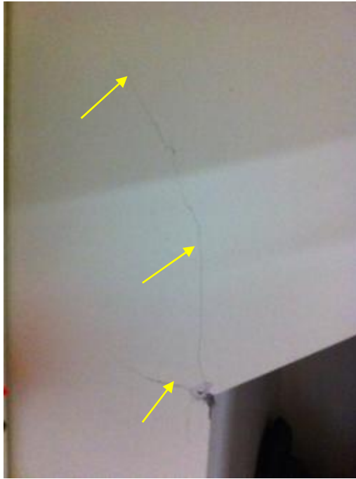
Photo 63: Diagonal Cracking at Stair Re-Entrant Corner in First aid Room
