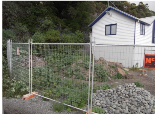
Photo 4 – Rubble removed from behind historic boat shed.
