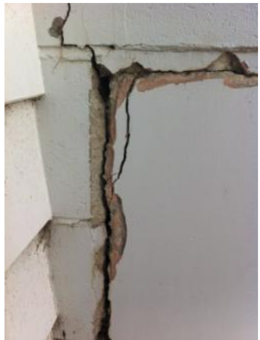
Photo 20: Cracking between Concrete Retaining Wall & Masonry Wall Joint
