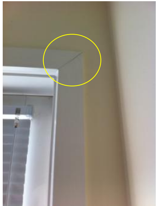
Photo 82: Close up of Photo 81
