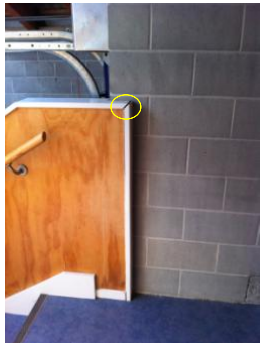
Photo 46: Mitre Joints in Wooden Balustrade Trim have Opened up
