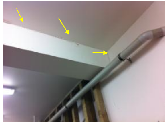
Photo 56: Cracking Between Floor Beam Lining and the Ceiling and Wall Lining Joints – North Wall of Main Boat Shed
