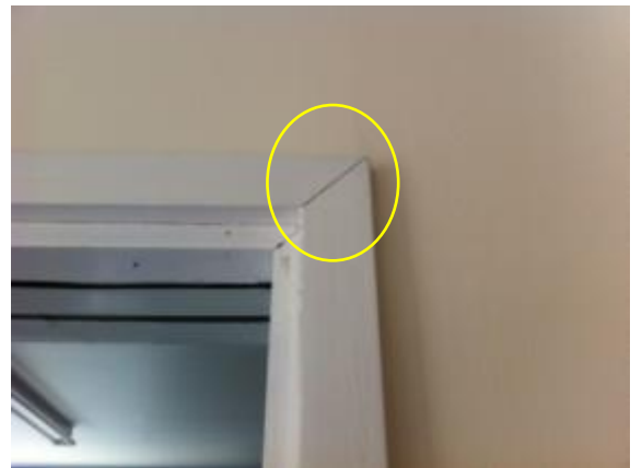
Photo 80: Close up of Photo 79
