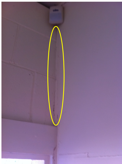
Photo 15: Hairline Cracking between Block and Timber Wall Joint in SW Corner of East Stair
