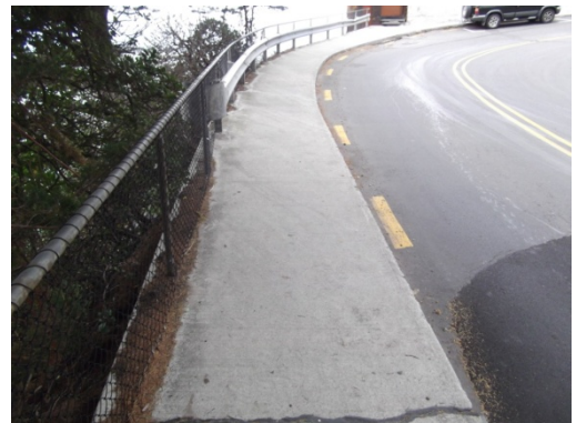
Photo 6 – Section of road which has moved approximately 15mm (looking north).
