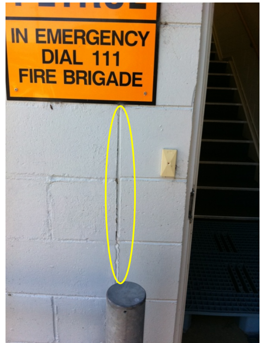
Photo 6: Minor Cracking to Block Wall Mortar Joints Near SE Corner
