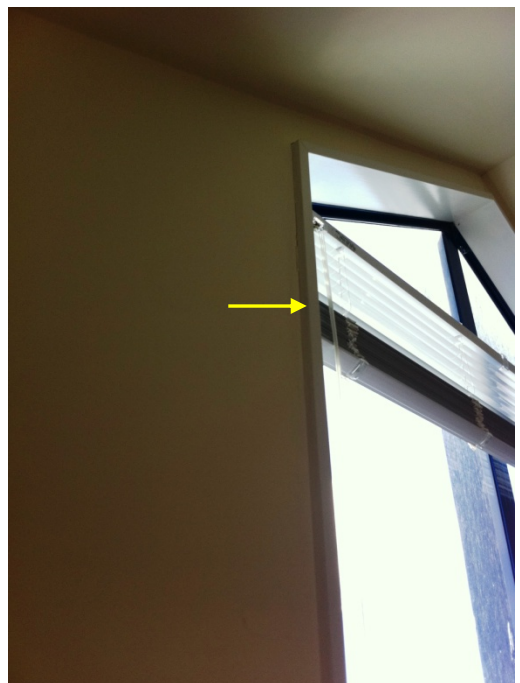
Photo 32: Hairline Cracking Between the Window Architrave and the Wall Lining Joint
