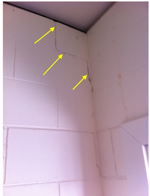
Photo 12: Minor Cracking to Block Wall Mortar Joints in SE Corner
