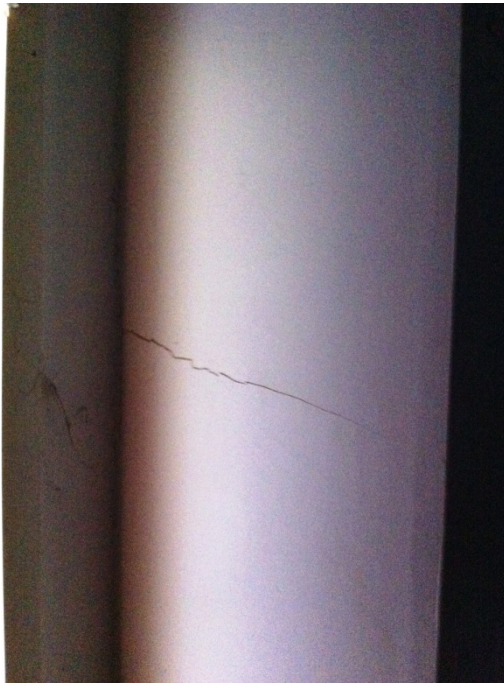
Photo 29: Cracking to Wall Lining in the SE Corner of the Garage
