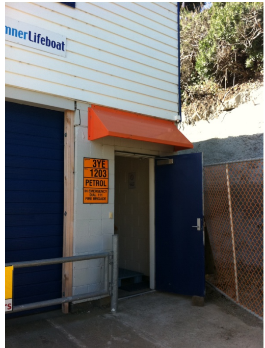
Photo 4: Cracking to Block Work Near Roller Door
