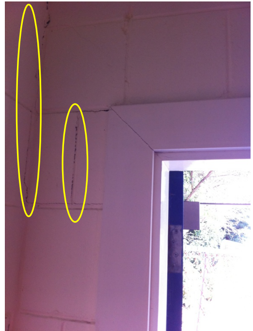
Photo 14: Minor Cracking to Block Wall Mortar Joints in SE Corner of East Stair
