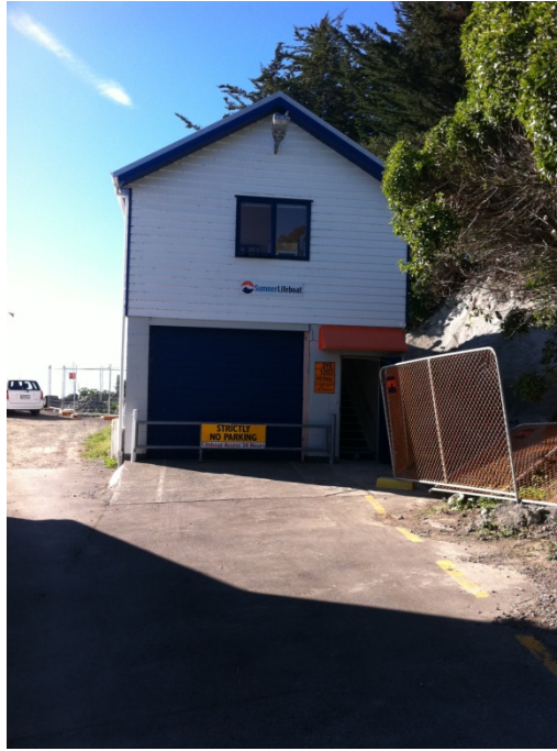
Photo 1: South Elevation. No bracing wall at ground floor level
