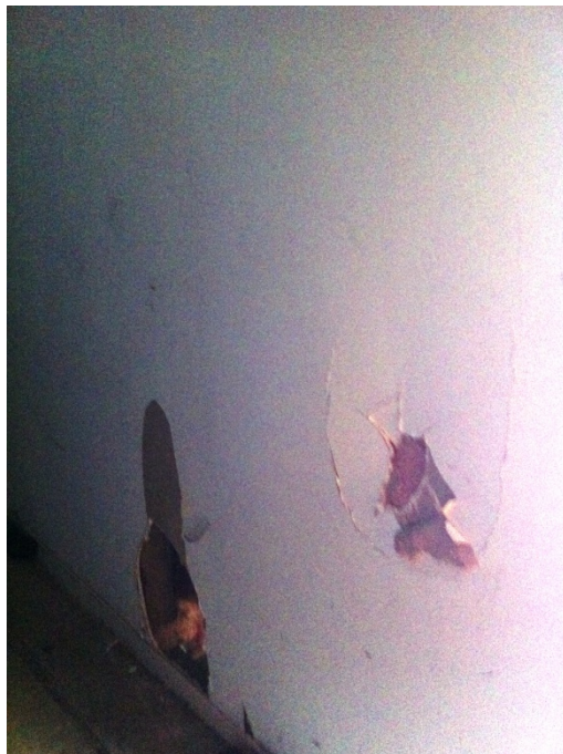
Photo 27: Damage to East Wall of Garage – Not EQ Damage
