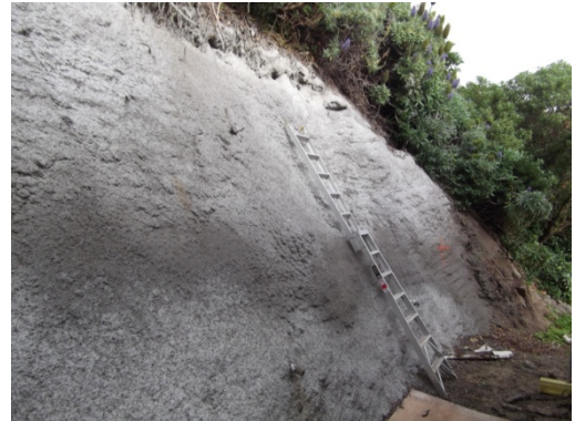
Photo 2 – Shotcrete wall behind jet boat shed
