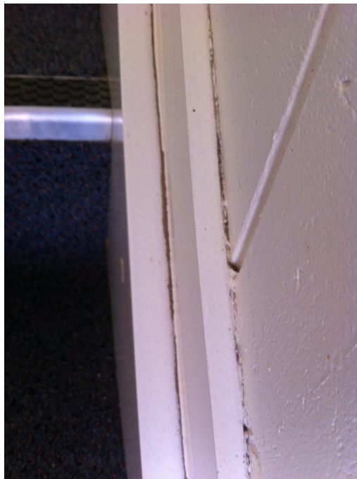
Photo 19: Cracking along Timber Stair Skirting Joints
