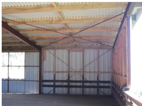
Photo 9: Steel cross-bracing in the walls and
