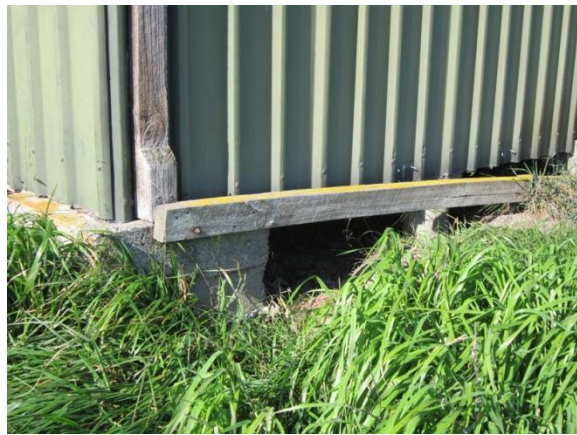
Photo 5: Concrete footing and timber pile on northwest corner of three-walled structure
