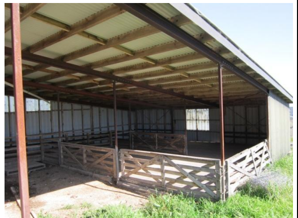
Photo 8: Steel beams and posts spanning longitudinally in three-walled structure
