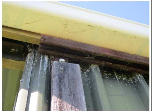
Photo 6: Rusted steel element (typical)
