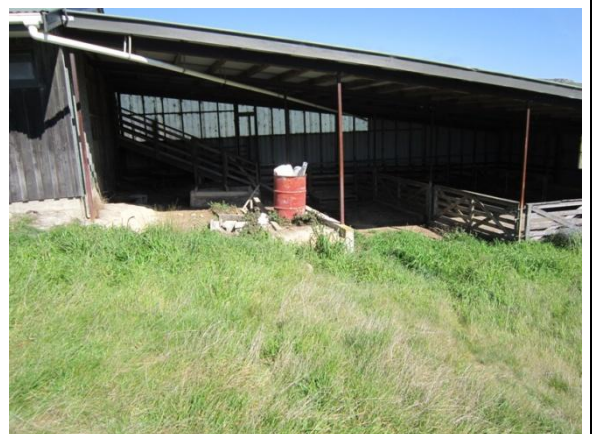
Photo 10: Sloping ground causing height
