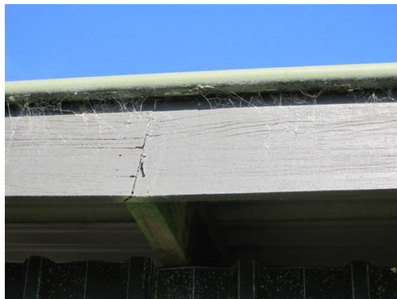
Photo 7: Splitting of timber element along the grain (typical)
