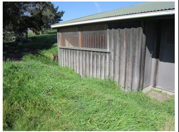
Photo 16: Trench created around eastern end of enclosed structure
