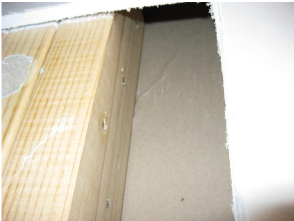
Photograph 14 Close up of opening up work to cracking above internal doorway.
