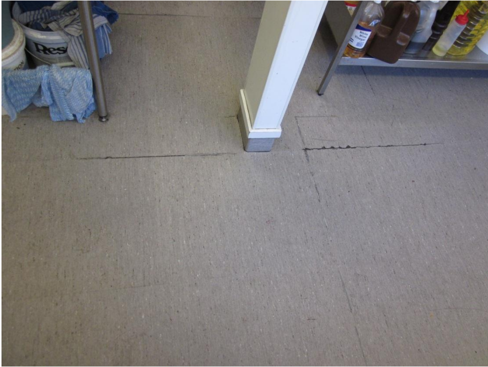
Photograph 11 Minor residual displacement of floor shown by displaced carpet floor tiles.
