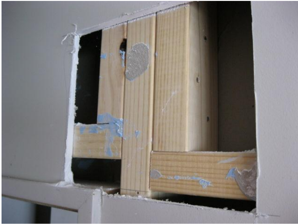
Photograph 13 Opening up works to determine extent of damage to timber structure.
