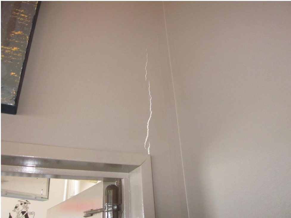
Photograph 6 Cracking to plasterboard lining above internal doorway.
