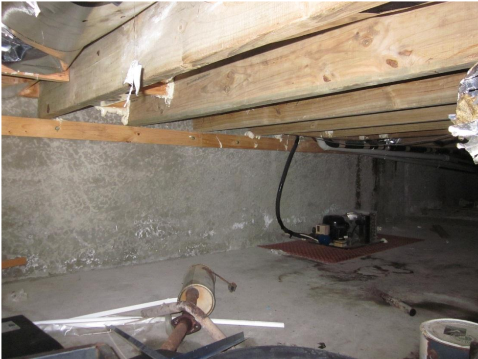
Photograph 12 Substructure and foundations of extension to southern side of original building.
