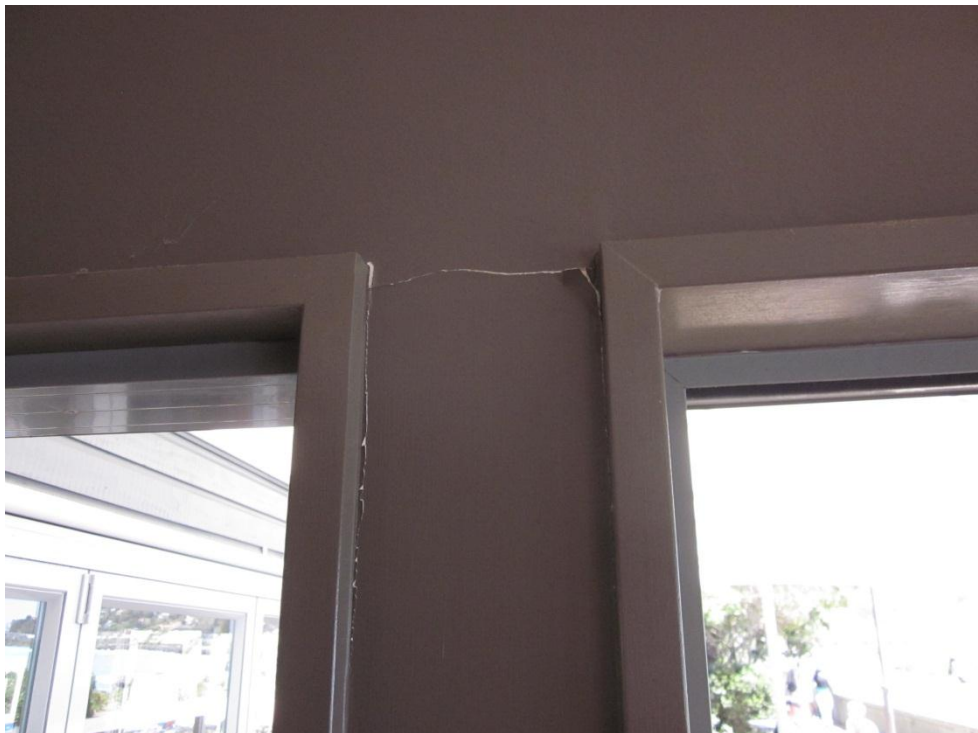
Photograph 10 Cracking to plasterboard lining between external door and window.
