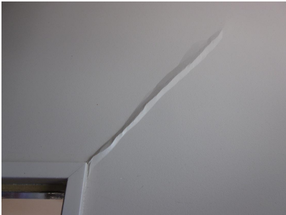
Photograph 8 Further cracking to plasterboard lining above internal doorway.
