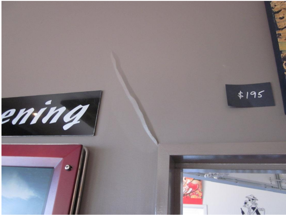
Photograph 7 Diagonal cracking to plasterboard lining above internal doorway.
