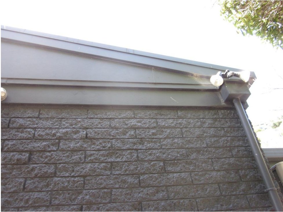
Photograph 5 Brick veneer cladding.
