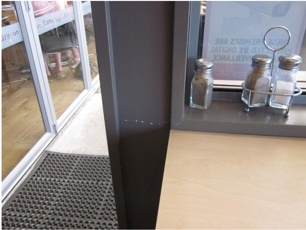
Photograph 9 Cracking to plasterboard lining between external door and window.
