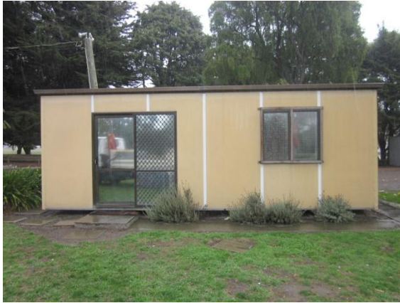
Photo 1: Front Elevation of Building
