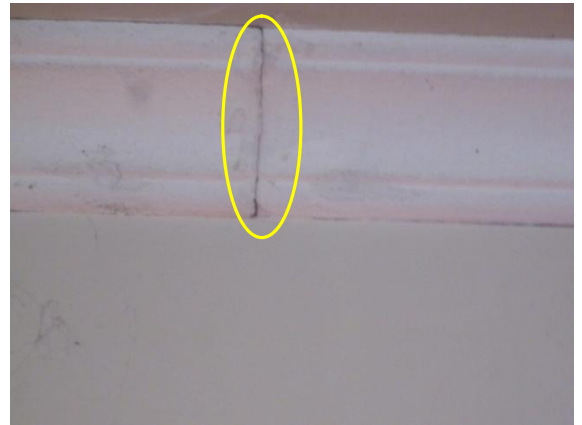
Photo 4: Hairline Cracking at Scotia Joints
