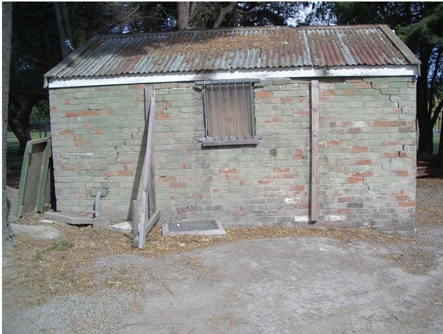
■ Figure 8 Visible damage to the tool shed
