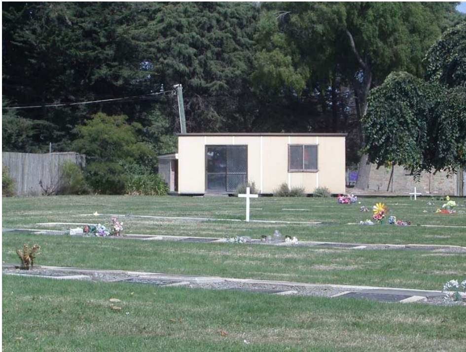
■ Figure 9 No visible damage to land or the building
