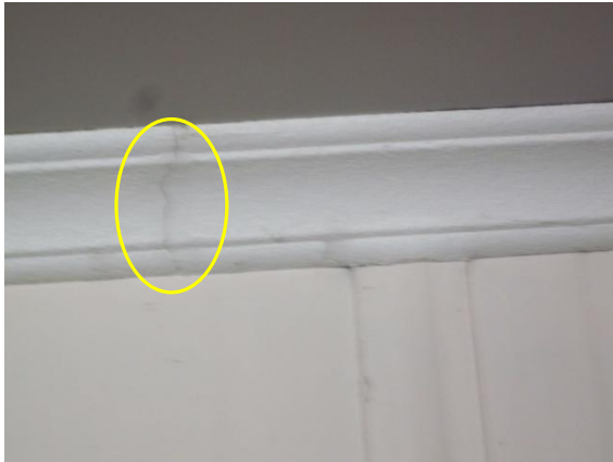
Photo 5: Hairline Cracking to Scotia
