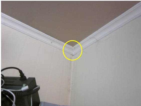
Photo 3: Hairline Cracking at Scotia Joints
