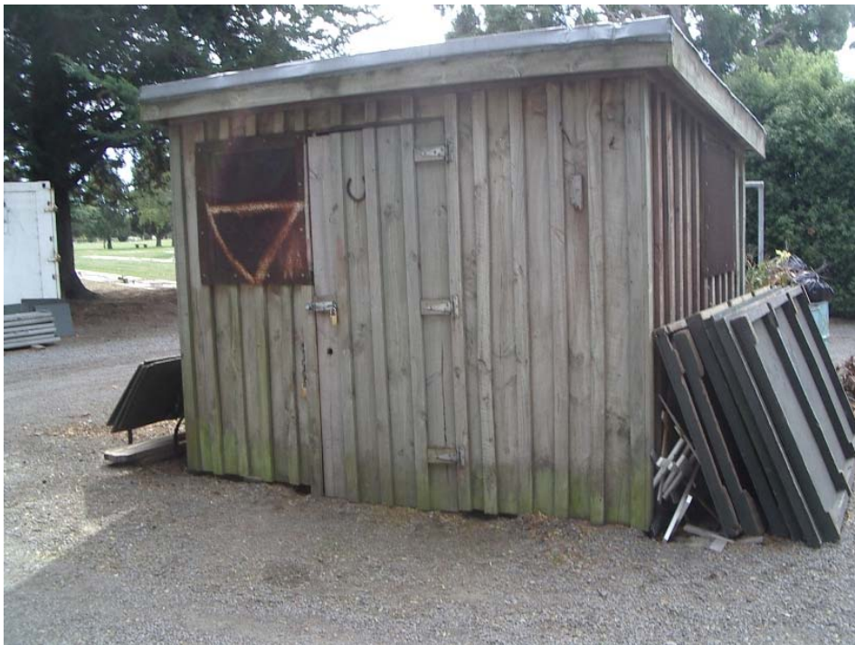
■ Figure 10 No visible damage to the pump house
