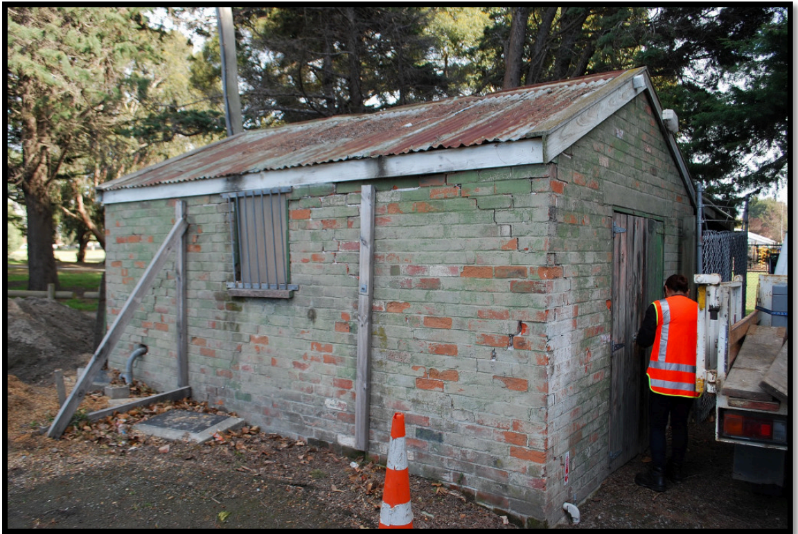
Photograph 10 Temporary prop strengthening on outside of the building.
