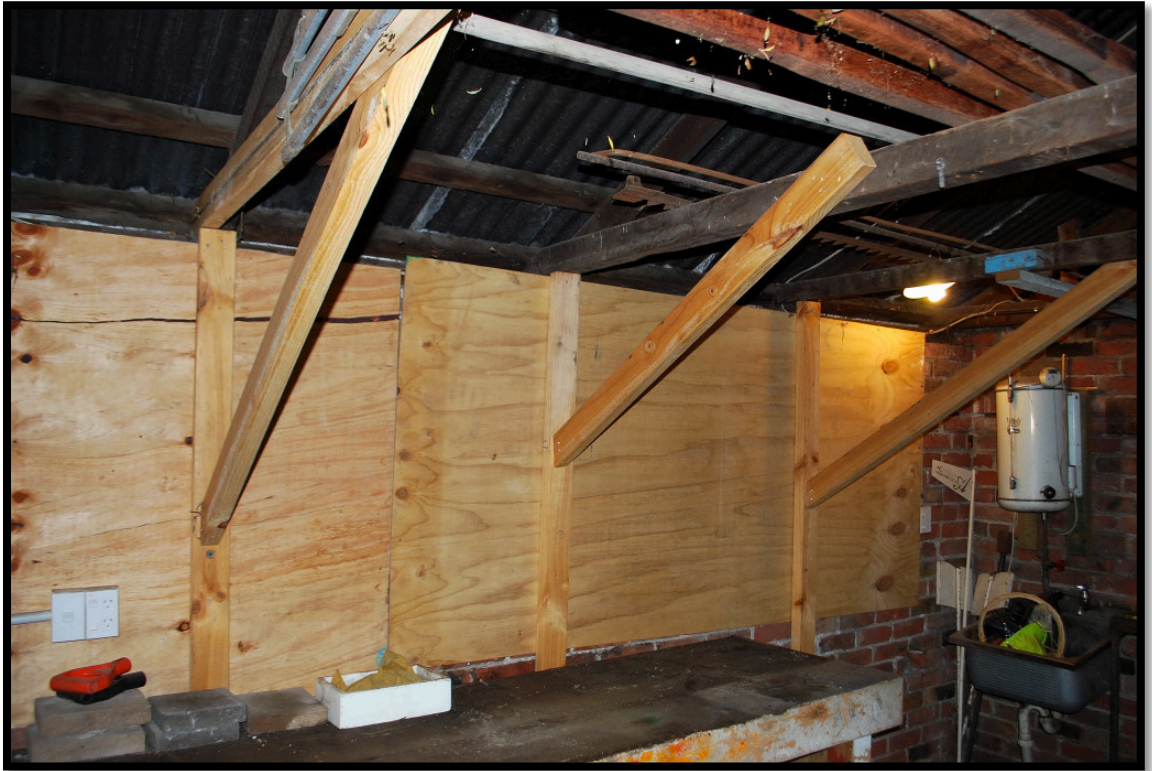
Photograph 9 Temporary prop strengthening on the inside of the building with Ply and 4x2 timber.
