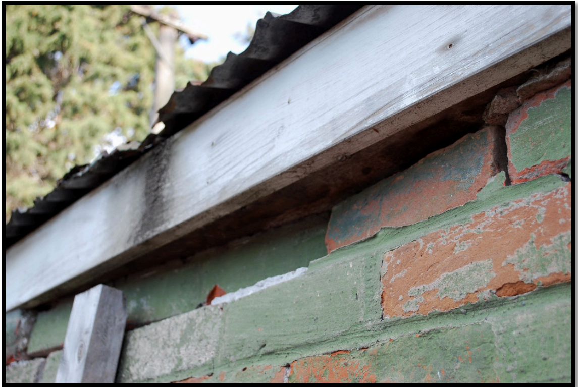
Photograph 7 Northeast walls top row of bricks separating.
