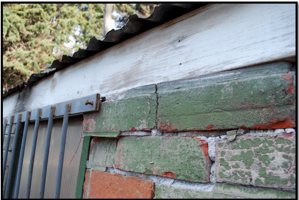
Photograph 7 Northeast walls top row of bricks separating.
