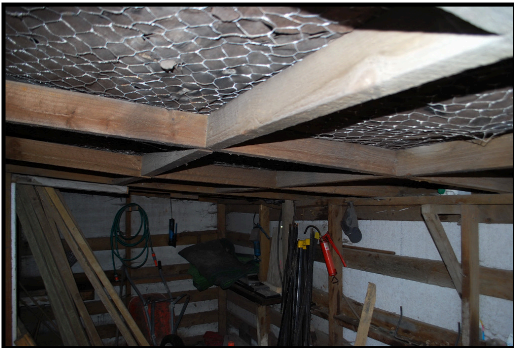
Photograph 12 Lean-to structures underside of roof.
