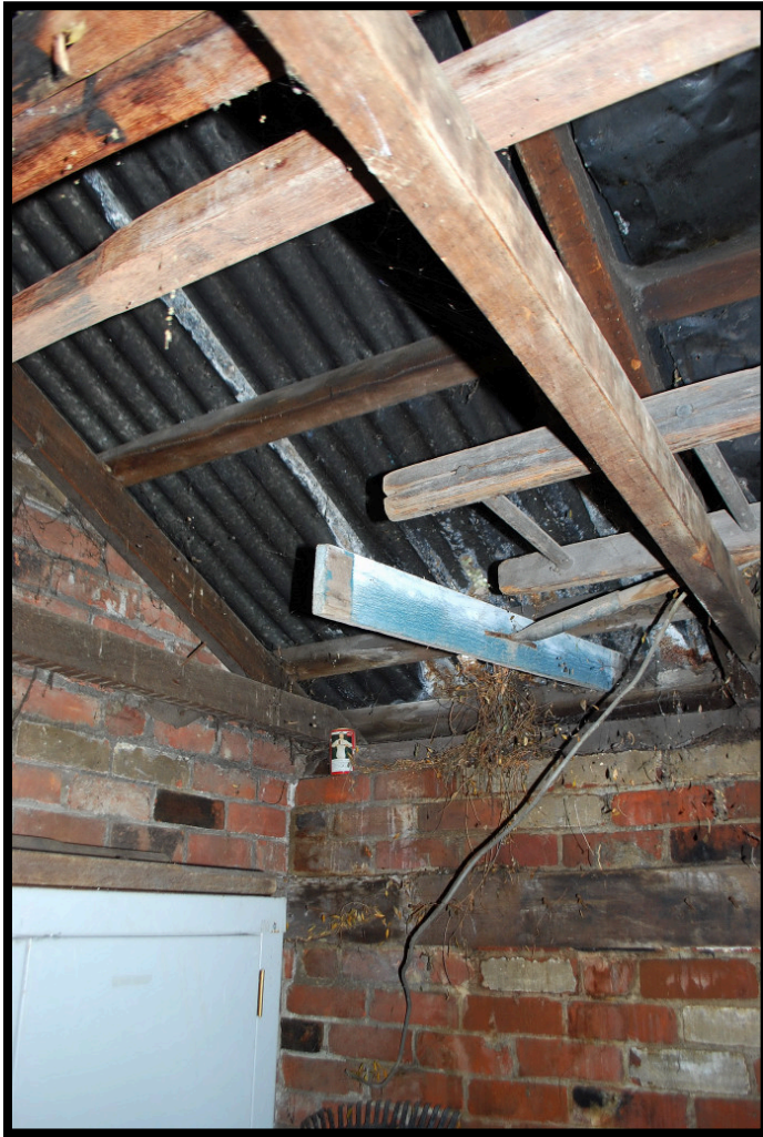
Photograph 11 Original structures underside of roof.
