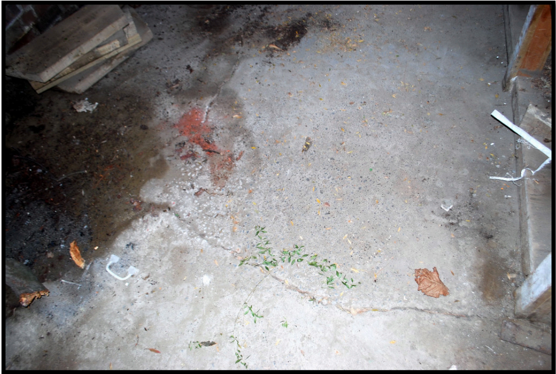
Photograph 3 Cracks in original structure's slab.
