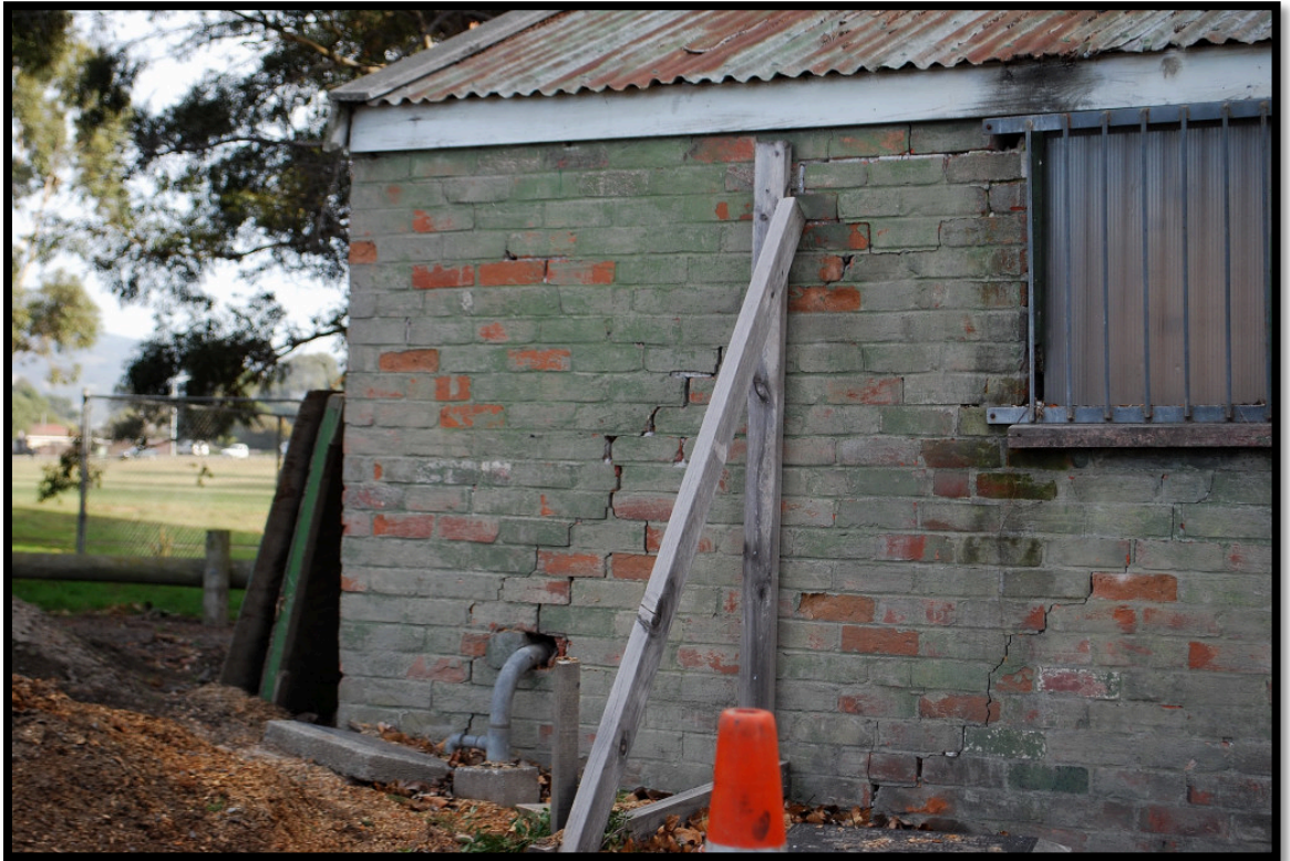
Photograph 5 Northeast corner of building showing extensive vertical and horizontal cracking along brickwork joints.
