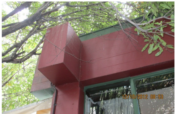
Typical view of the top external concrete beam at the corner of the building.
