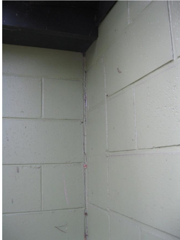
Photograph 7 Cracking at construction joint 2.
