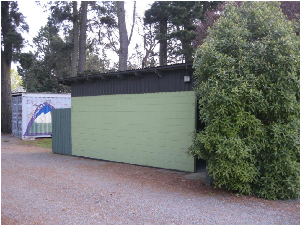
Photograph 2 Eastern elevation showing timber stud over concrete masonry wall.
