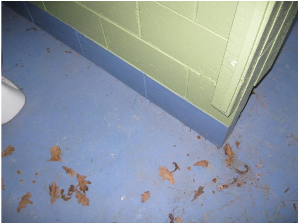
Photograph 8 Concrete floor slab.
