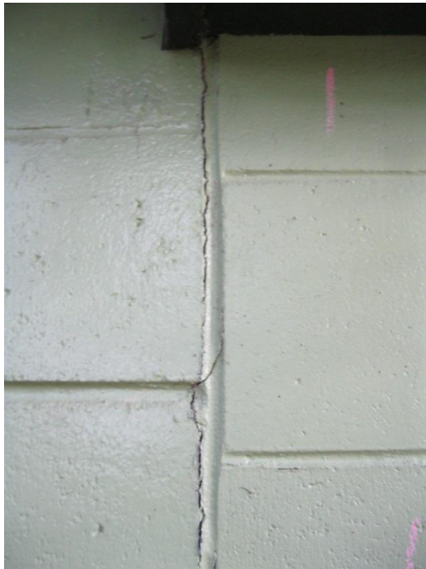
Photograph 6 Cracking at construction joint.
