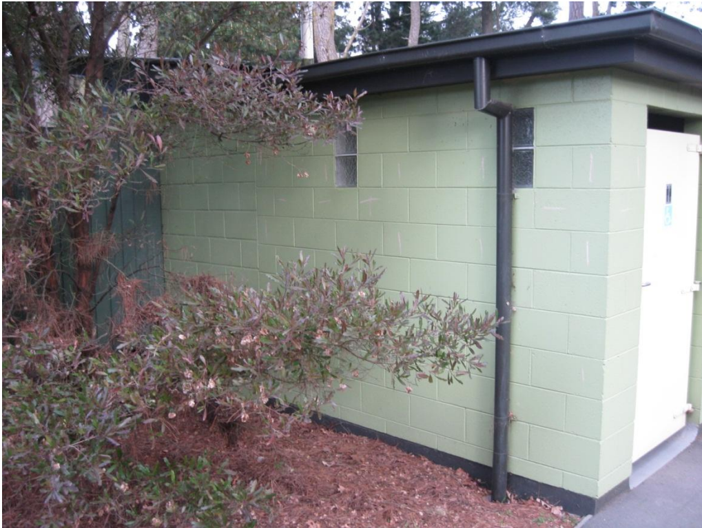
Photograph 3 View of the toilet block from the north.
