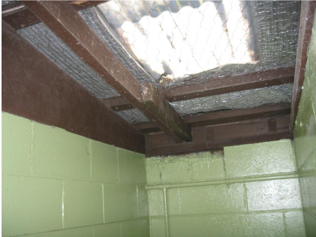
Photograph 5 Mono-pitch roof structure.
