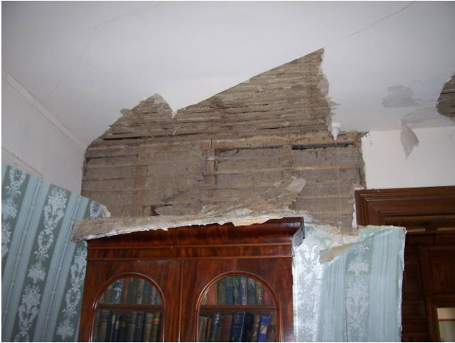
Lath and plaster wall and ceiling delamination in study
