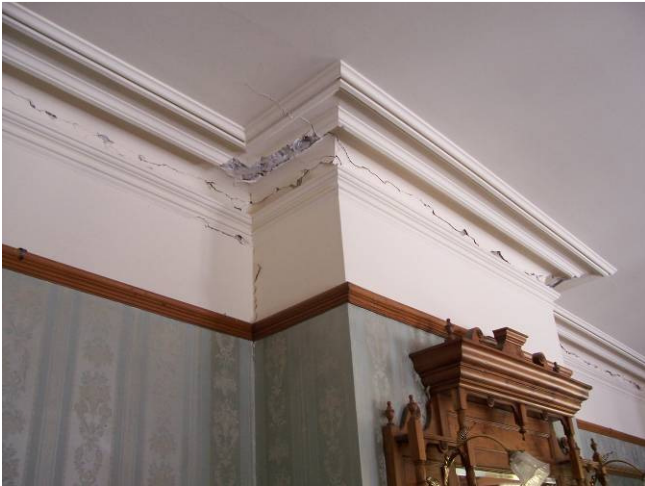
Cracking to drawing room scotia
