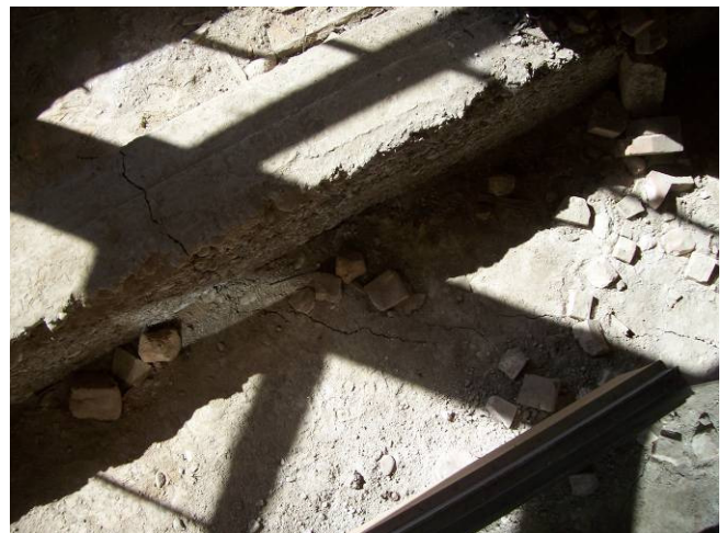
Ground crack extending under morning room bay window
