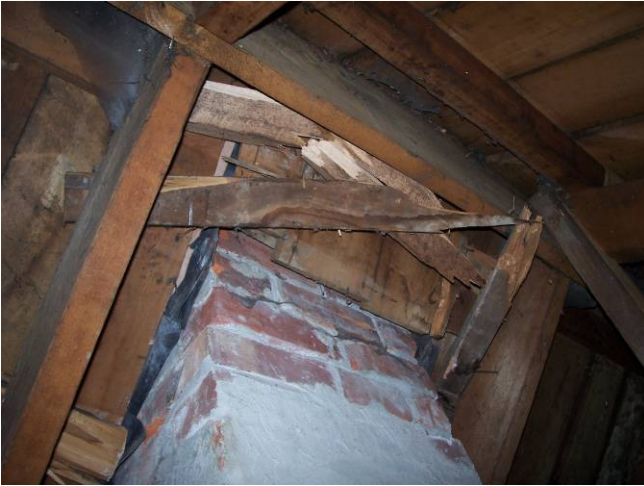
Localised damage to roof framing from chimney
