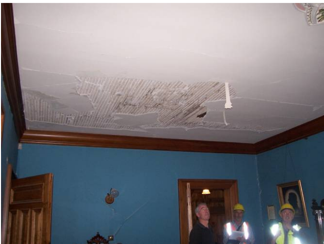
Lath and plaster ceiling delamination in dining room
