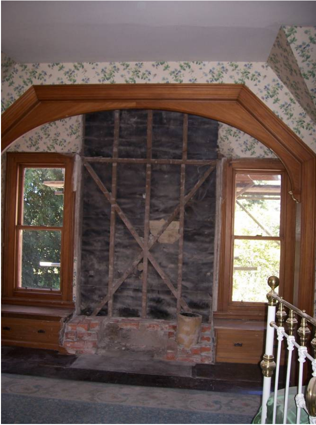
Collapse of chimney 2 breast at first floor
