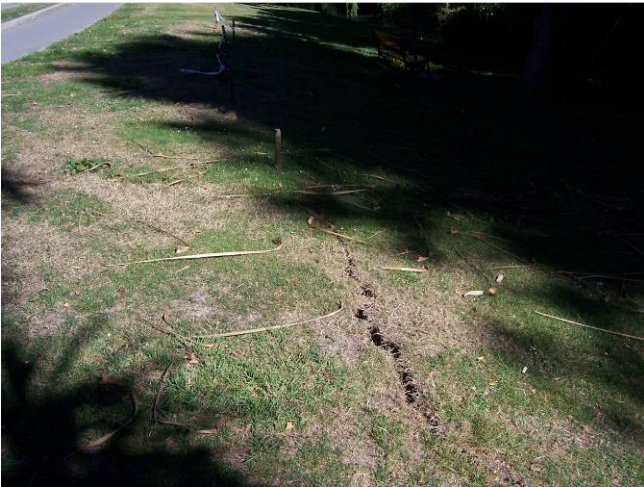
Ground cracking between path and stream
