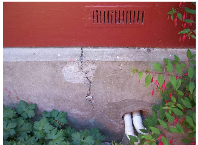
Minor isolated cracking to foundation wall
