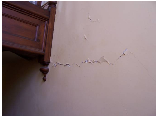
Cracking to lath and plaster walls at rear stair well
