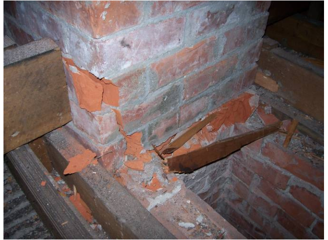
Damage to base of chimney 6
