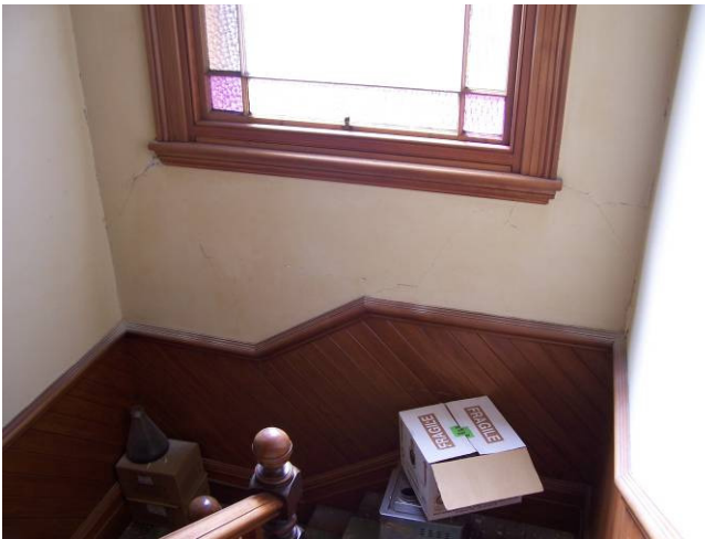
Cracking to lath and plaster walls at rear stair well
