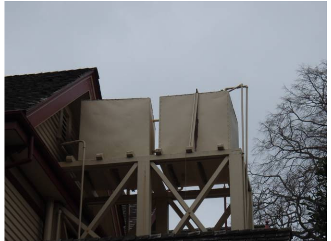
Displaced water tanks
