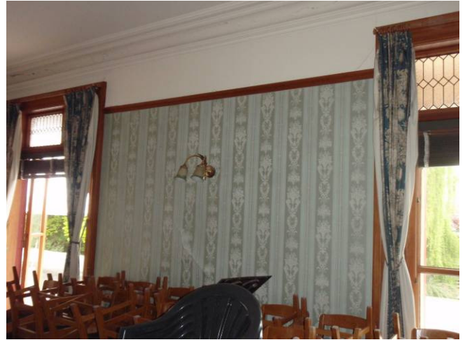
Diagonal cracking to lath and plaster wall in drawing room
