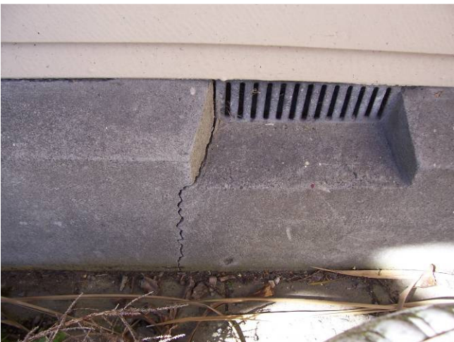
Minor isolated cracking to foundation wall
