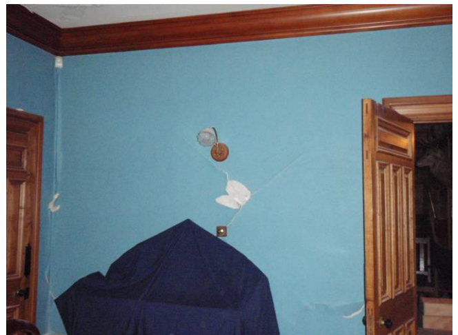
Diagonal cracking to lath and plaster wall in dining room
