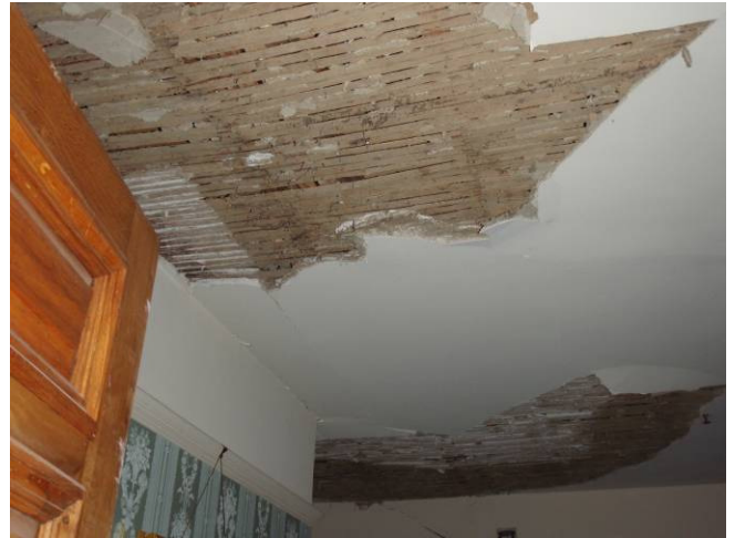
Lath and plaster ceiling delamination in study
