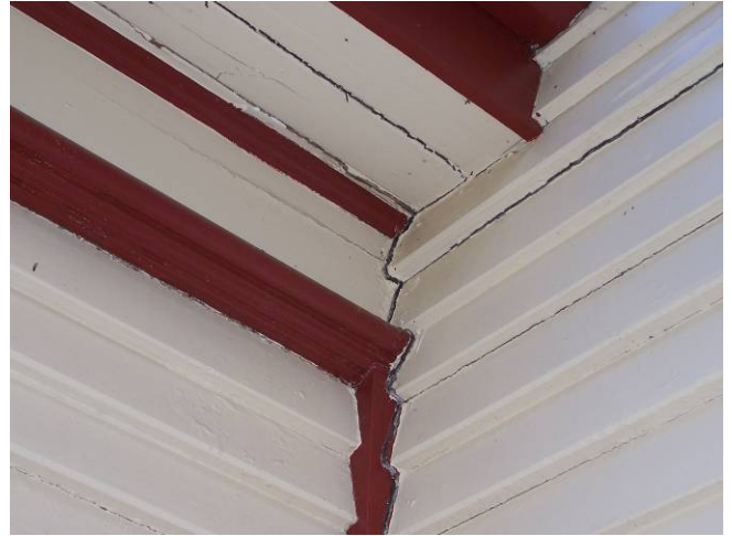
Separation between timber weatherboards
