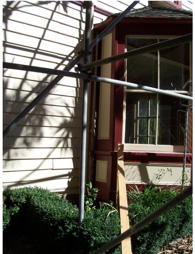
Morning room bay window pulled away from main building
