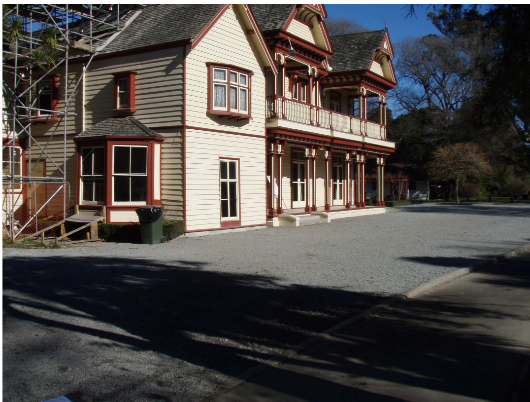
Figure 1: Northern side of Riccarton House. Damaged bay window in left of view.
