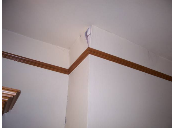
Damage to chimney 6 breast at first floor
