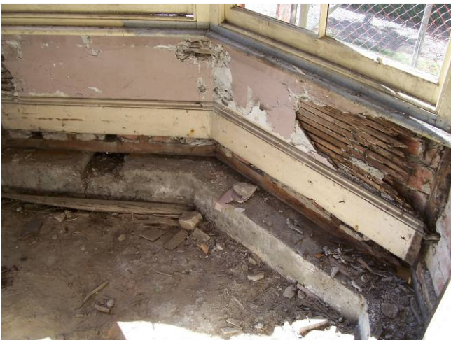
Morning room bay window from inside
