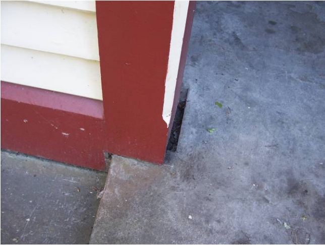
Rear porch framing displaced from concrete landing
