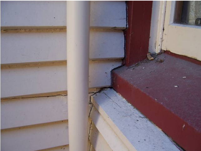
Separation between timber weatherboards
