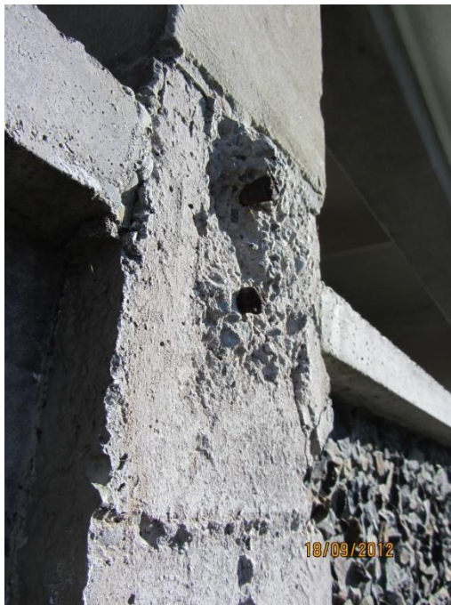
Photo 15: Close up view from photo 14 showing the exposed reinforcing at the top of the column
