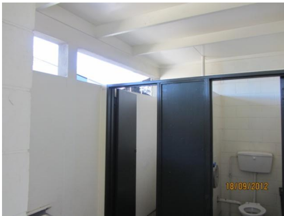
Photo 11: Interior view of womens toilet (2)
