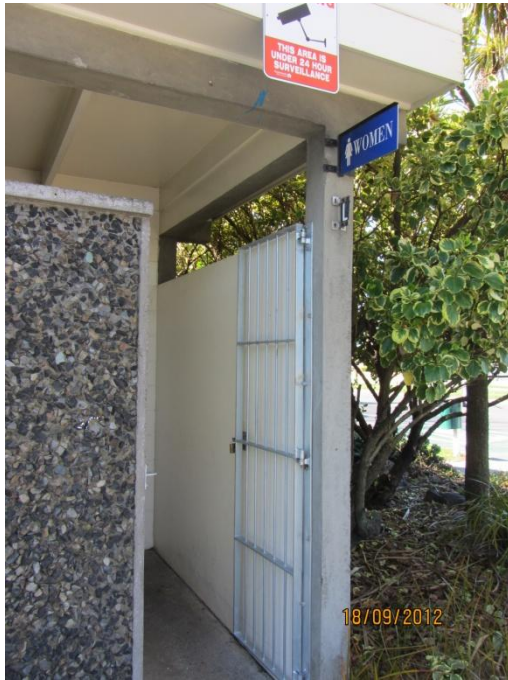
Photo 9: Entrance to womens toilet
