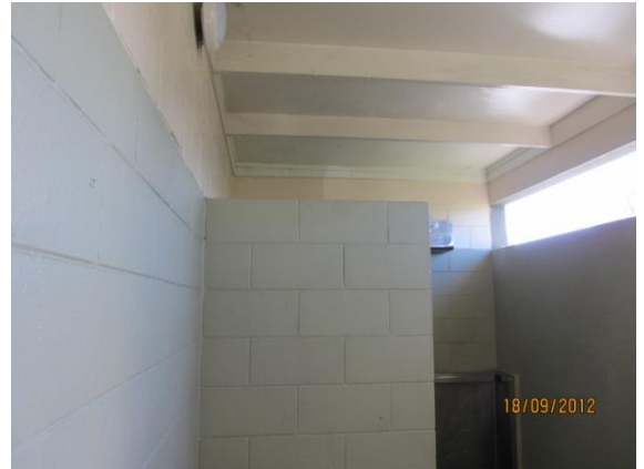
Photo 8: Interior view of mens toilet (3)
