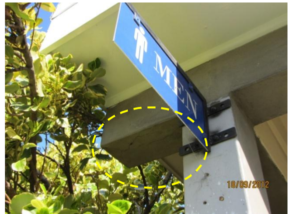
Photo 12: View of cracking on the underside of the cantilever concrete beam (1)
