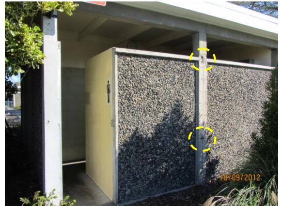
Photo 14: Mens toilet wall showing centre column with damage
