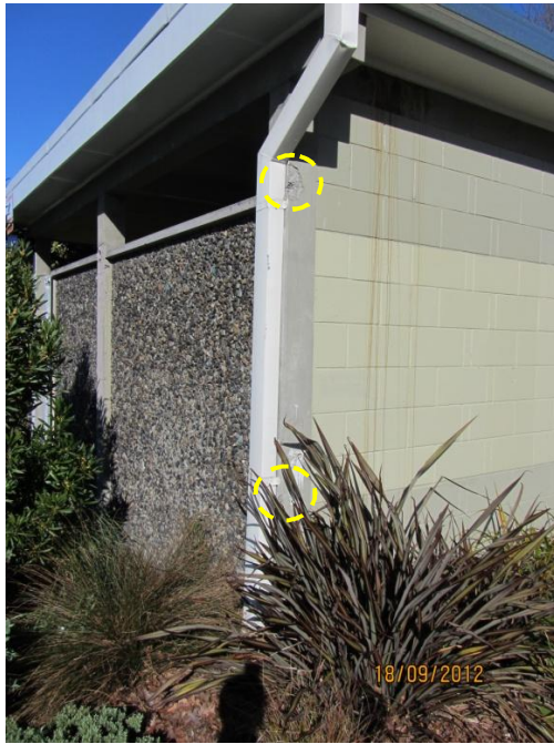
Photo 17: View of concrete column on the northwest corner, showing locations of damage
