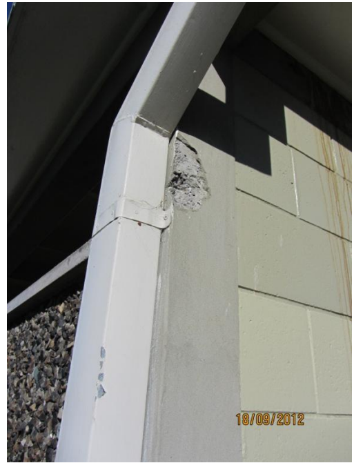
Photo 18: Close up view from photo 17 showing spalled grout near the top of the column
