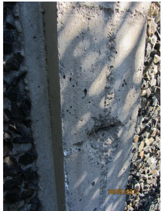
Photo 16: Close up view from photo 14 showing damage near the bottom of the column
