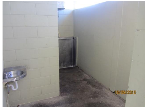
Photo 6: Interior view of mens toilet (1)
