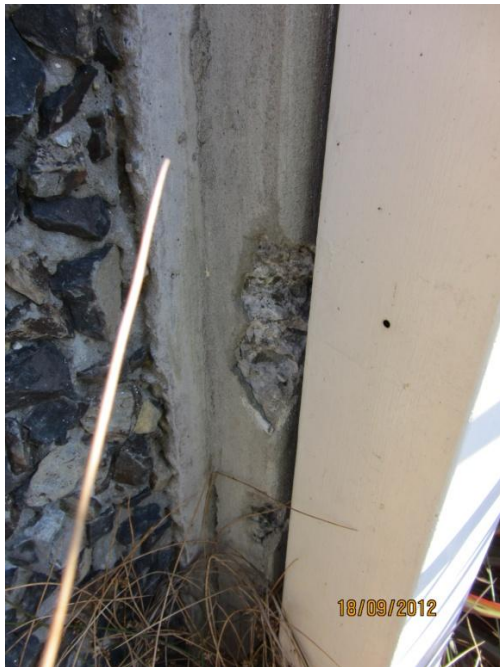
Photo 19: Close up view from photo 17 showing spalled grout near the bottom of the column
