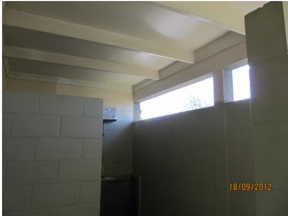
Photo 7: Interior view of the mens toilet (2)
