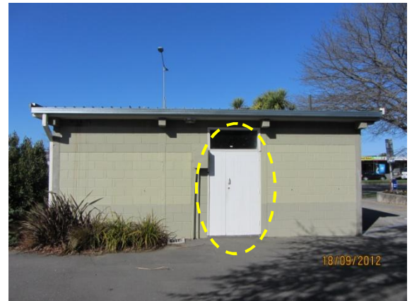
Photo 4: West Elevation, showing service doorway that could not be entered during the visual inspections
