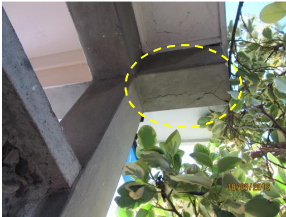
Photo 13: View of cracking on the underside of the cantilever concrete beam (2)
