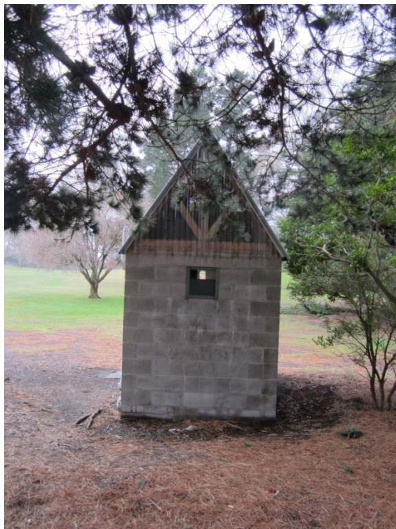
Photograph 2 View of the toilet from the south.
