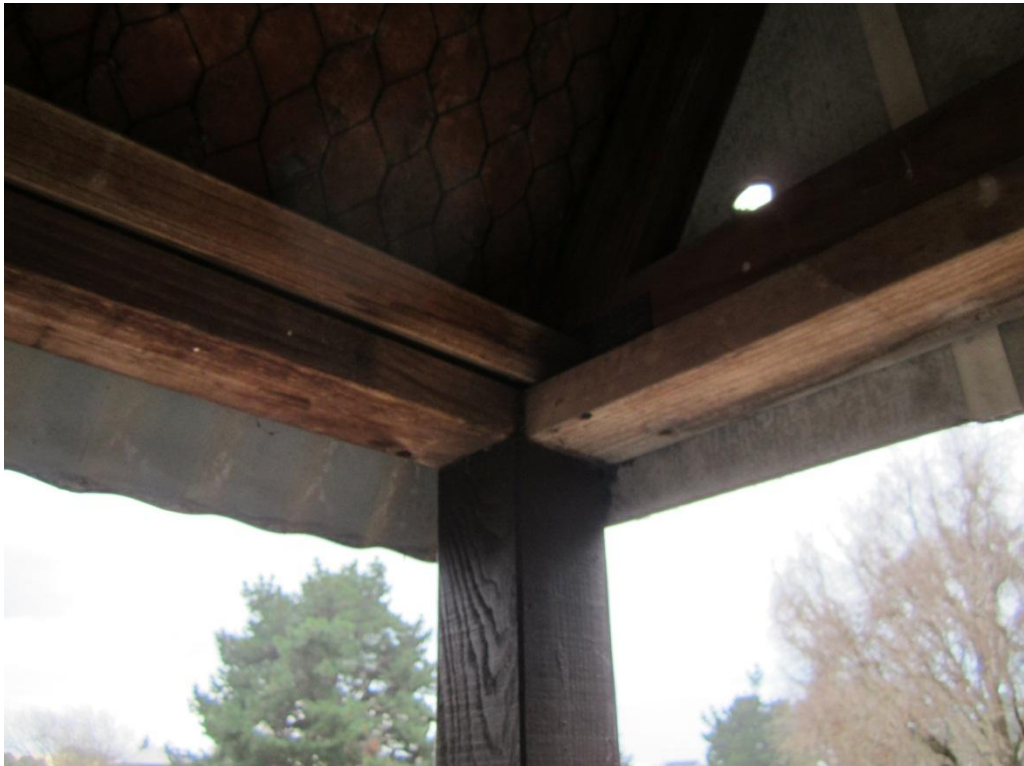
Photograph 4 90mm x 90mm timber post supporting roof truss.
