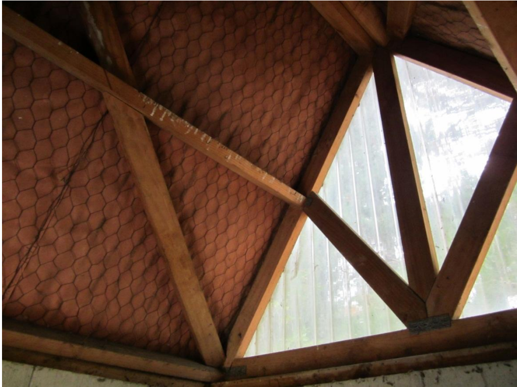
Photograph 3 Roof structure showing truss, purlins and diagonal brace.
