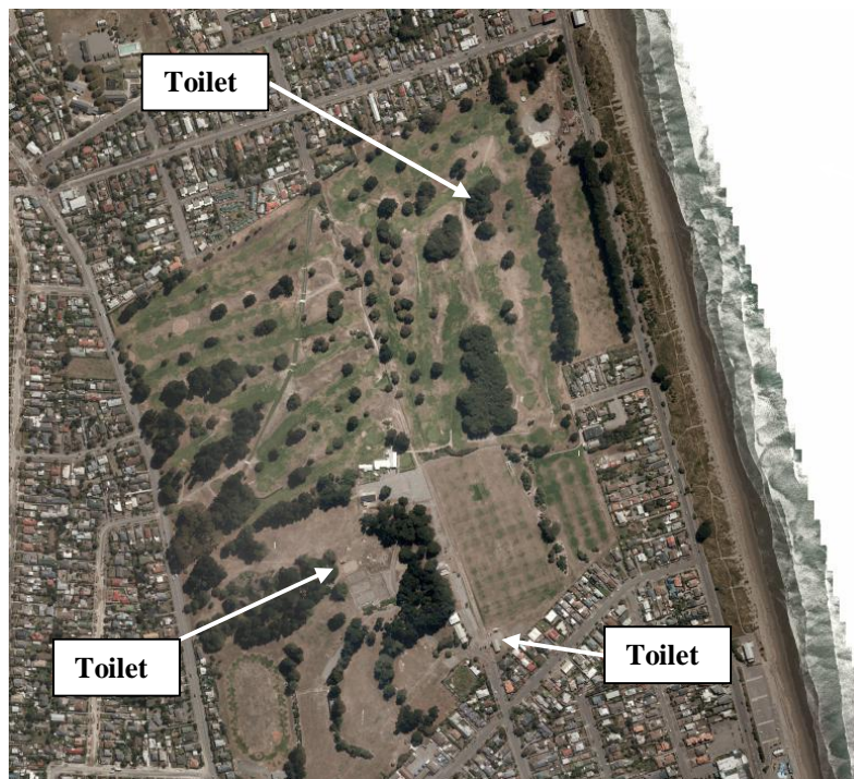
Figure 3 Post February 2011 Earthquake Aerial Photography 2
