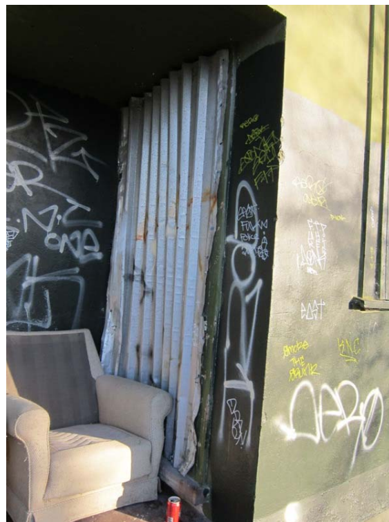
Photo 20: Entrance to building boarded up with corrugated metal sheeting.
