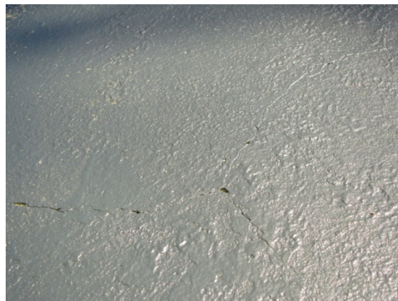
Photo 23: Crack in plaster on north wall has been painted over.
