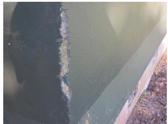
Photo 24: Existing impact damage to wall on northwest corner.
