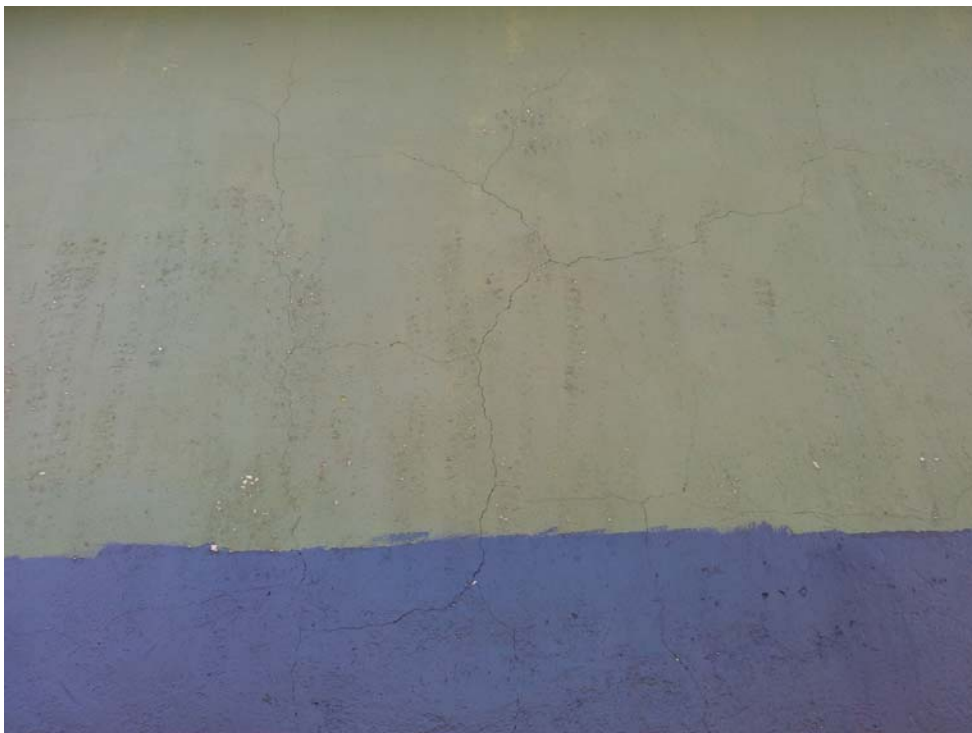
■ Figure 10 - Observed cracks in the wall
