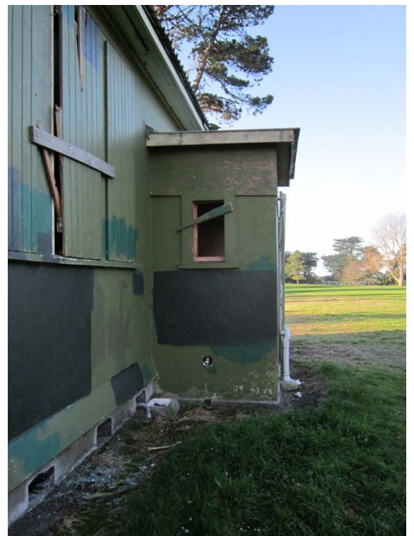
Photo 12: Lower section of building on southeast corner.
