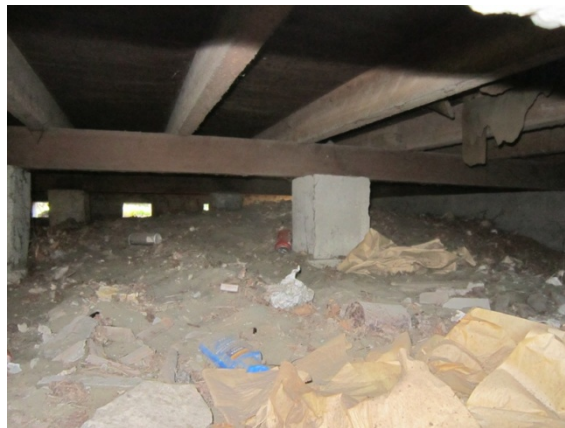
Photo 7: Timber floor supported by timber joists and bearers, resting on concrete blocks on ground.
