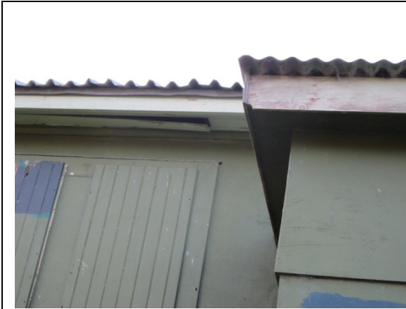
Photo 13: Timber edge beam on south side.
