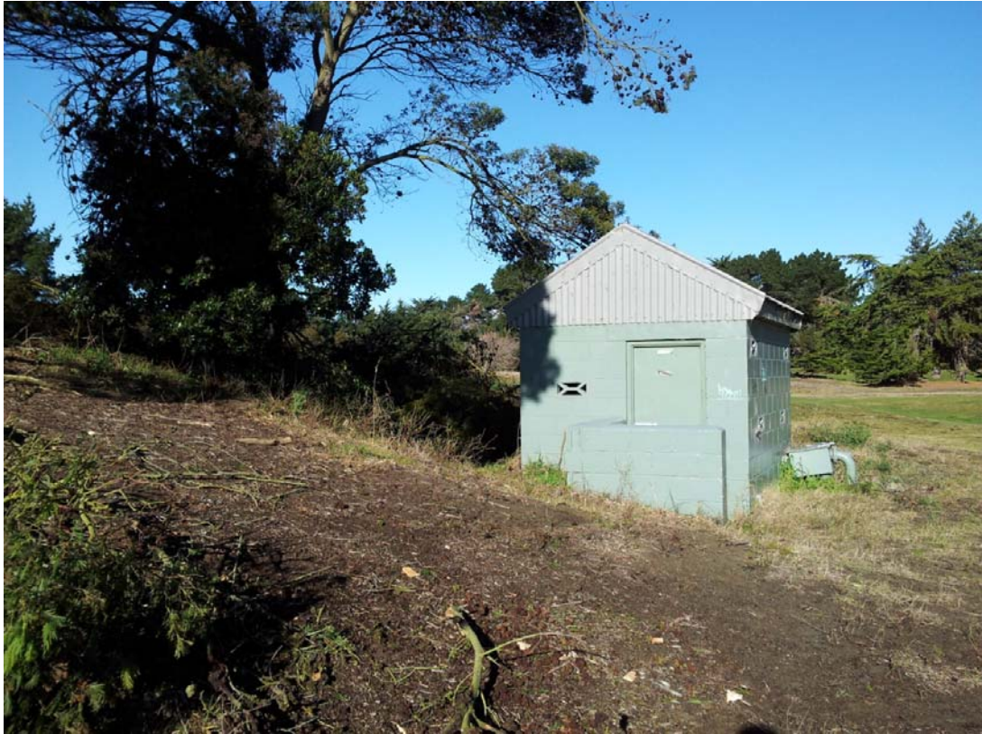
■ Figure 8 - Overview of the building (northern elevation)
