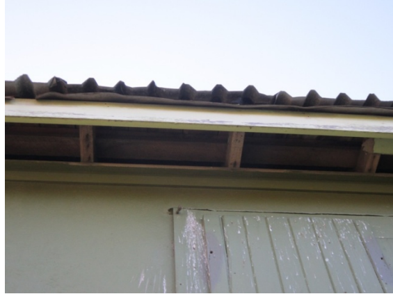
Photo 5: Soffit on south side with timber members missing.
