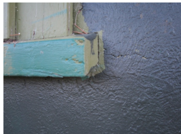
Photo 16: Crack in plaster on east wall by timber windowsill has been painted over.
