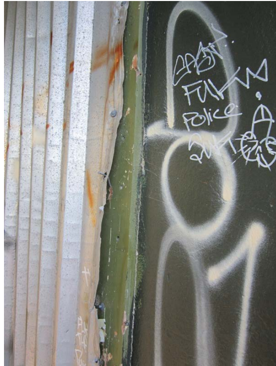
Photo 21: Corrugated metal sheeting over entrance secured with screws into timber doorframe.
