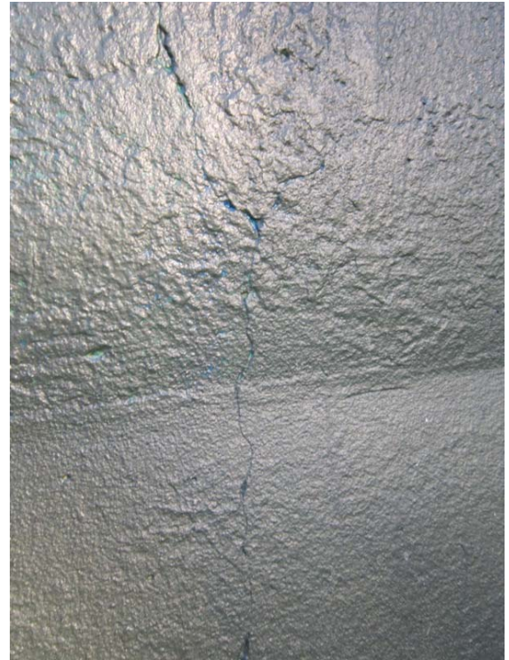
Photo 22: Crack in plaster on north wall has been painted over.
