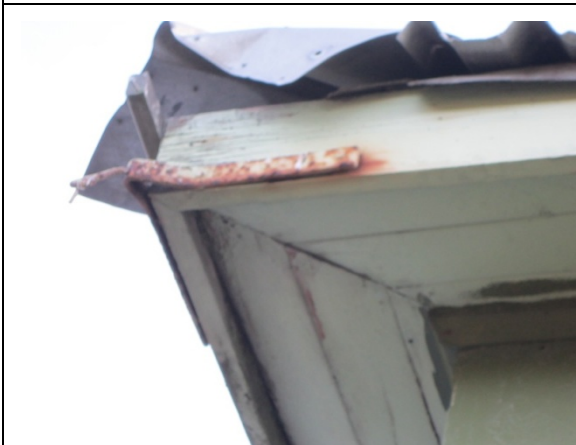
Photo 15: Rusted steel element on southeast corner of roof.
