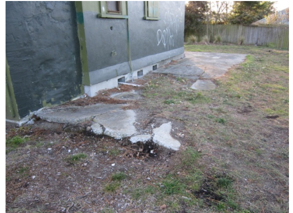
Photo 14: Concrete ground slab on east side.
