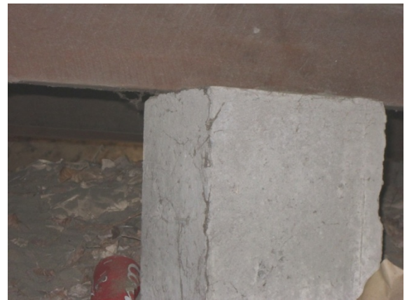
Photo 8: No visible connection between timber bearers and concrete block.
