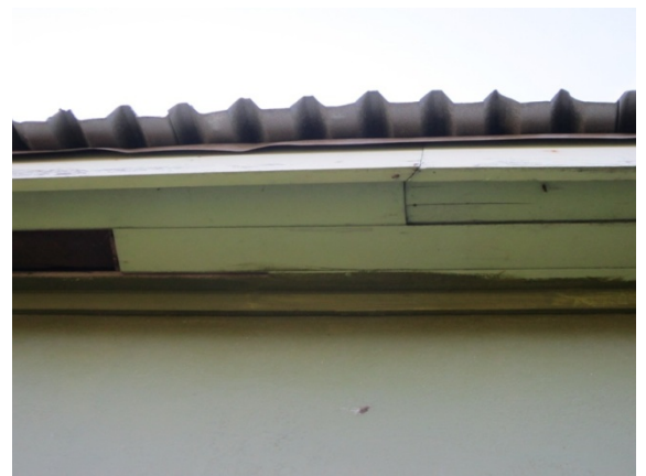
Photo 10: Soffit on south side.
