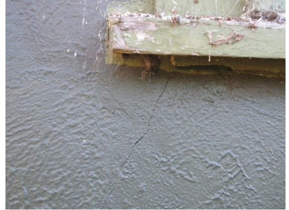
Photo 6: Crack in plaster on south concrete wall under timber windowsill has been painted over.
