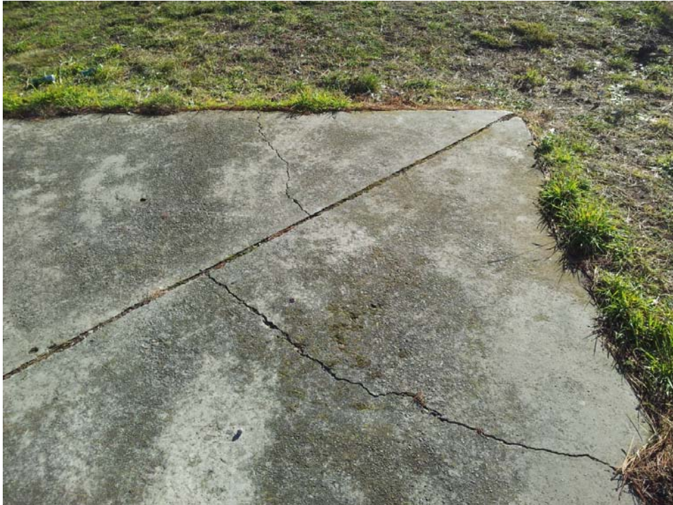
■ Figure 11 - Cracking in external concrete ground slab
