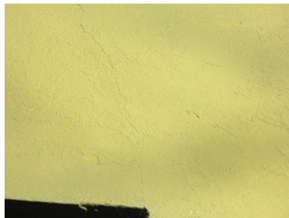
Photo 18: Crack in plaster on north wall has been painted over.
