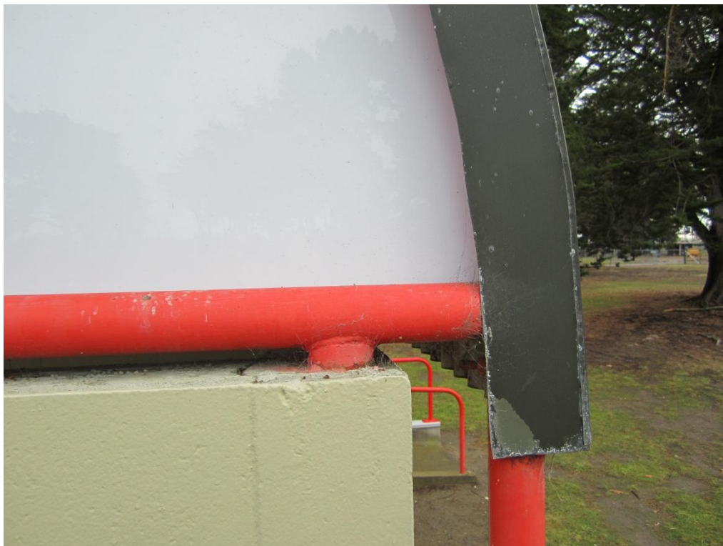
Photograph 4 Roof truss anchored into top of wall, column adjacent.
