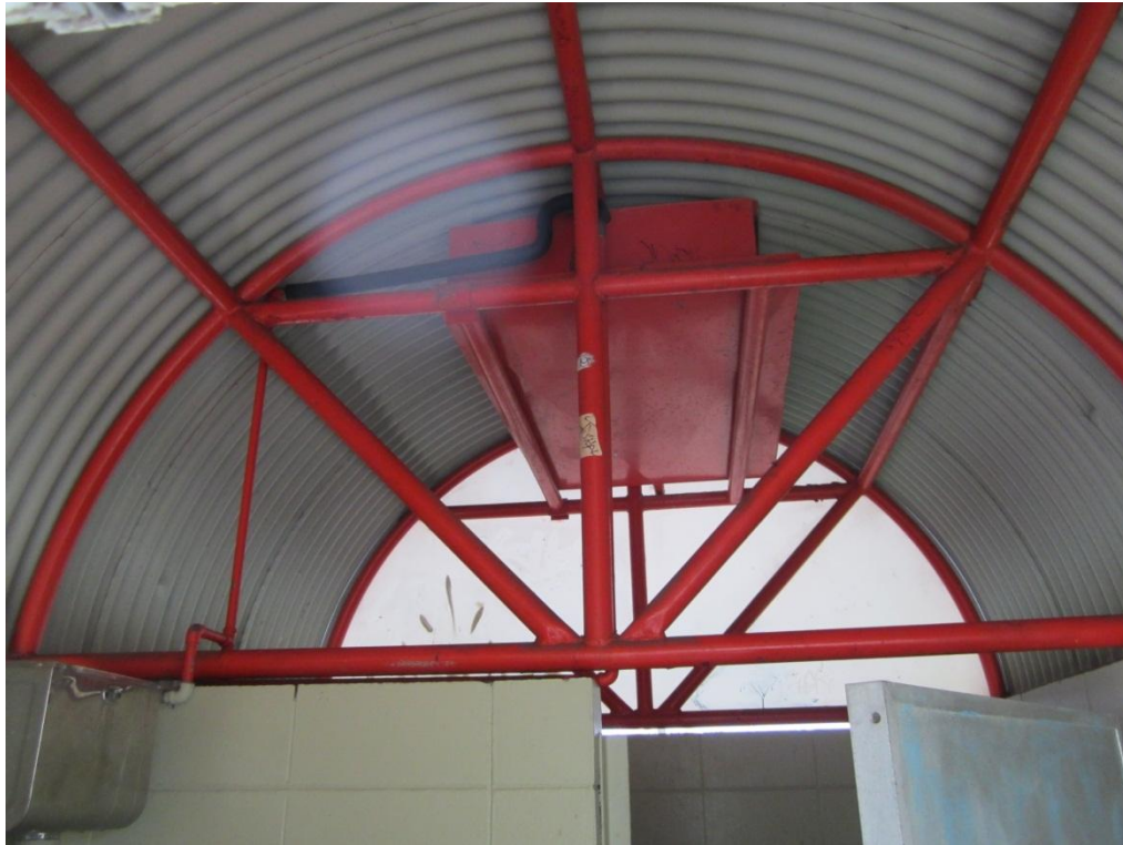
Photograph 3 Roof truss and purlins.
