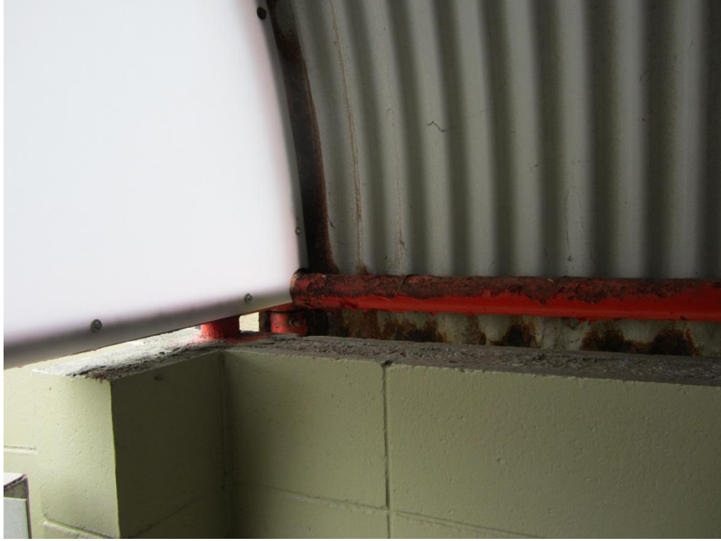
Photograph 5 Purlin with rust.
