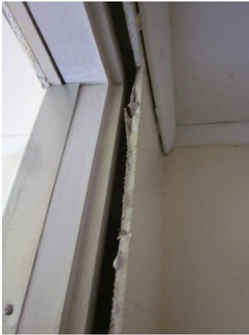
Photo 19: Plasterboard around internal door penetration
