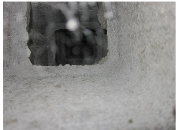
Photo 12: Photo up through the masonry block cell, above the ventilation point. Masonry walls partially filled
