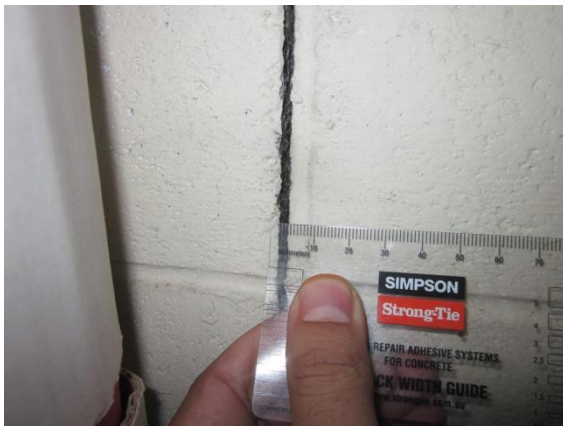
Photo 23: Cracking approximately 1.5 to 2mm in width
