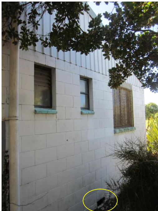
Photo 7: South end of the building with ventilation to the subfloor
