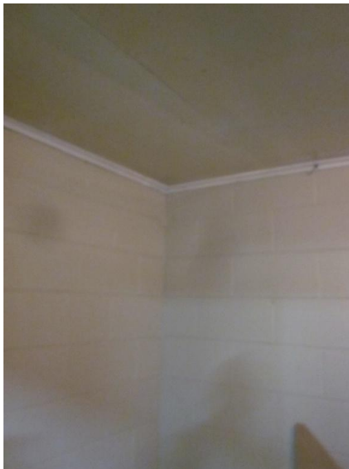
Photo 31: Storage room/ hall entry off main hall
