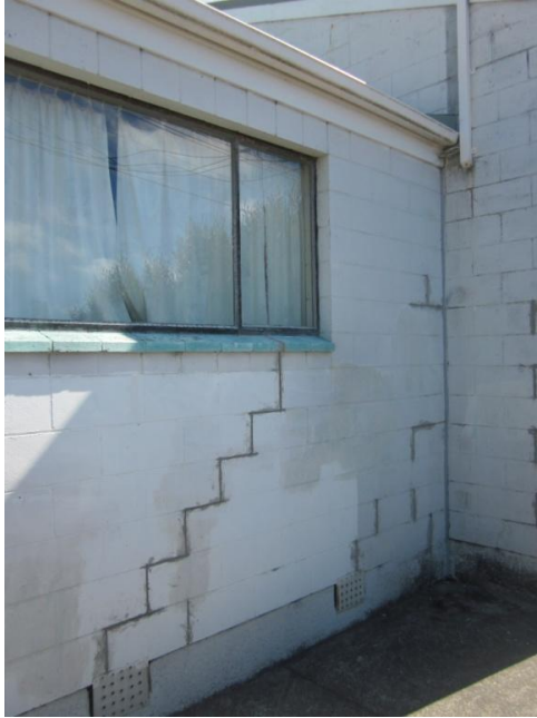
Photo 1: Repointed mortar joints on the Southeast amenities block
