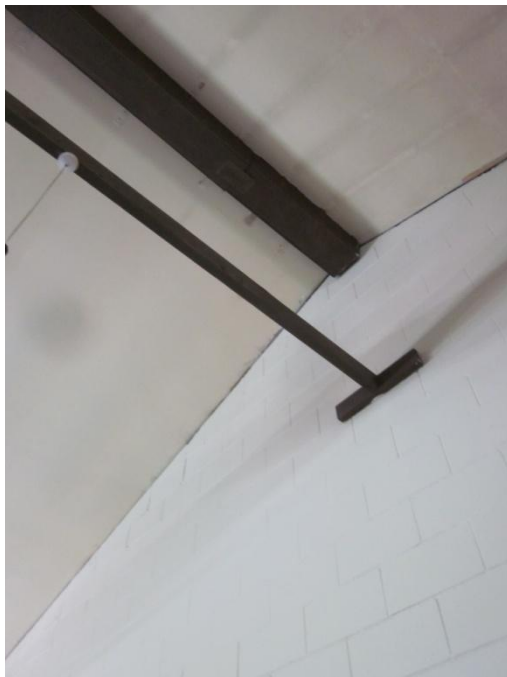
Photo 27: Perpendicular member connected to a timber end plate to the end masonry wall.
