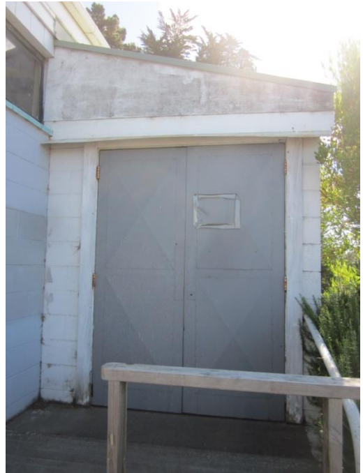
Photo 6: East storage room/ hall entry off the main hall
