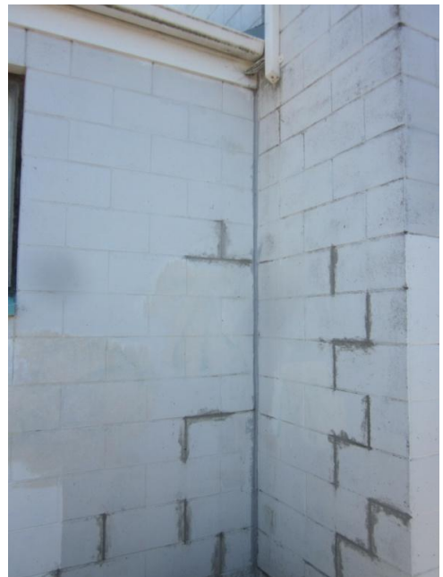
Photo 4: Mortar cracking around the building transition from amenities to main hall.
