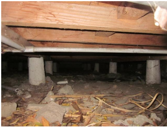
Photo 9: Subfloor timber particle board flooring on timber joists and bearers. Joist spacing approximately 600mm bearer and pile spacing approximately 2000mm
