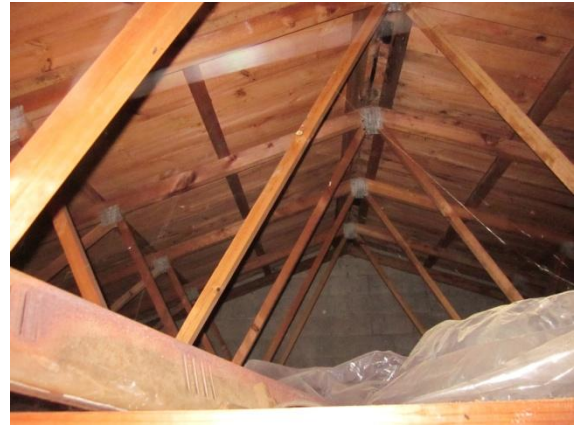
Photo 34: Timber tongue and groove roofing beneath corrugated metal. Supported by light timber trusses
