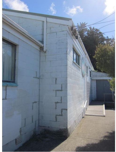
Photo 2: Repointed mortar joints on the Southeast amenities block
