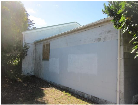
Photo 13: Southwest corner of the building with cracking below the window. See photos 14 and 21 to 23
