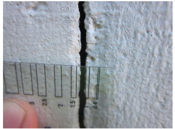
Photo 14: Block separation between masonry units
