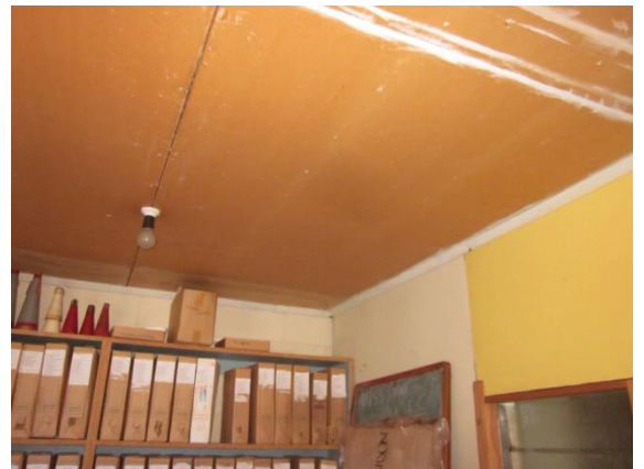
Photo 24: Plasterboard roofing in amenities area library
