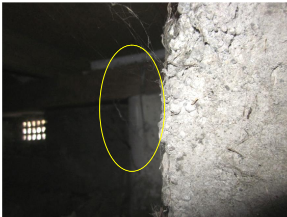
Photo 11: Bearers tied to concrete piles by wire
