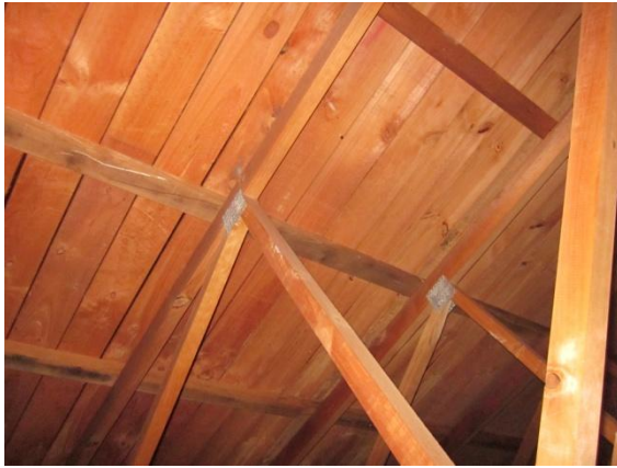
Photo 33: Roof structure above the amenities block
