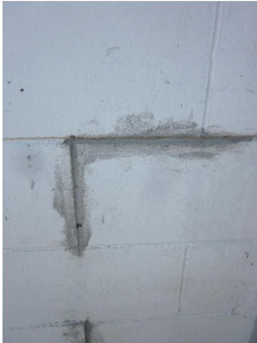
Photo 5: Repointed masonry, still to be painted
