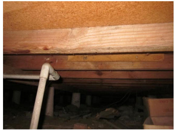
Photo 10: Particle board flooring
