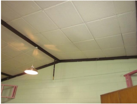
Photo 29: Structure of ceiling support unknown
