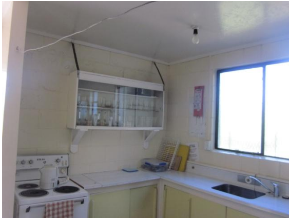
Photo 17: Amenities have masonry perimeter walls with light timber framed internal walls and plasterboard ceiling linings.
