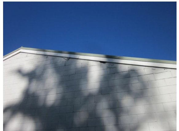
Photo 16: Spalling to the concrete infill along the gable end wall between blockwork and roof
