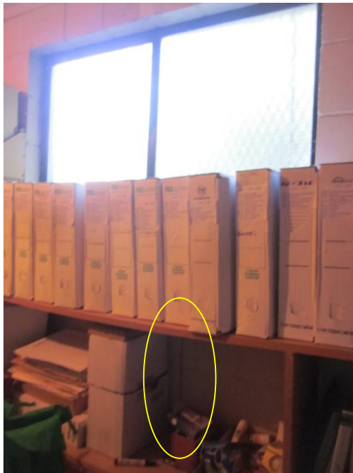
Photo 21: Cracking beneath south west window
