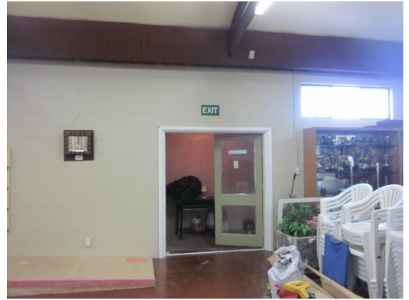
Photo 30: Entry/ storage room off the main hall. East wall
