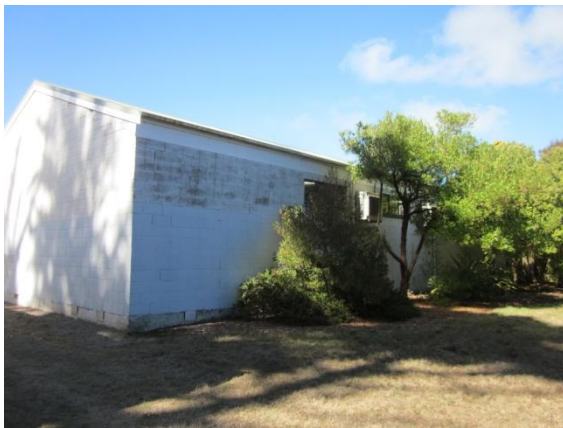
Photo 15: North west corner of the building
