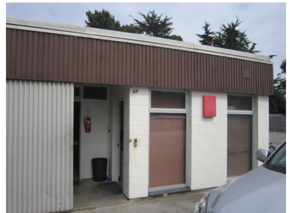
Photo 16: Entrance to office on east side of building
