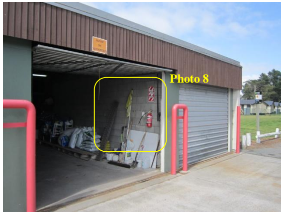
Photo 7: View of one of the entrances to the 3 bay garage
