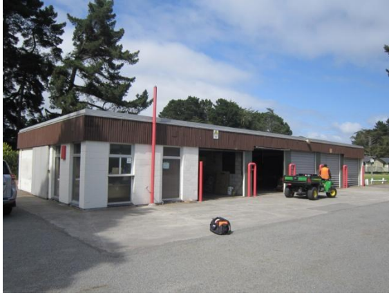
Photo 1: View of garage
