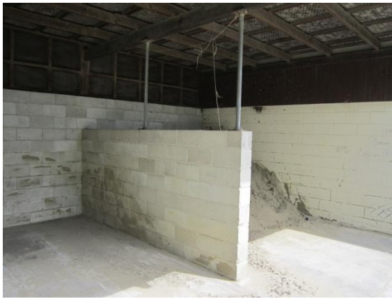
Photo 19: Interior view of soil storage area
