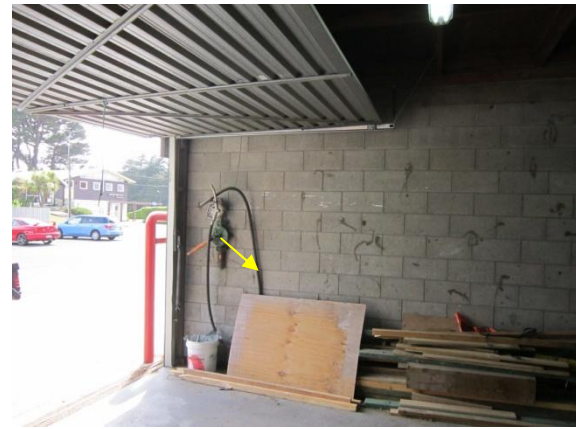
Photo 14: Masonry wall inside of 3 bay garage
