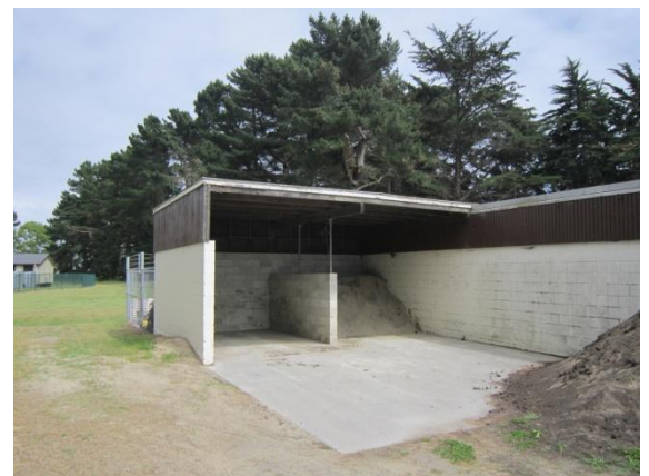
Photo 18: Soil storage area on South side of building
