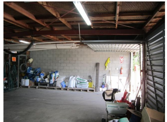
Photo 10: Interior view of 3 bay garage
