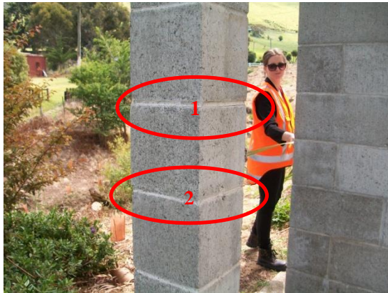
Photo 9: Western column masonry with minor cracking at two locations
