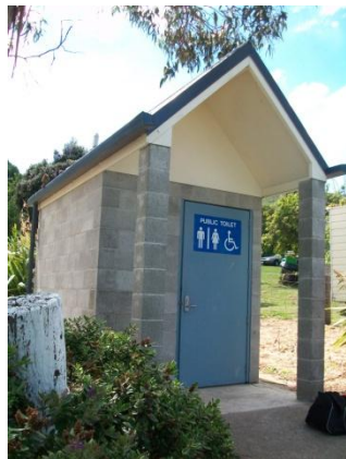
Photo 3: West and South elevation
