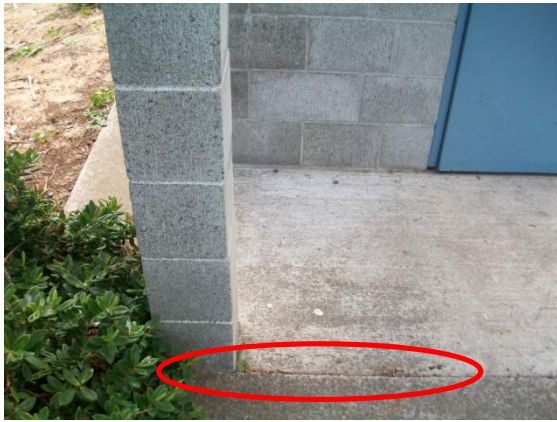
Photo 13: Displacement between foundation, column and pathway
