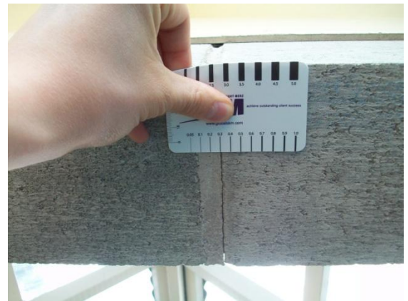
Photo 8: A maximum of 0.3mm cracking between masonry blocks above doorway (2)
