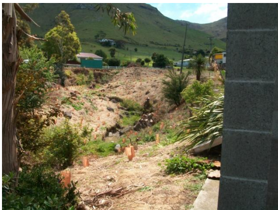
Photo 17: Slope and creek next to building
