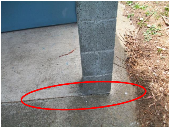
Photo 15: Displacement and cracking between foundation, column and pathway
