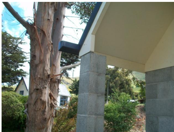
Photo 11: Displacement between columns and timber
