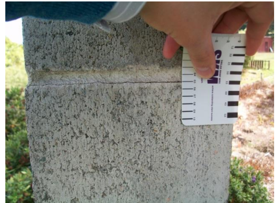
Photo 10: 0.5mm cracking between masonry blocks in the western column (1)
