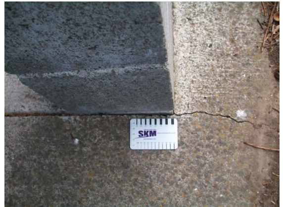
Photo 16: Size of displacement and cracking
