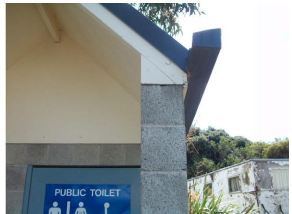
Photo 12: Displacement between columns and timber
