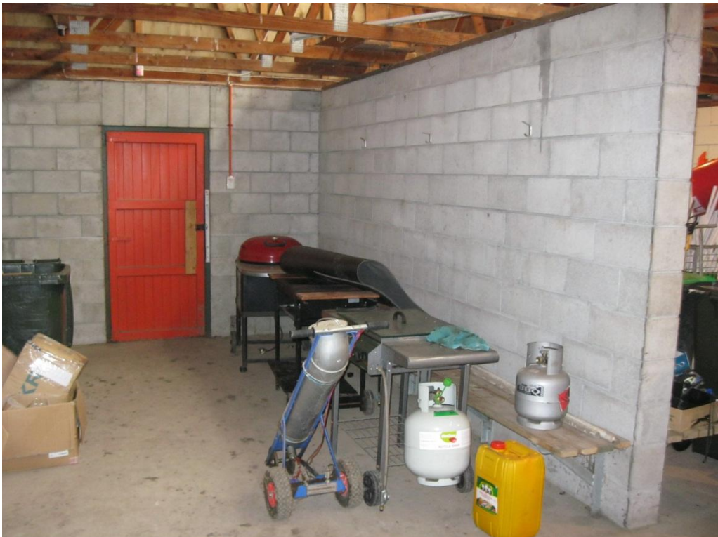
Photograph 6 Interior partition Wall.
