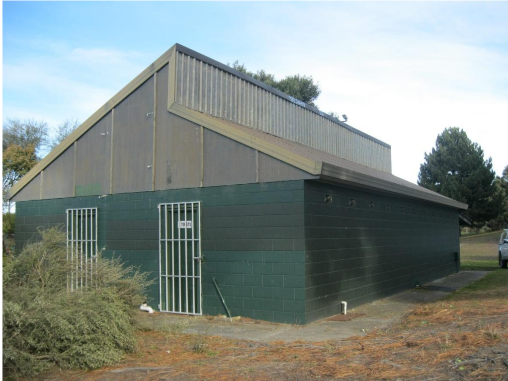
Photograph 1 View from the north.
