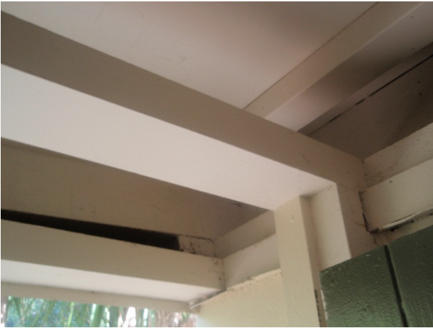
Photo 9: Door Head Restraint
