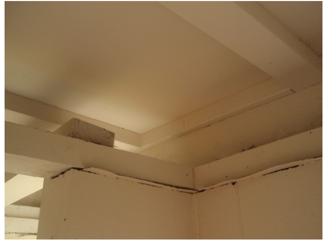
Photo 10: DPC beneath Wall Plate
