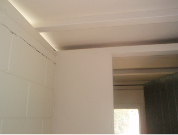
Photo 7: Roof and Wall Plate
