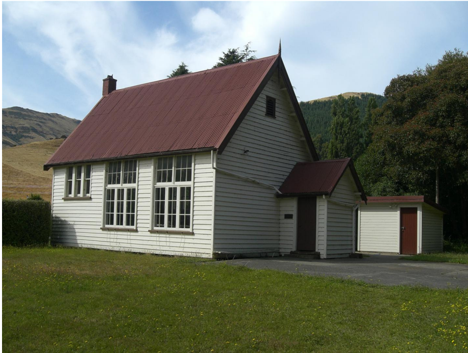
Photo 3: View of the building from the north
