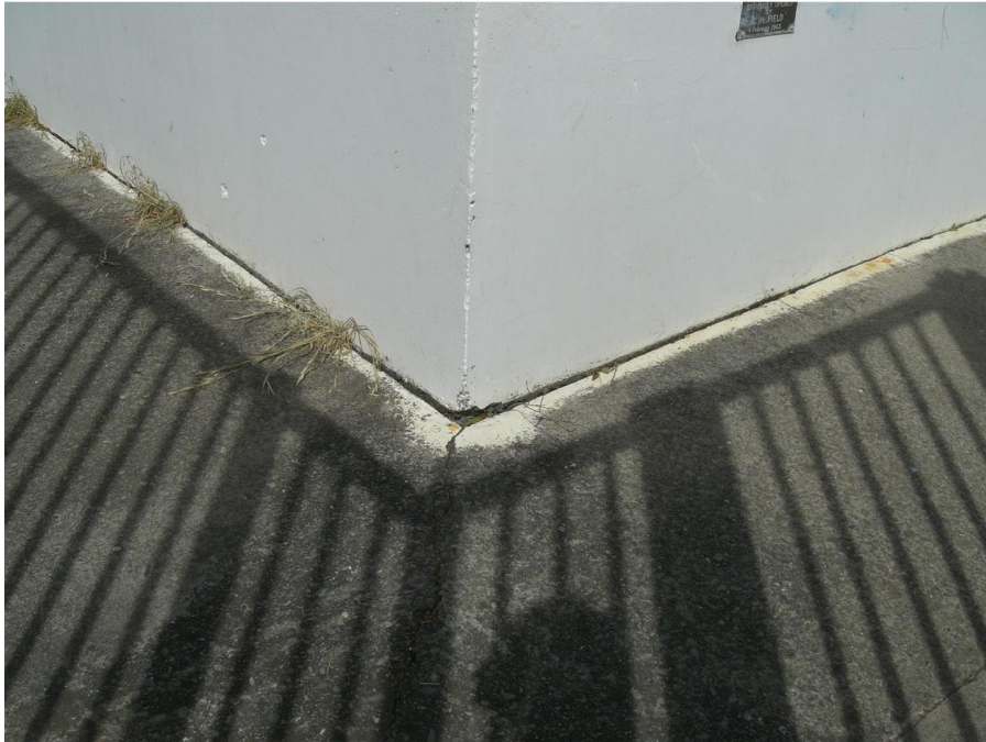
Photo 2: 10mm of pavement settlement around the north east corner of the swimming pool.
