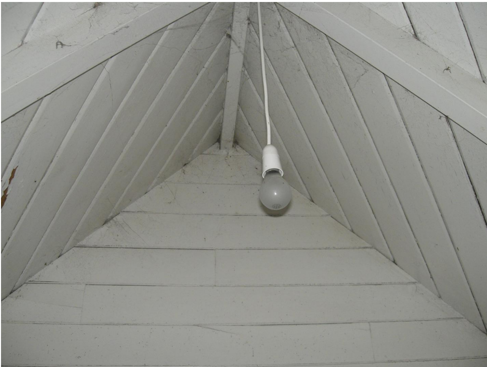
Photo 6: View of the tongue and groove ceiling and walls in the entrance area
