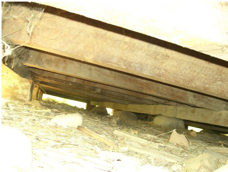
Photo 3: Foundation of the Community Hall.
