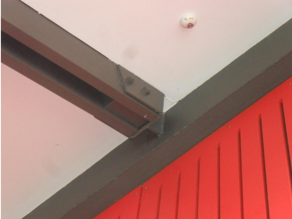
Photograph 19 Connection between in-situ concrete beam and timber rafters.
