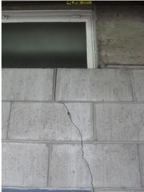
Photograph 23 Cracking in concrete masonry wall on eastern side of the building.
