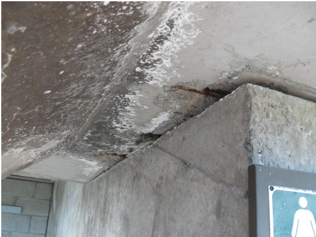
Photograph 14 Separation of the seating between the concrete beams supporting the grandstand and the northern concrete steps.
