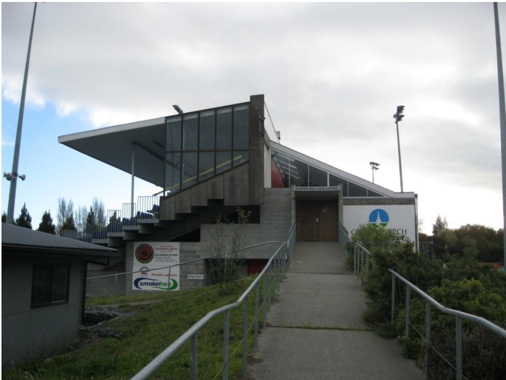
Photograph 2 Southern face of the Porritt Park Complex.
