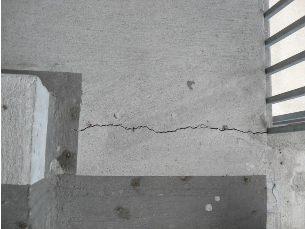
Photograph 15 Cracking in the in-situ floor slab in the middle of the grandstand.
