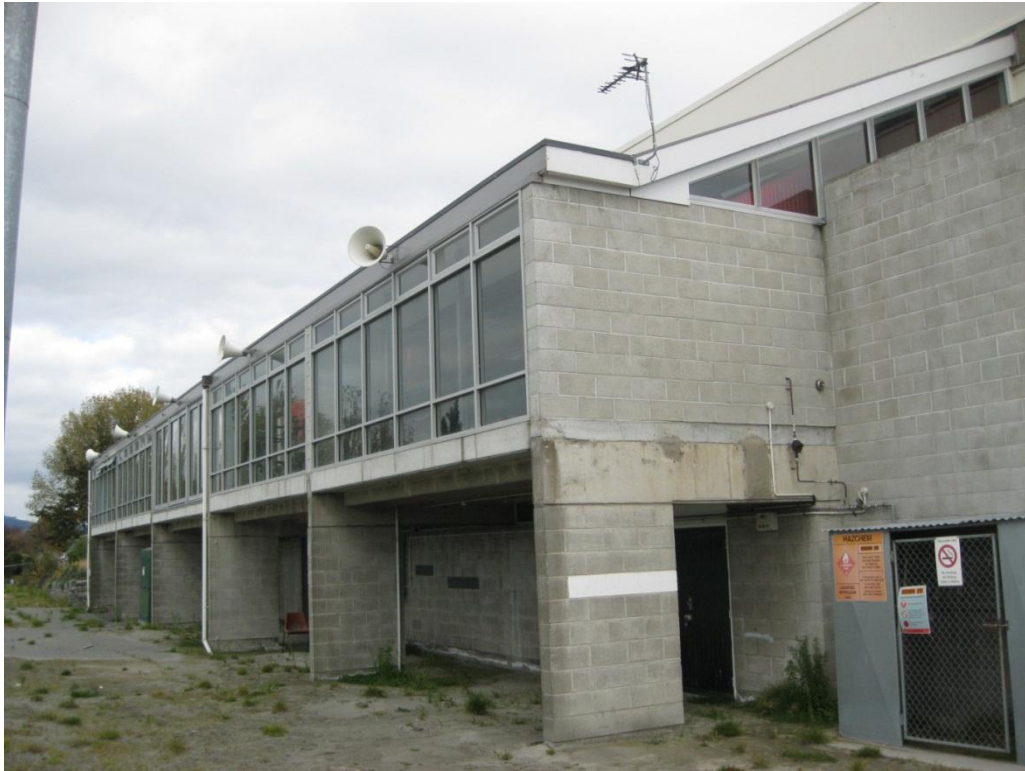
Photograph 5 Eastern face of the Porritt Park Complex.
