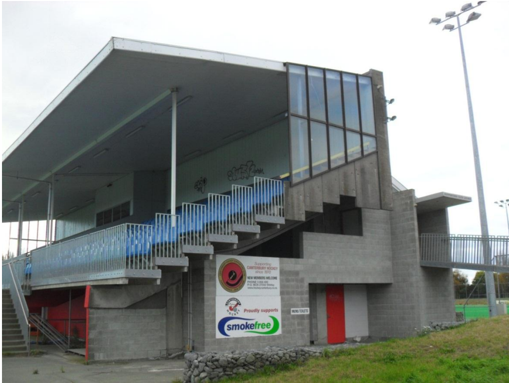
Photograph 11 Steel framed roof structure.
