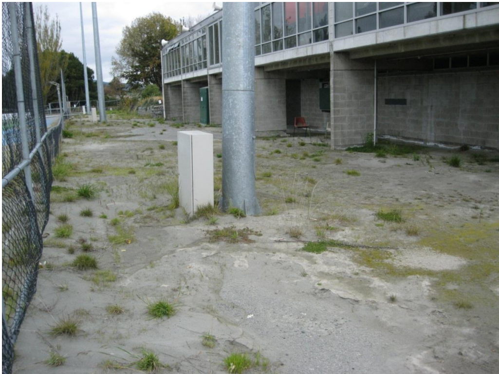
Photograph 6 Sand and silt on the ground east of the building due to extensive liquefaction.
