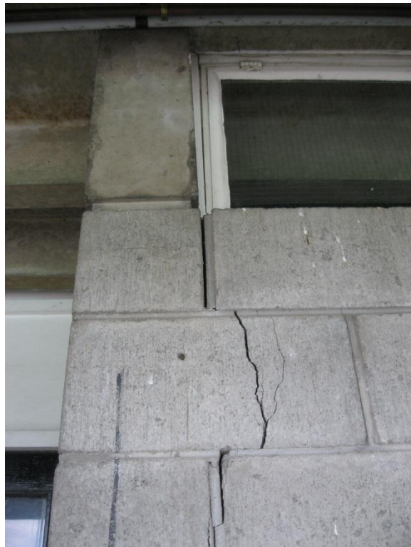
Photograph 8 Cracking in a concrete masonry wall along the eastern face of the building.
