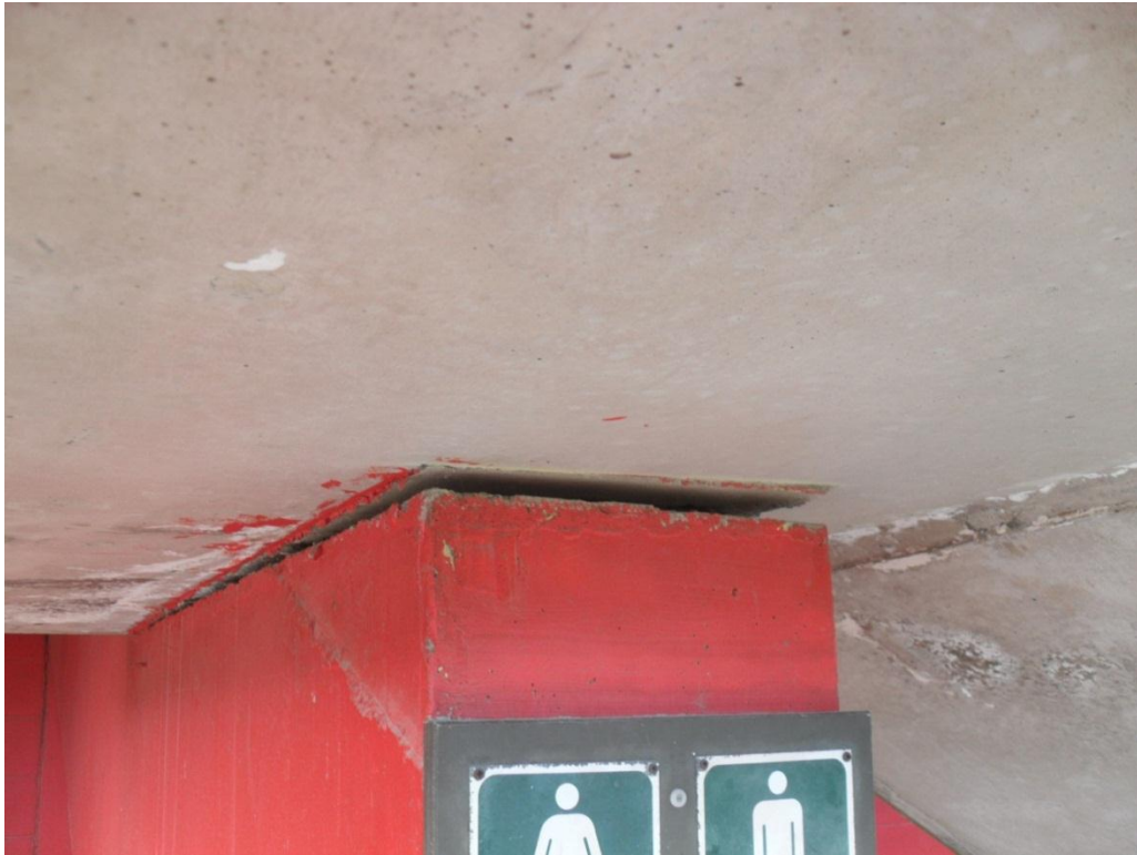
Photograph 13 Separation of the seating between the concrete beams supporting the grandstand and the southern concrete steps.
