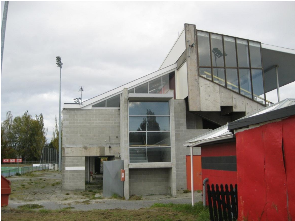
Photograph 4 Rear section of northern face of the Porritt Park Complex.
