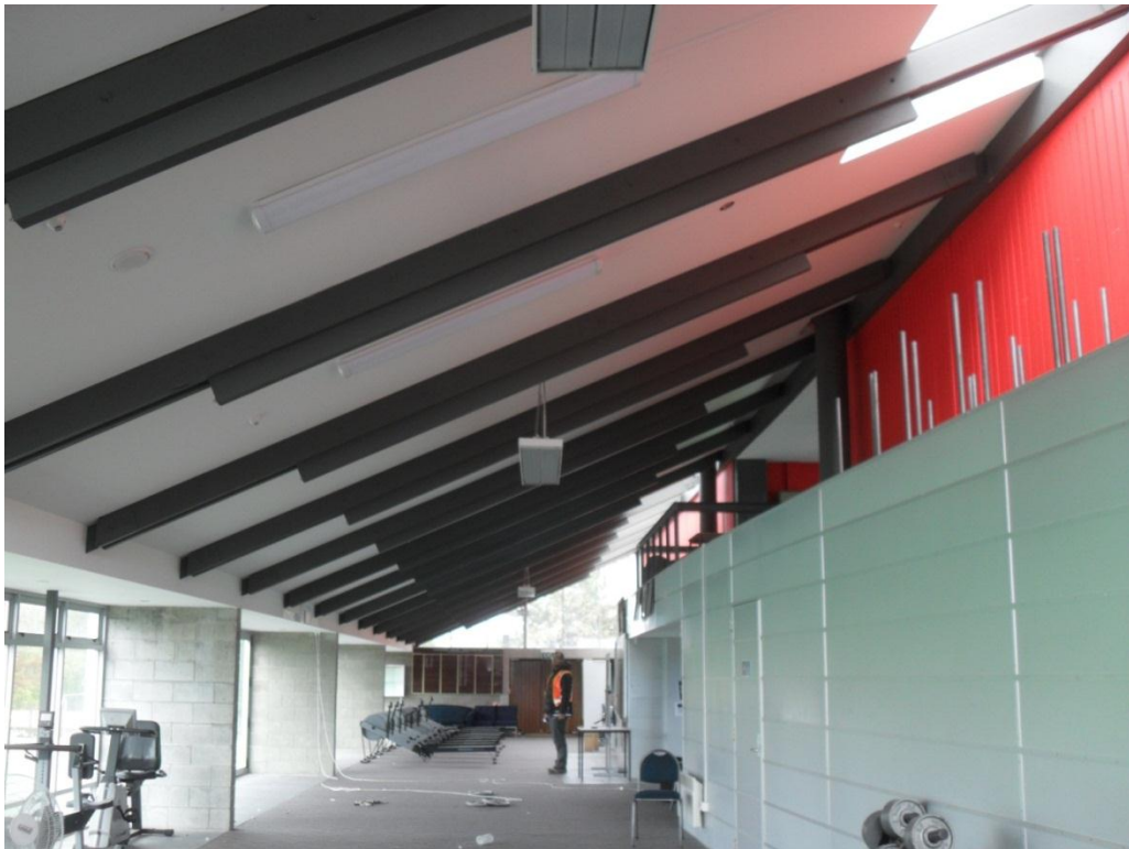
Photograph 18 Timber rafters supporting the roof along eastern half of the building.
