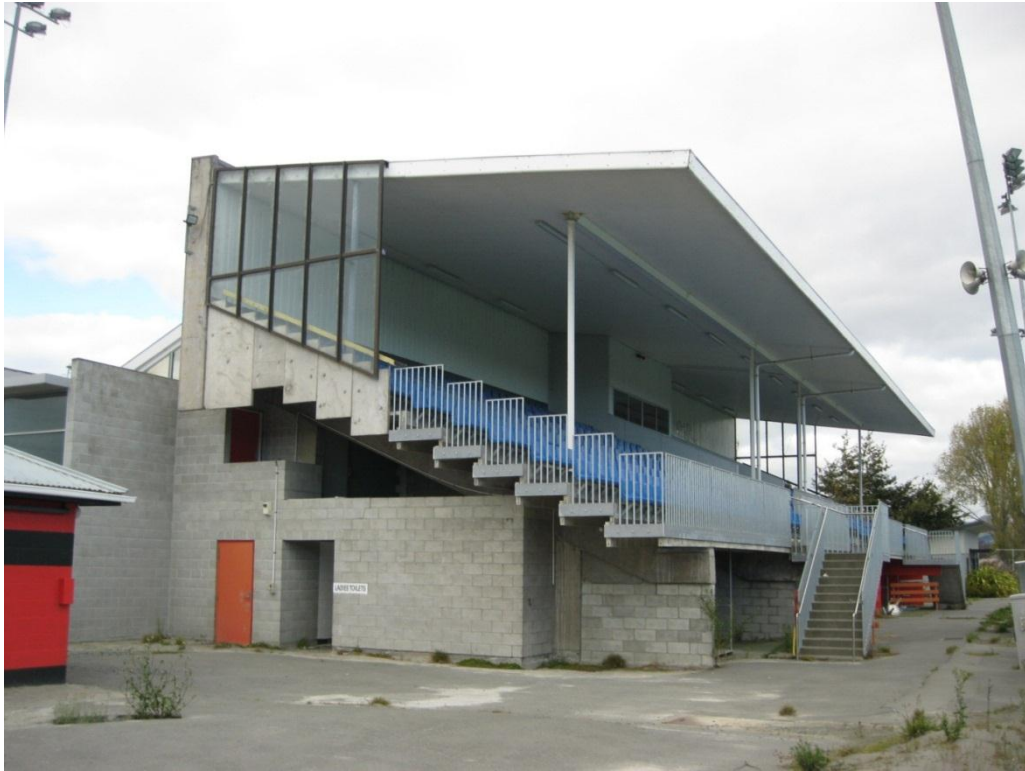
Photograph 3 Northern face of the Porritt Park Complex.
