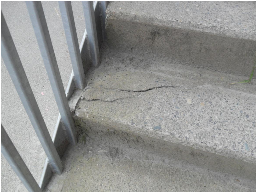
Photograph 12 Cracking in grandstand stairs along the western side of the grandstand.
