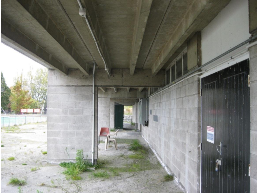
Photograph 7 Precast double tee flooring units.
