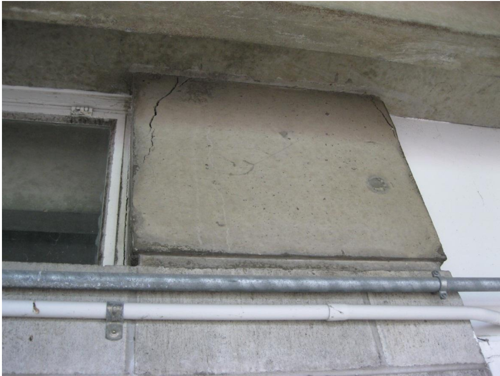
Photograph 21 Cracking in concrete beam supporting precast flooring units.
