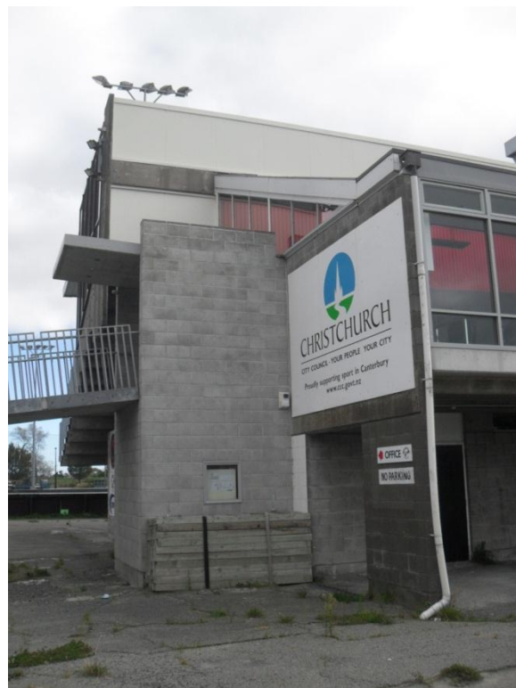
Photograph 10 Concrete masonry wall in the south-east corner of the building.
