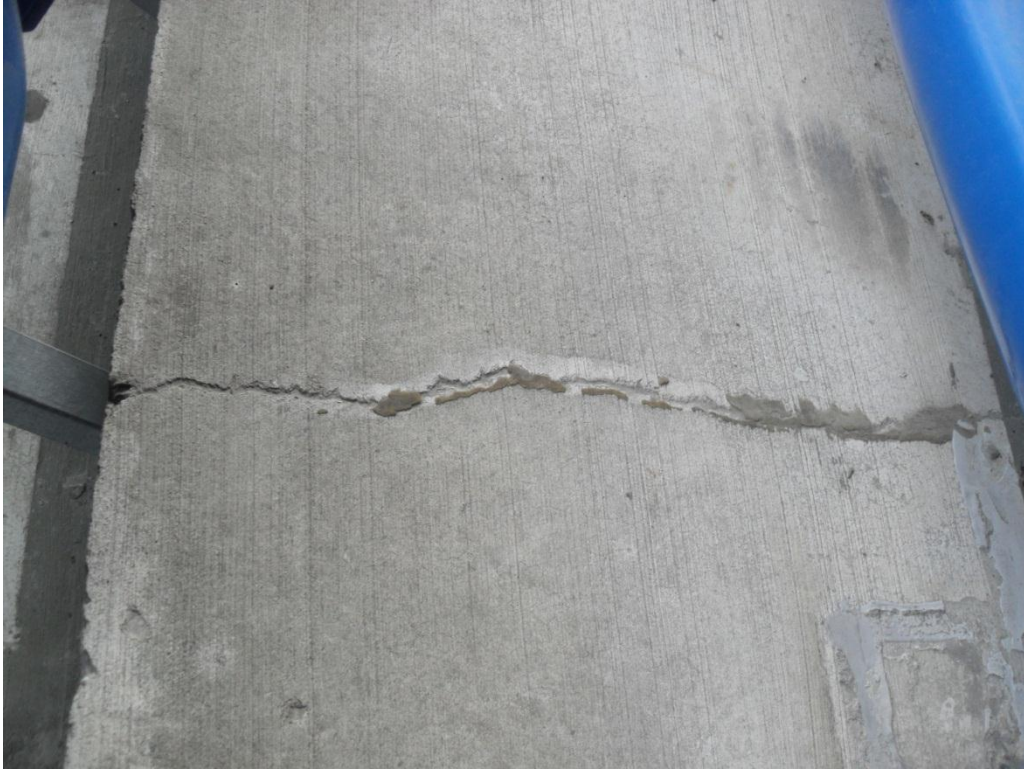
Photograph 25 Cracking in precast concrete seating units.
