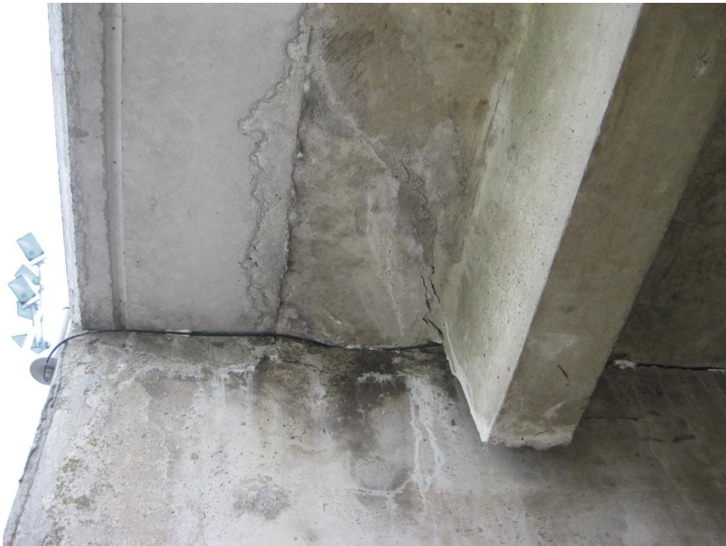
Photograph 22 Cracking in precast double tee flooring unit near supporting beam.
