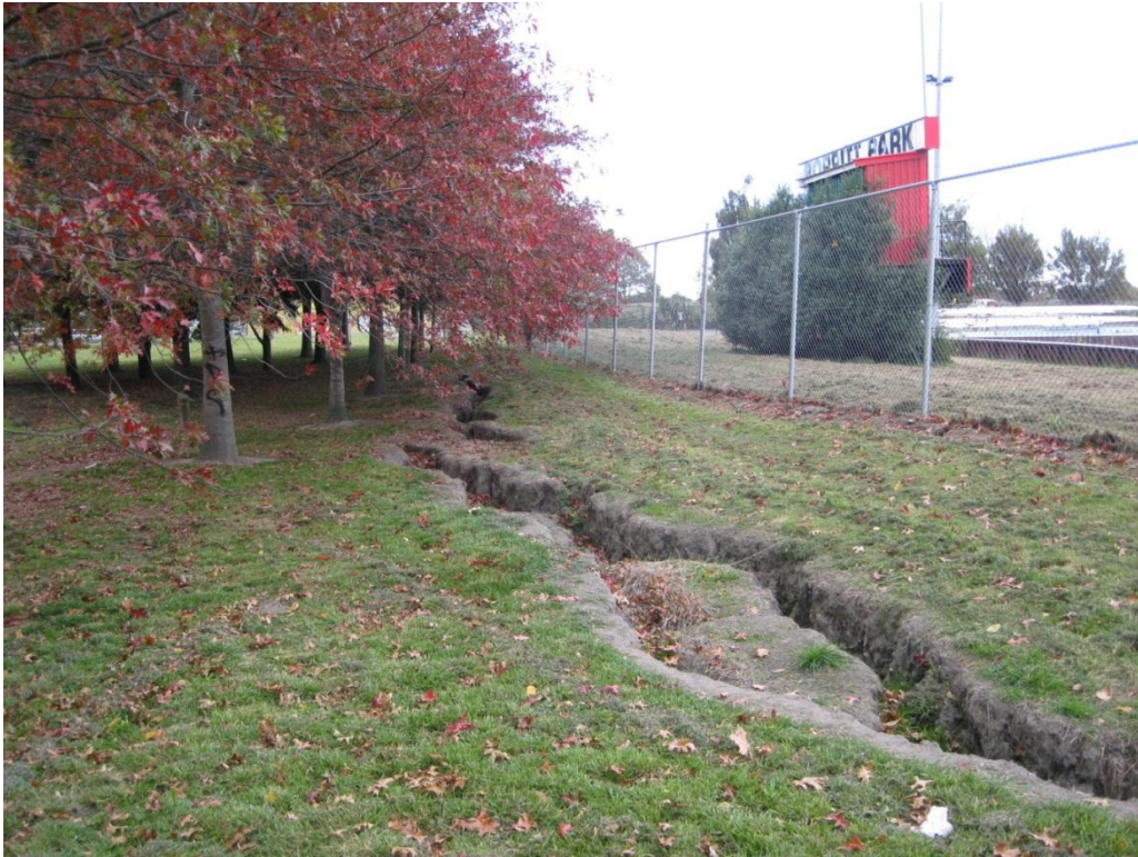
Photograph 1 Ground cracks near the river south of the grandstand.
