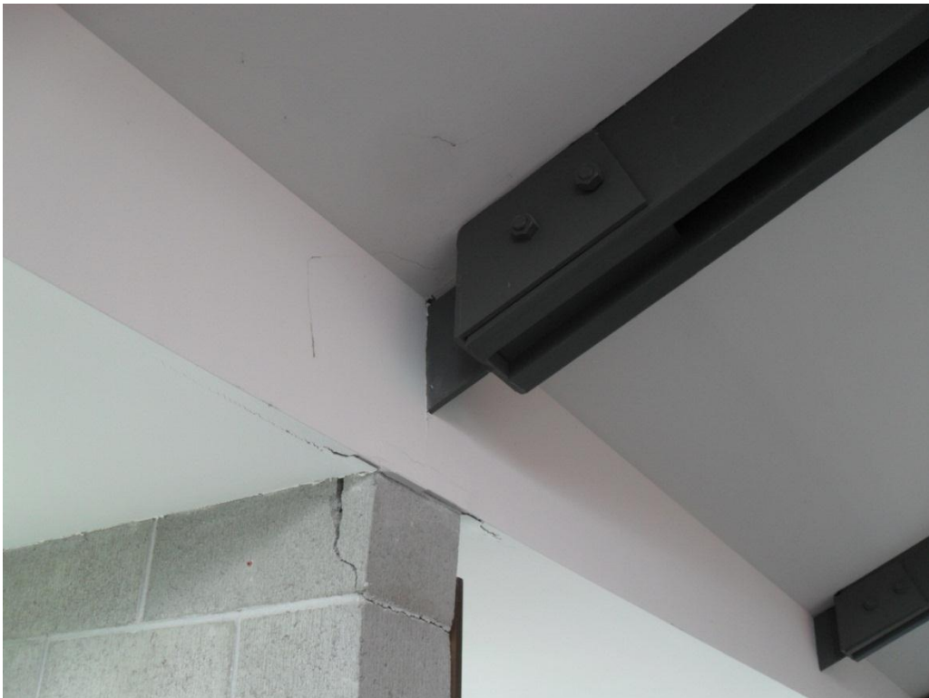
Photograph 20 Damaged connection between a concrete masonry wall and timber rafter.
