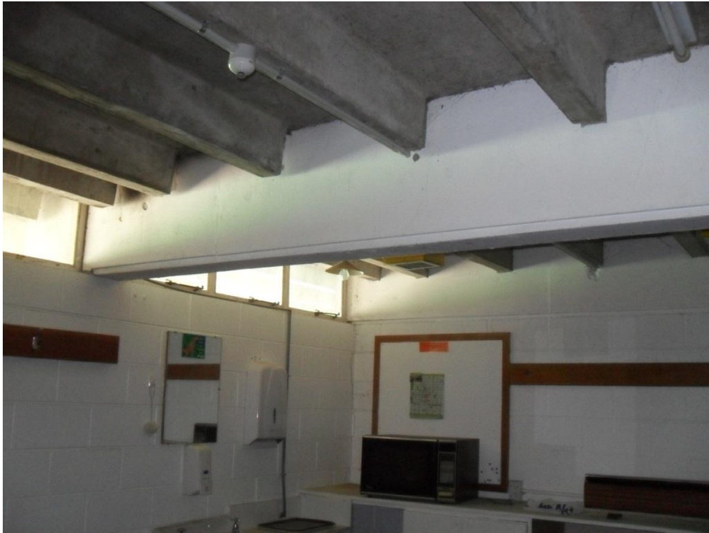
Photograph 17 In-situ beam supporting precast double tee flooring units.
