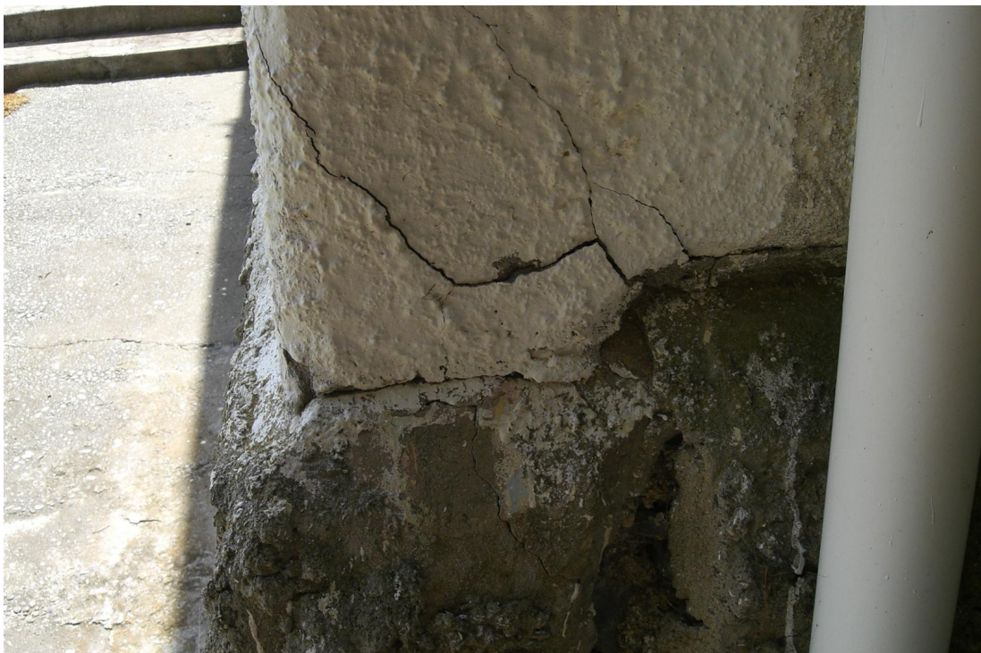
Photo 6: Multiple cracks on the north-west corner.
