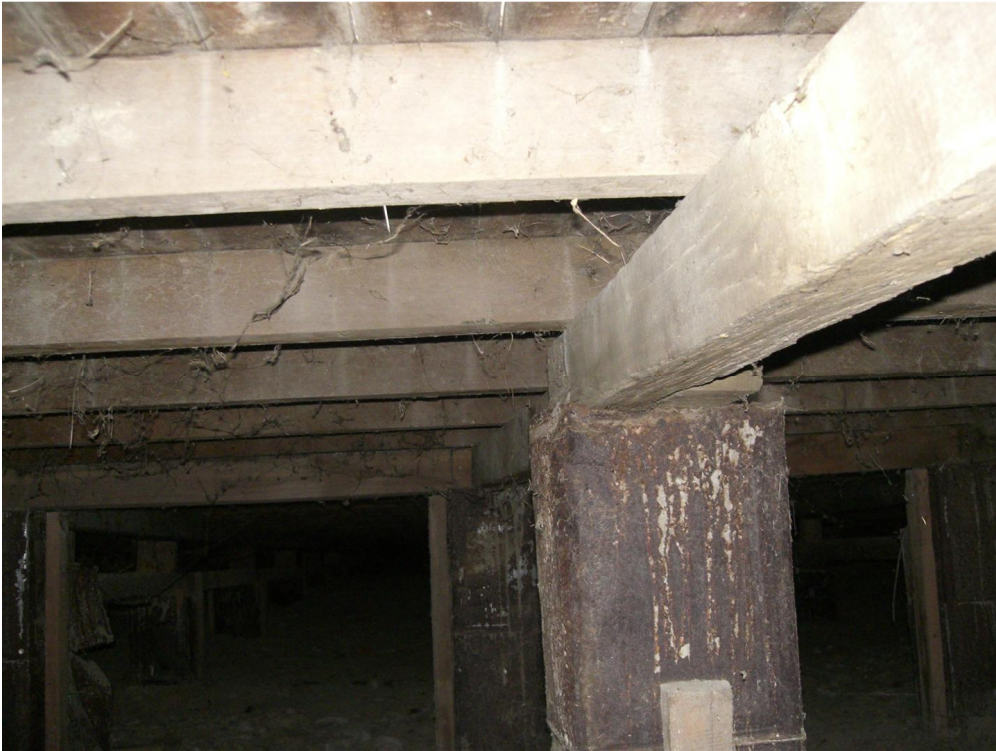
Photo 7: View of the subfloor and foundations
