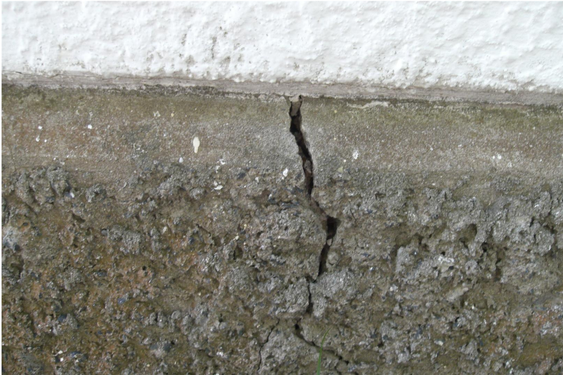
Photo 5: 10mm crack in the concrete perimeter strip footing.
