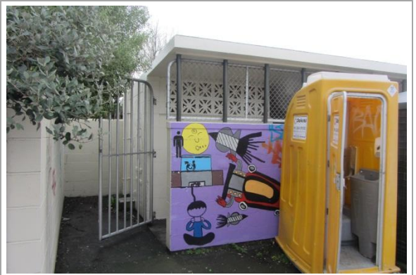
Photo 4: South Elevation – West Wing
