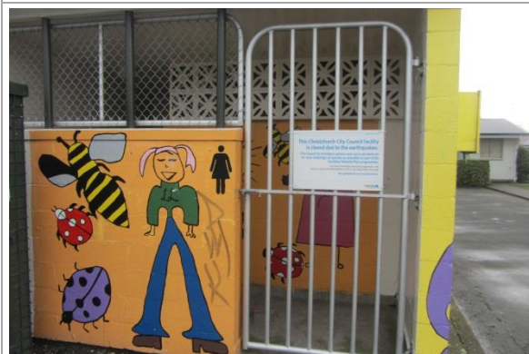
Photo 5: South Elevation – East Wing
