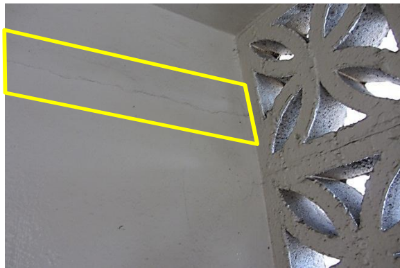
Photo 7: Crack at the top section of the wall adjacent to decorative masonry blocks
