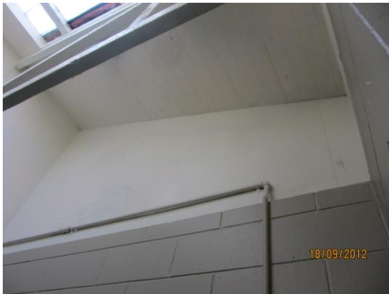
Photo 9: View of roof
