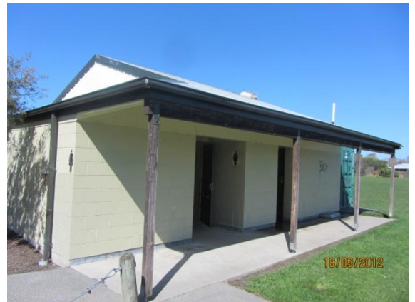
Photo 4: View of womens toilet entrance
