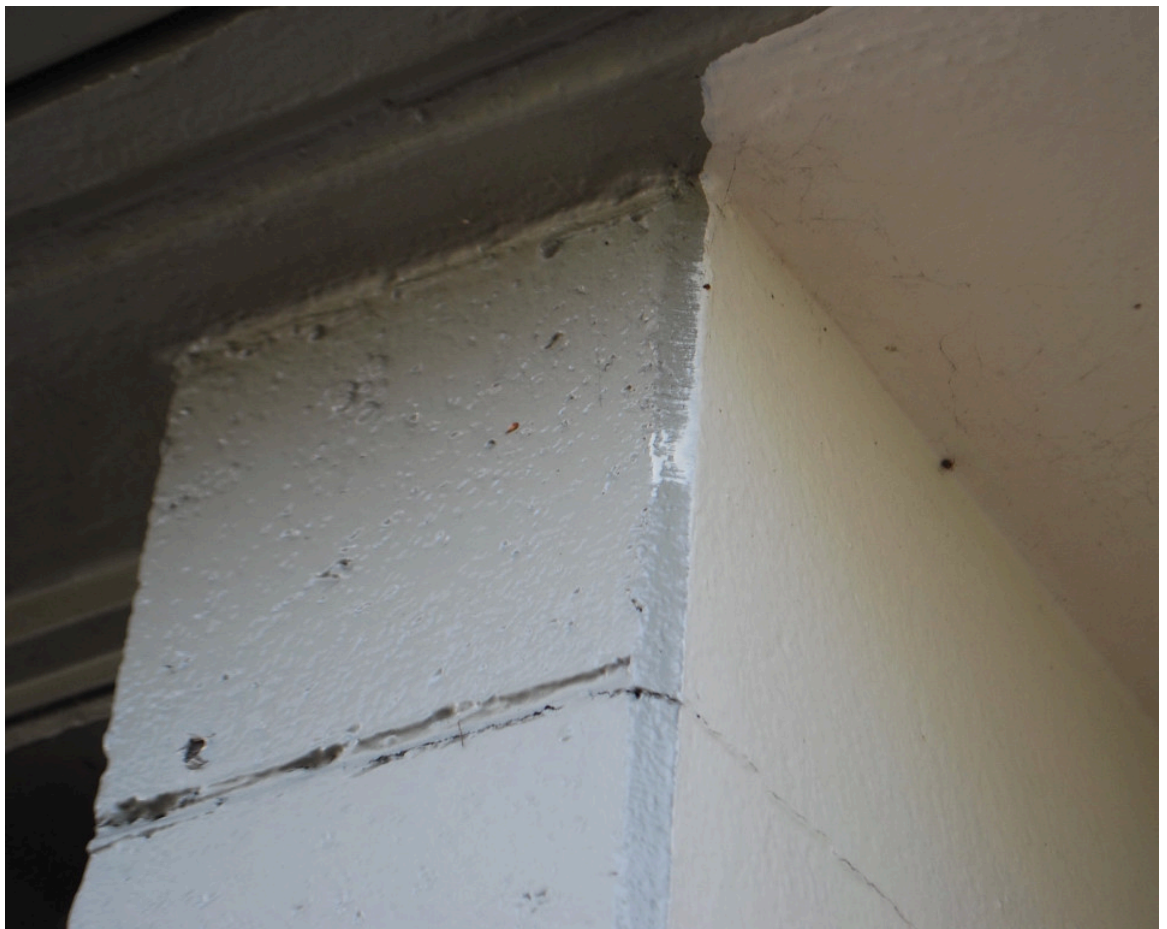
Photograph 6 Detail view showing cracking at wall to roof connection.
