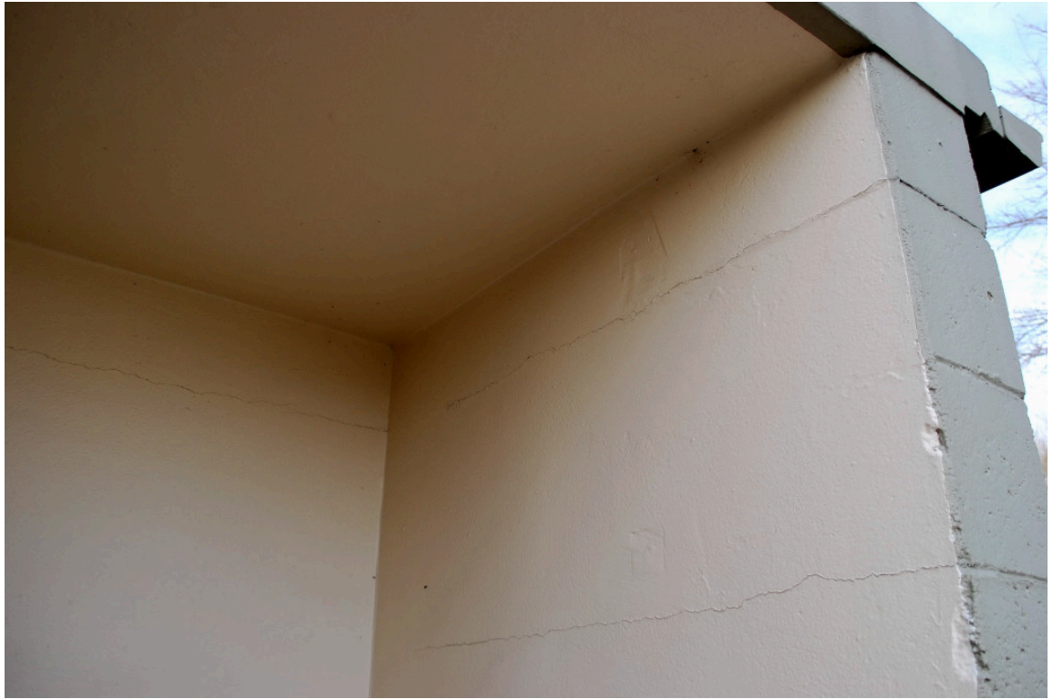
Photograph 7 Horizontal cracking along the top and lower row of blocks.
