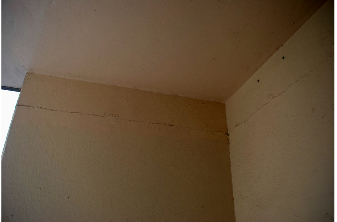
Photograph 5 Horizontal cracking along the top row of blocks.
