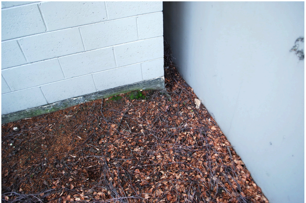
Photograph 8 Foundations on Southeast side of building also showing Separation between neighbouring structure.
