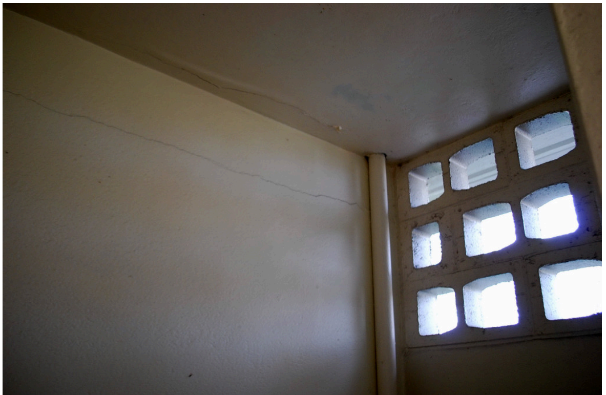
Photograph 10 Horizontal cracking along the top row of blocks.
