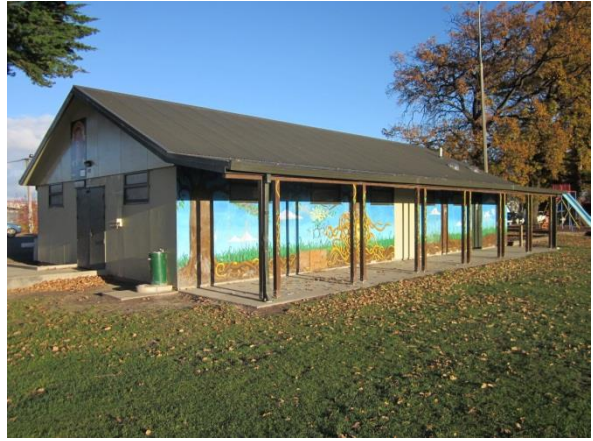
Western elevation of Papanui Domain – Toilets.
