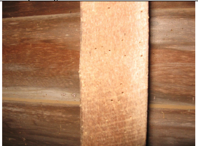
Extensive borer's holes observed throughout building
