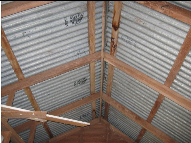
Lightweight corrugated iron roof
