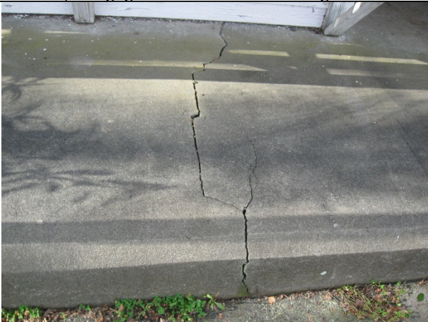
10mm crack in slab – external
