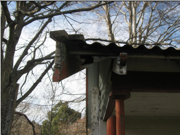
Rotten wood skirting
