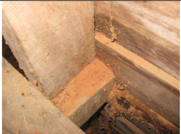
Dust from borer observed
