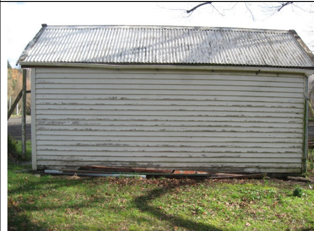
Eastern face of building
