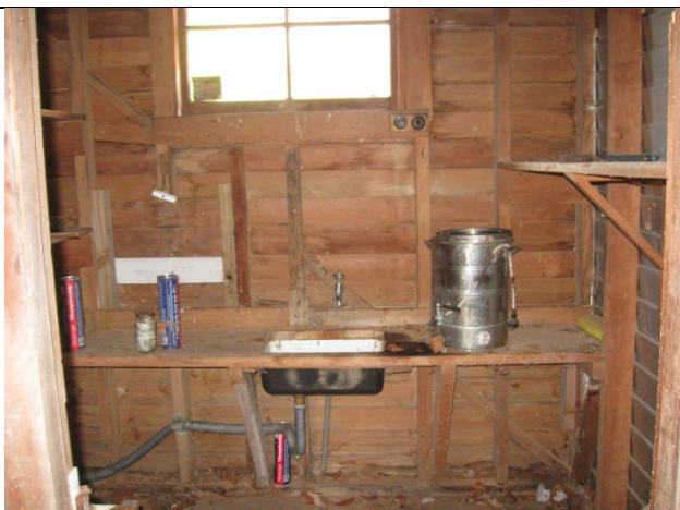
Cut diagonal brace
