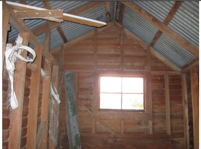
Timber framed. No internal cladding
