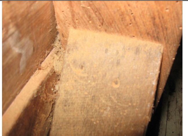
Bracing fixed with skew nail
