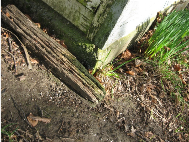
Rotten wood observed
