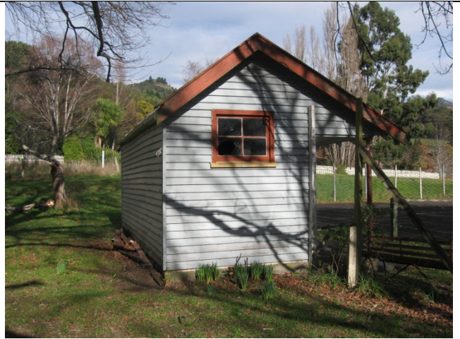
Northern face of building
