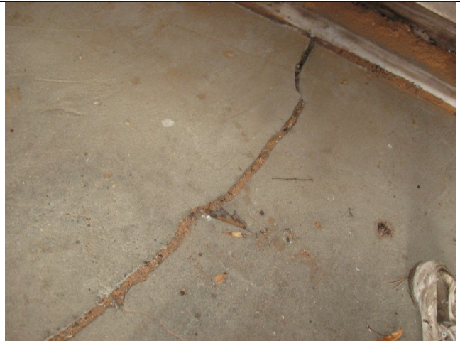
10mm crack observed in slab – internal
