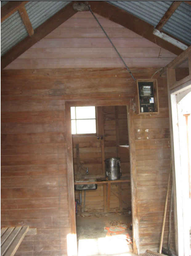
Kitchen/storage area at end of building
