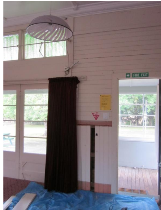
Photo 22: View of north wall in the east corner of building showing location of intrusive investigation, confirming the lack of bracing element behind the tongue and groove lining.
