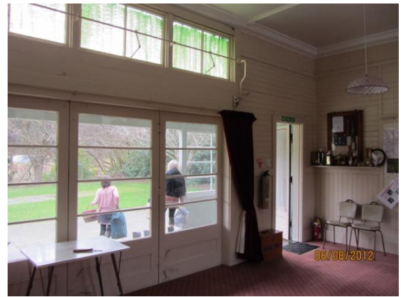
Photo 10: View of the main hall area, north east corner.
