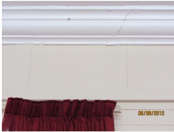
Photo 15: Close up view of photo 14 showing crack in lining and cornice.
