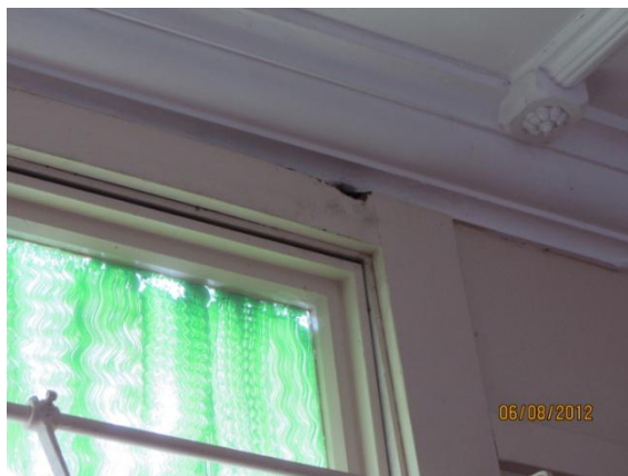
Photo 17: Close up view of photo 16 showing deteriorated timber window frame.
