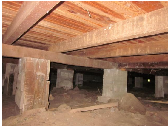
Photo 22: View of foundation in the east part of the building
