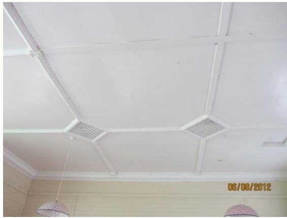
Photo 13: View of the ceiling in main hall area.
