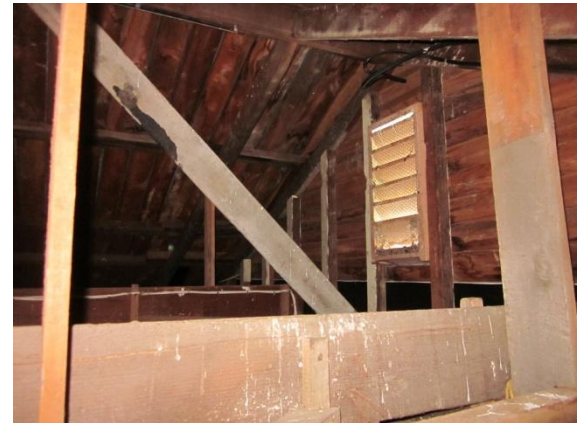
Photo 23: View of roof
