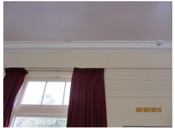
Photo 14: View of the cornice on the south wall
