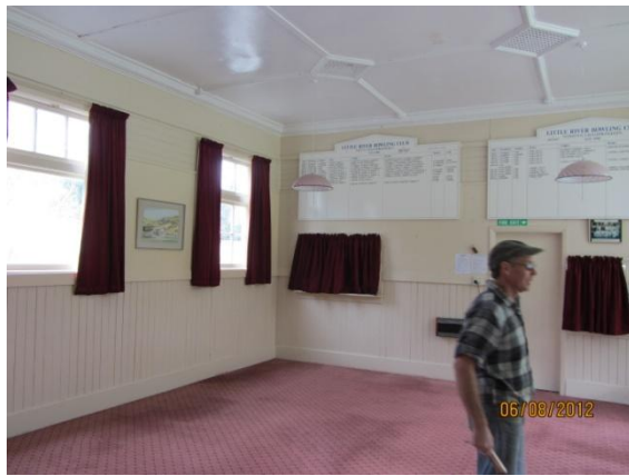
Photo 9: View of the main hall area, south west corner.
