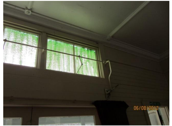
Photo 16: View of north wall and ceiling
