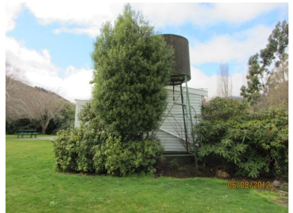
Photo 4: West Elevation (2). Note the leaning watertank.
