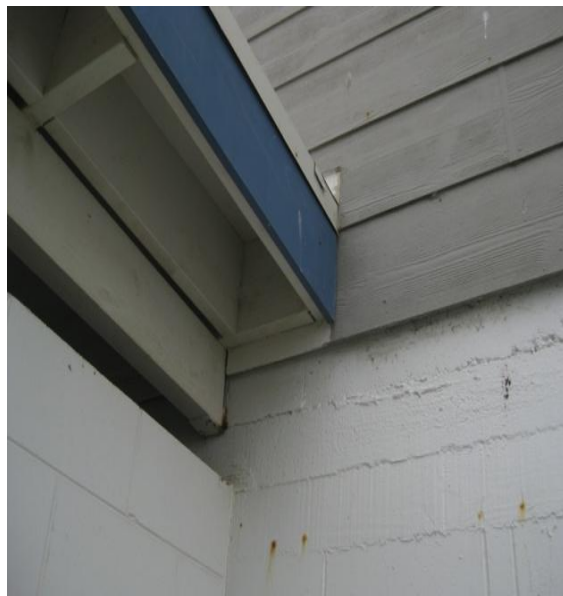
Photo 15: Internal wall between toilets and changing room connecting to share wall between toilet block and North Beach Surf Club.
