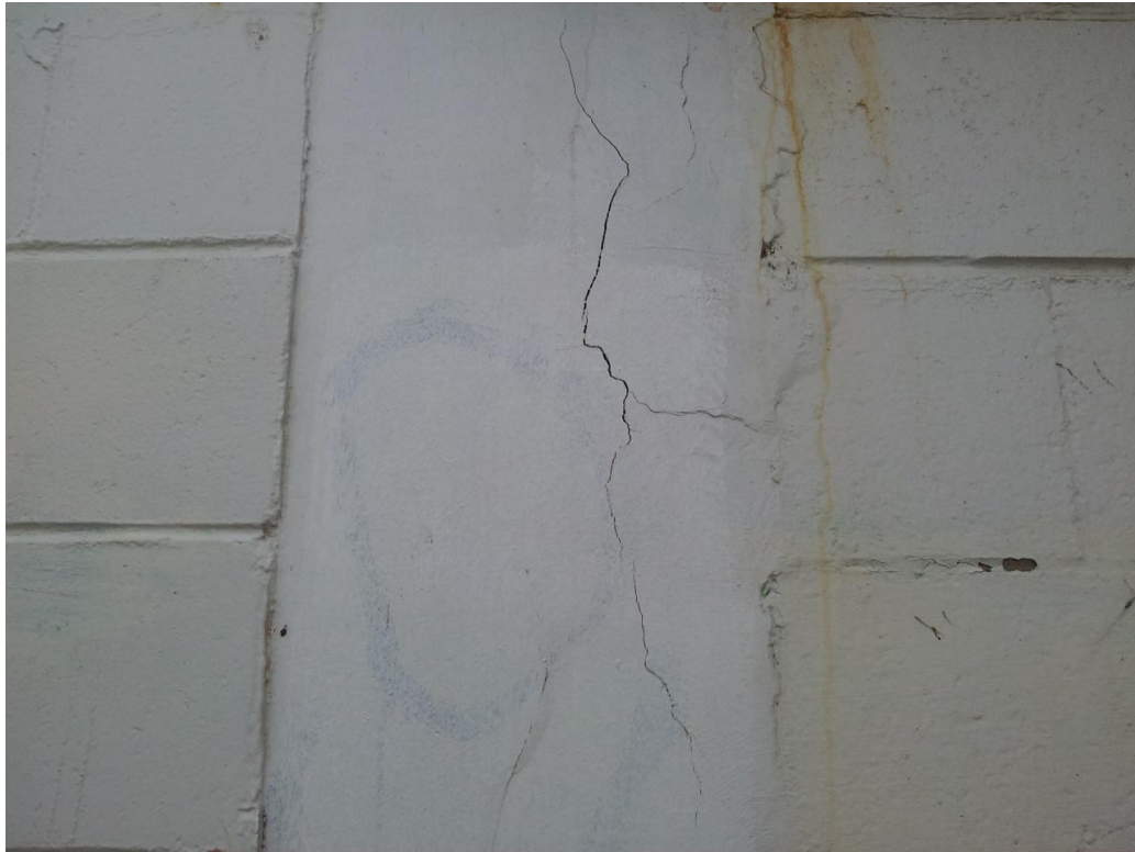
■ Figure 9 - Observed cracks in the wall
