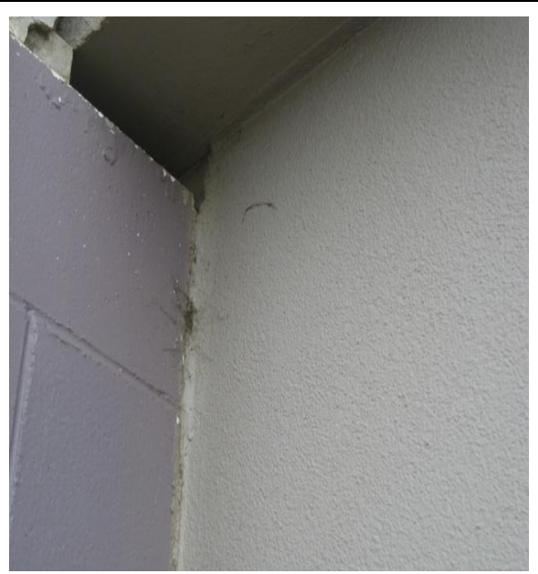
Photo 22: Connection between the masonry wall of the toilet block and the Surf Club on the southern wall.
