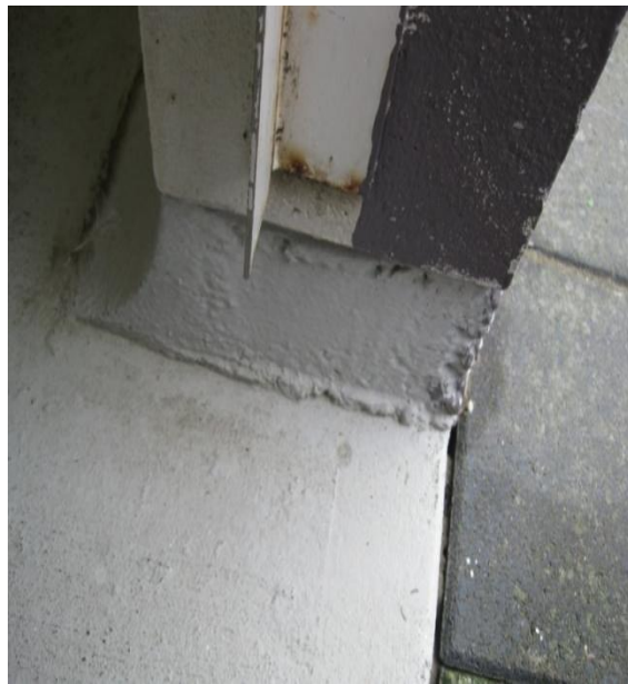
Photo 9: Footing of masonry wall and concrete ground slab.
