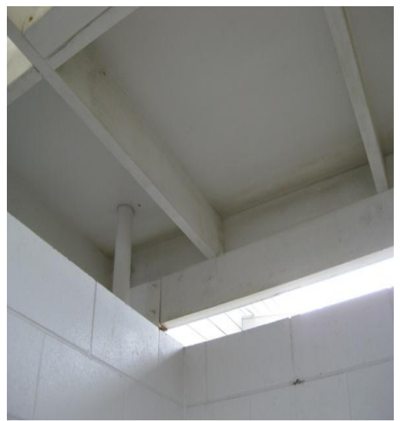
Photo 6: Timber-framed roof inside toilet block.
