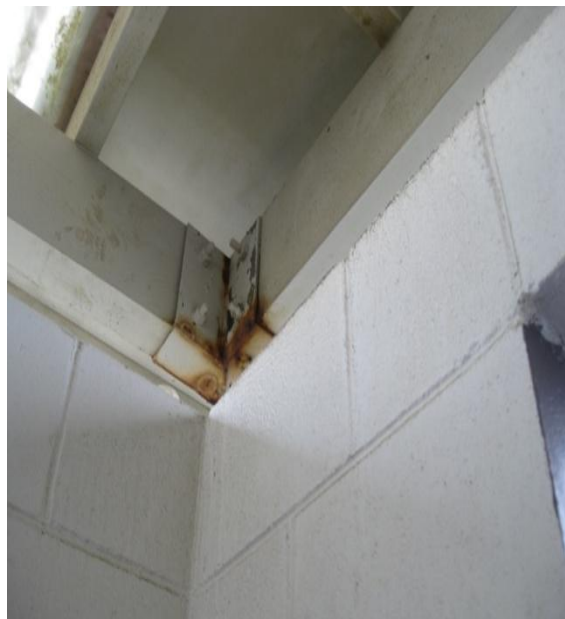
Photo 7: Rusting of timber-masonry steel connection (typical).
