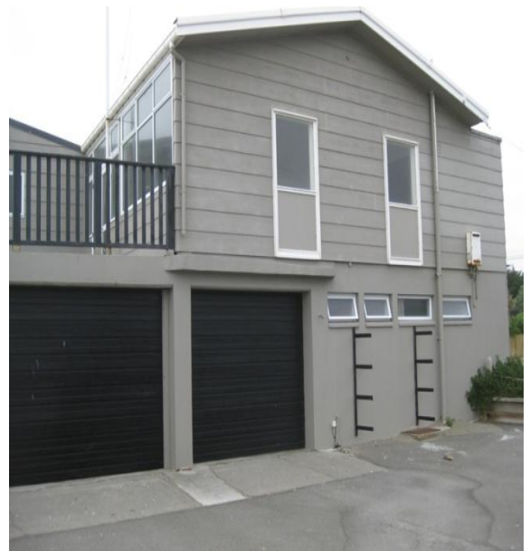
Photo 28: North elevation of Surf Club.
