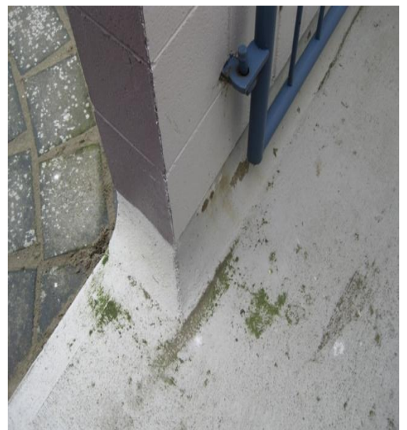
Photo 12: Footing and gate connection on masonry wall and concrete ground slab.
