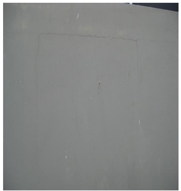
Photo 26: Cracking at assumed plasterboard joints on the first-floor east wall external cladding (typical).
