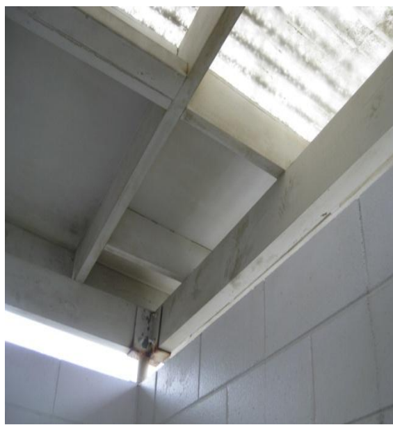
Photo 5: Timber-framed roof inside toilet block.
