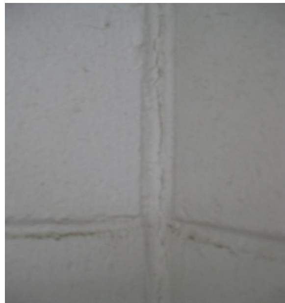
Photo 8: Cracking along mortar joint between internal and external wall.
