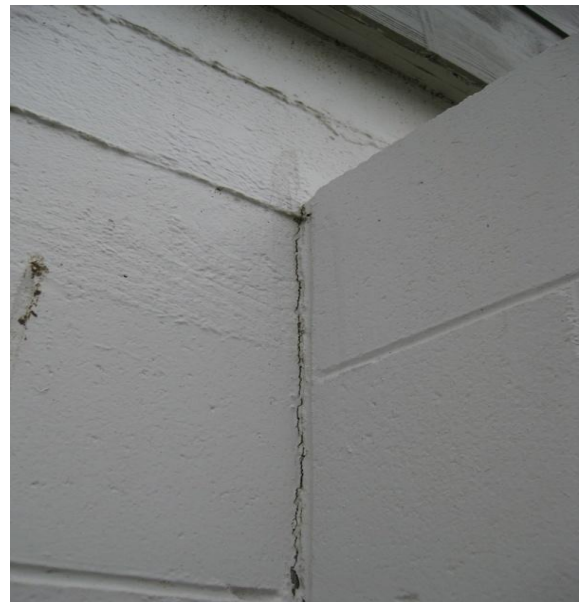
Photo 18: Gap opening up between shared wall and internal masonry wall along the mortar joint.
