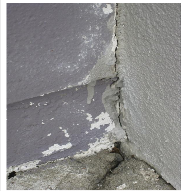
Photo 23: Gap opening up between external changing room masonry wall and Surf Club southern wall.
