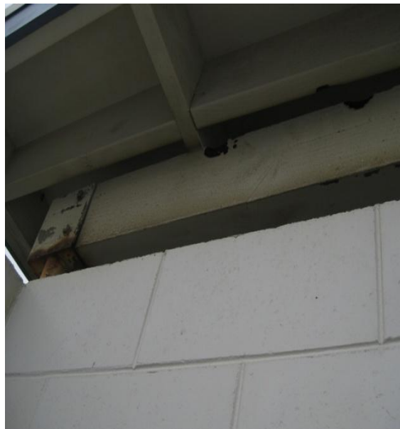
Photo 13: Paint removal on timber edge roof beam and rusting of timber-masonry steel connection.
