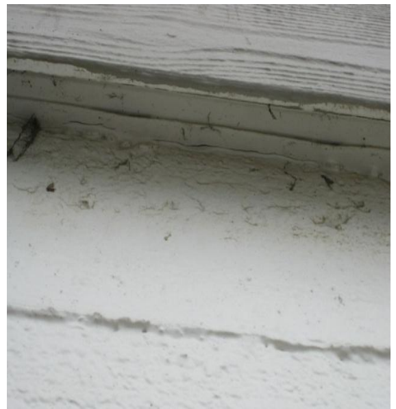
Photo 16: Masonry and weatherboard interface on shared south wall.
