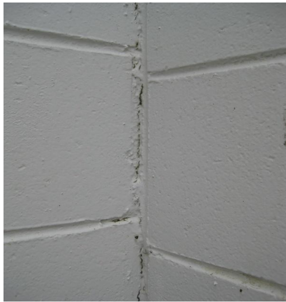
Photo 17: Gap opening up between shared wall and internal masonry wall along the mortar joint.
