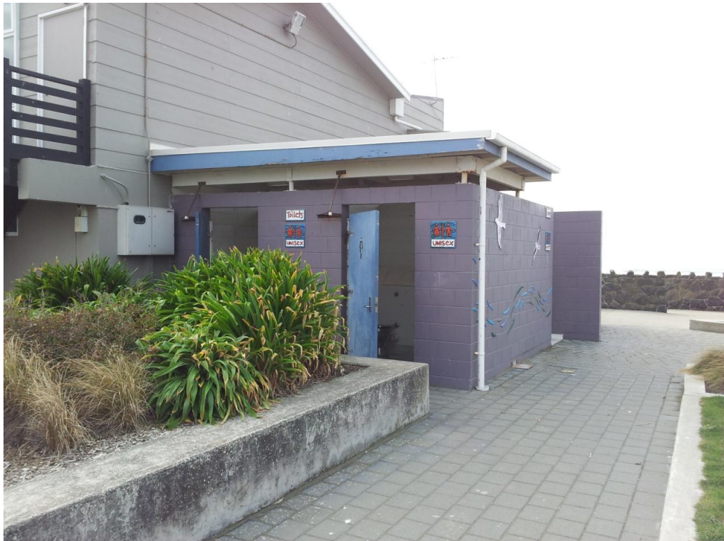
■ Figure 7 - External view of toilets (west elevation)
