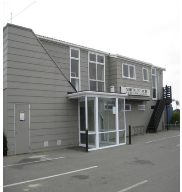
Photo 30: West elevation of Surf Club.
