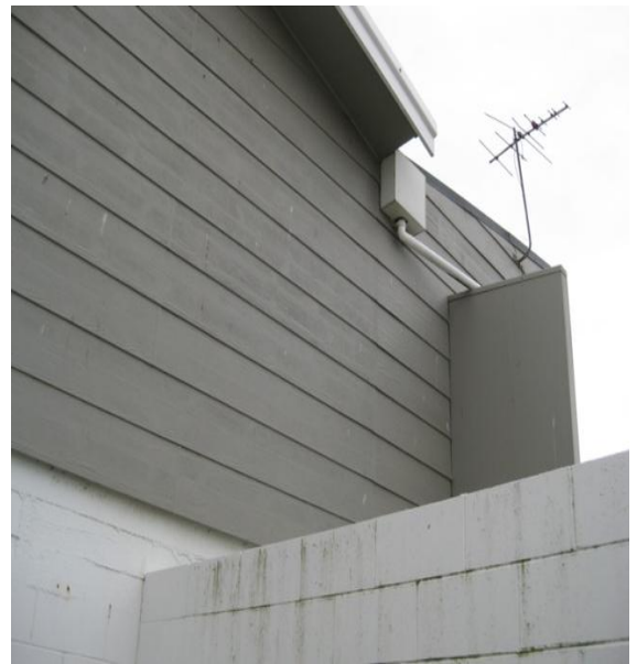
Photo 14: Internal wall between changing rooms connecting to shared wall between toilet block and North Beach Surf Club.
