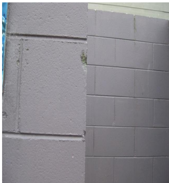
Photo 11: Existing impact damage to masonry on changing room entrance.
