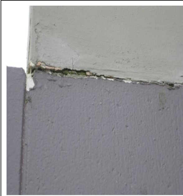
Photo 21: Gap opening up between masonry wall and wall extension (material unknown).
