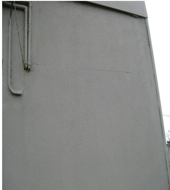
Photo 29: Cracking at assumed plasterboard joints on the first-floor east wall external cladding (typical).
