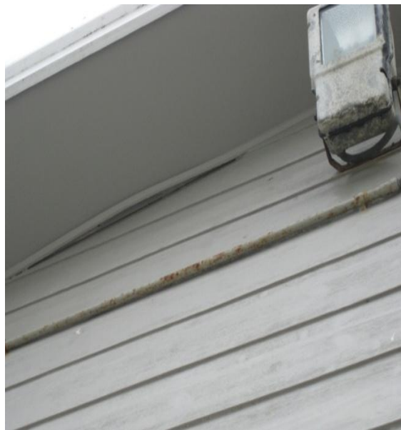
Photo 19: Buckling of soffit cladding element on south wall.
