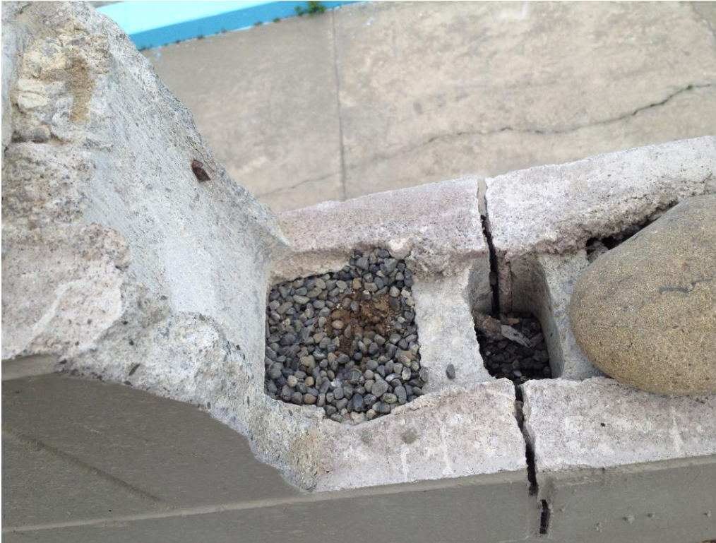
Photo 7: Concrete masonry fence to the north of the pool.
