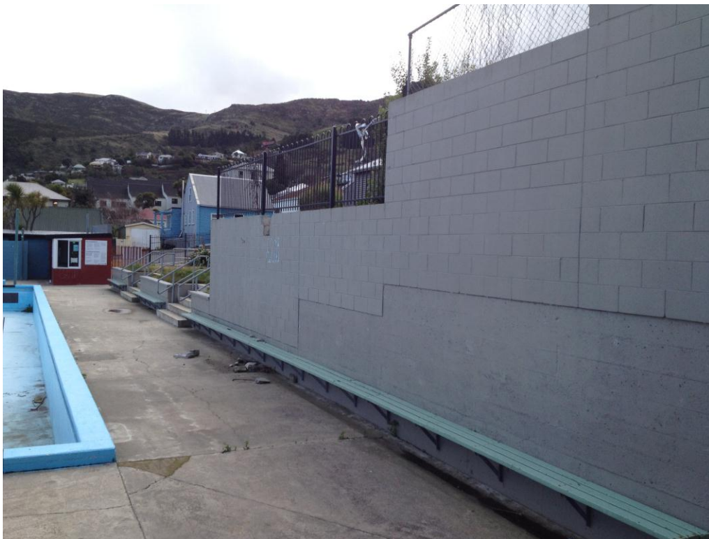
Photo 6: Concrete retaining wall and concrete masonry block fence to the north of the pool (view from south-east).
