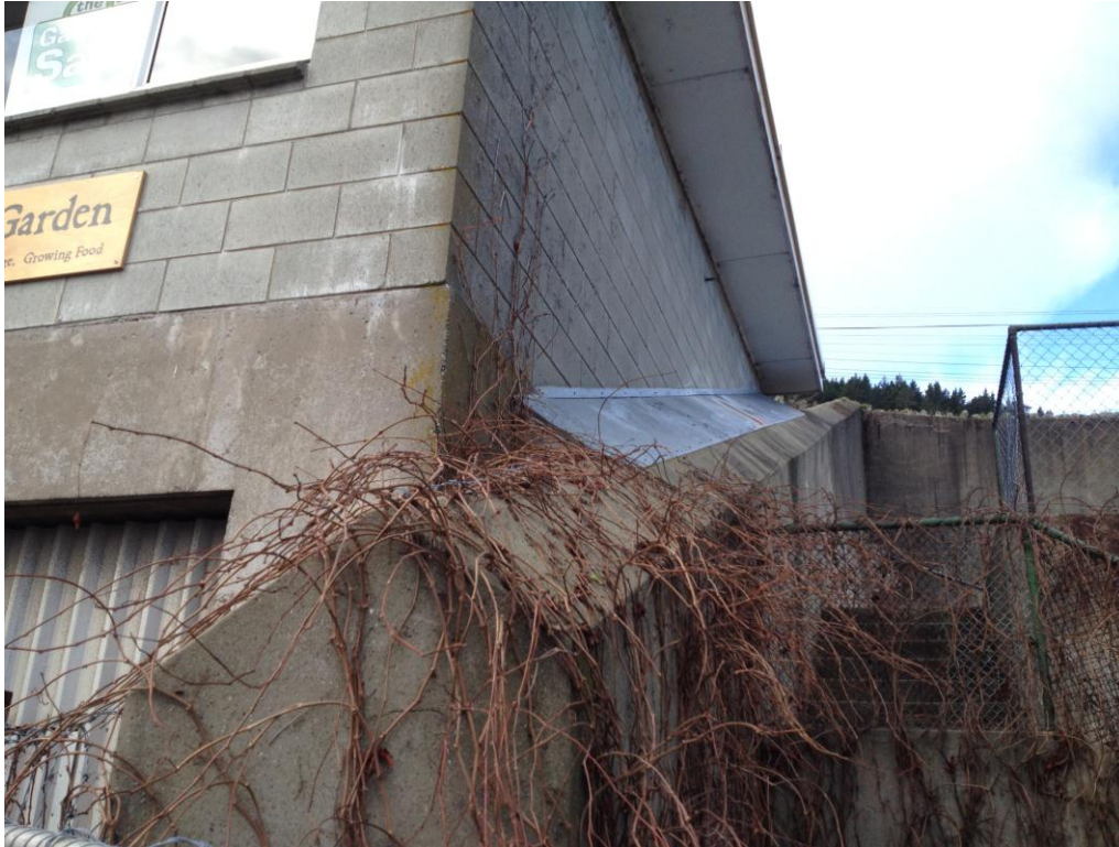
Photo 3: Retaining wall with pounding potential to the south of the Nursery Building.
