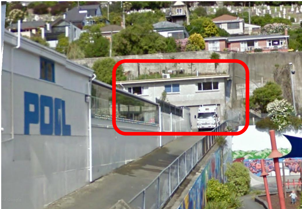
Photo 4: External view from the west, with concrete retaining walls to east and south shown. Source: Google Maps.
