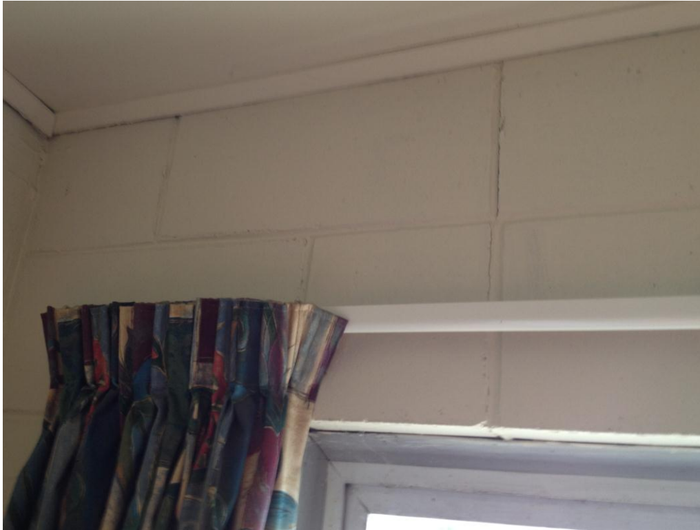
Photo 5: Internal concrete masonry block wall.
