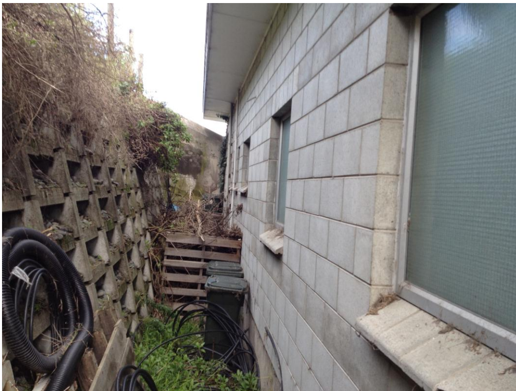
Photo 2: Crib Wall (left) to the east of Nursery Building (note: this is at first floor level).
