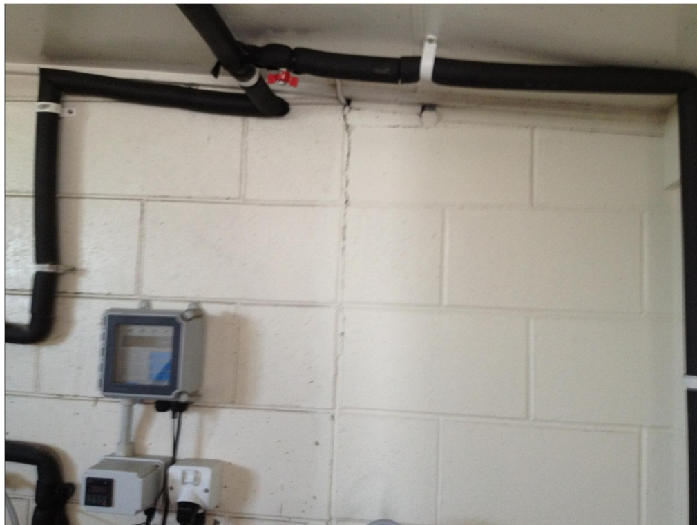
Photo 6: Internal concrete masonry block wall of Plant Room. Damage Description: Concrete masonry and mortar cracking.
