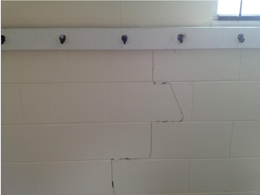
Photo 9: Internal concrete masonry wall of Men's Change Room. Damage Description: Concrete masonry and mortar cracking.
