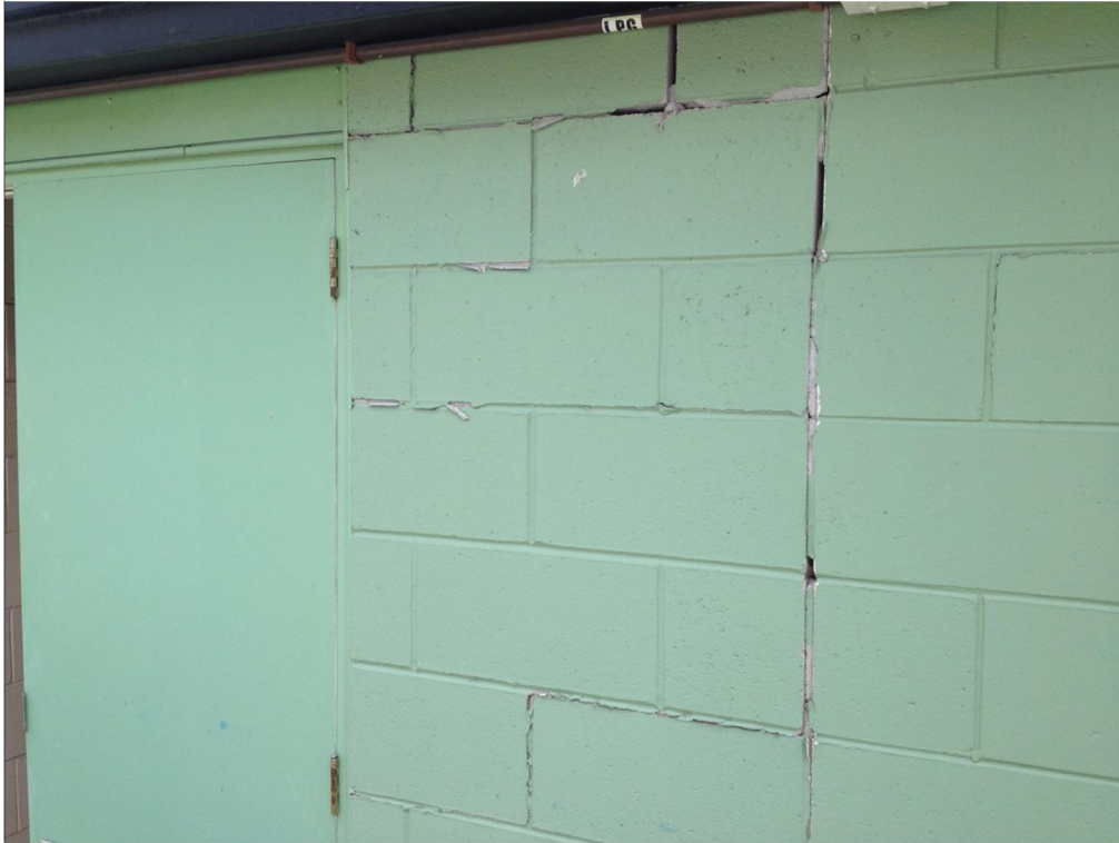
Photo 7: External concrete masonry wall of Plant Room.
