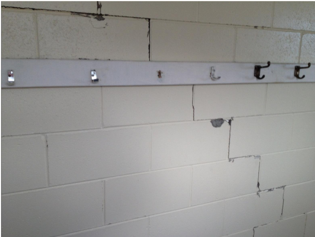
Photo 8: Internal concrete masonry wall in Men's Change Room.
