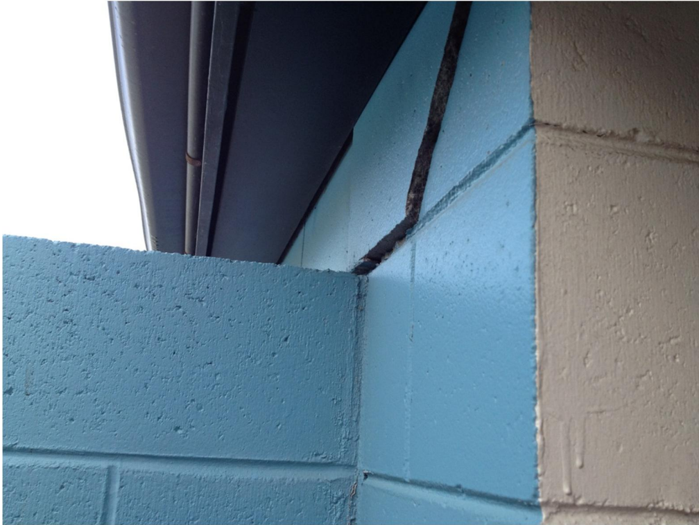
Photo 11: External concrete masonry block wall outside of Men's Change Room. Damage Description: Cracked and dislodged concrete masonry unit.
