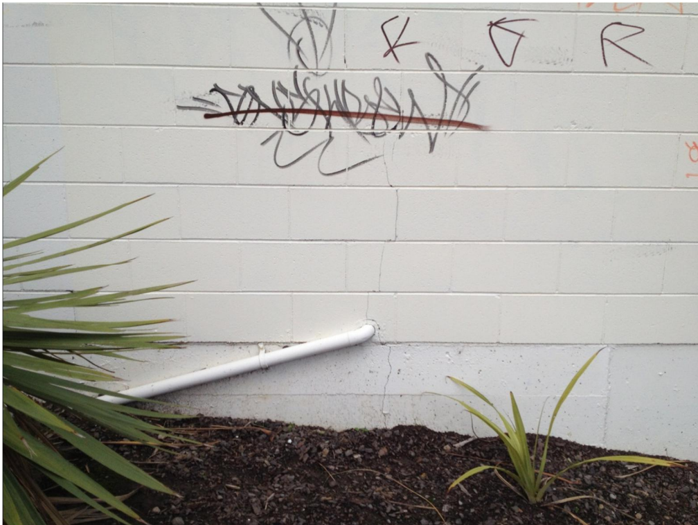
Photo 12: Concrete masonry block wall and concrete retaining wall on western side. Damage Description: Cracking in concrete masonry and mortar, and concrete retaining wall.
