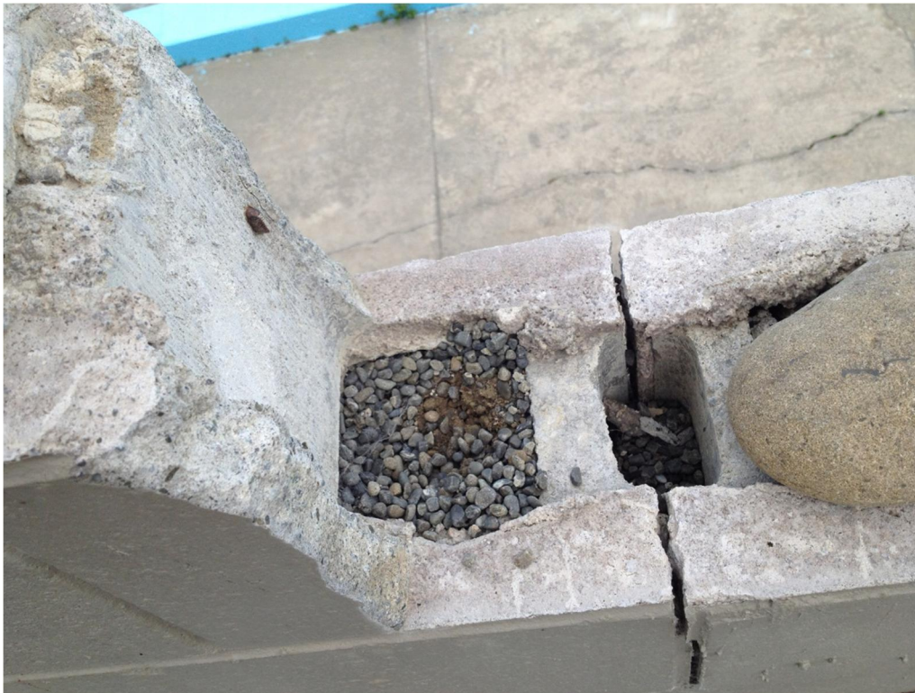
Photo 16: Concrete masonry fence to the north of the pool.
