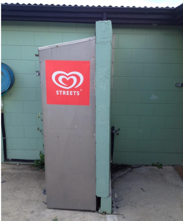
Photo 14: Privacy entrance wall to Disabled Bathroom (view from north).
