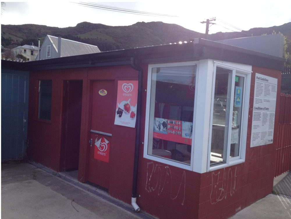
Photo 2: Office Building (Wing of Men's Change Room Block).
