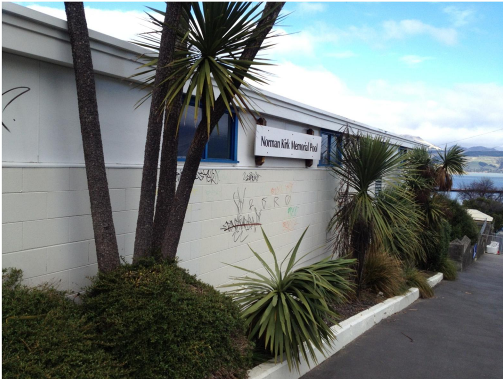
Photo 4: External view of Men's Change Room (view from west).
