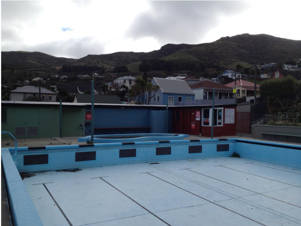
Photo 1: Men's Change Room Block. The Plant Room is on the left (green), the Men's Change Room is in the centre (blue) and the Office is on the right (red).
