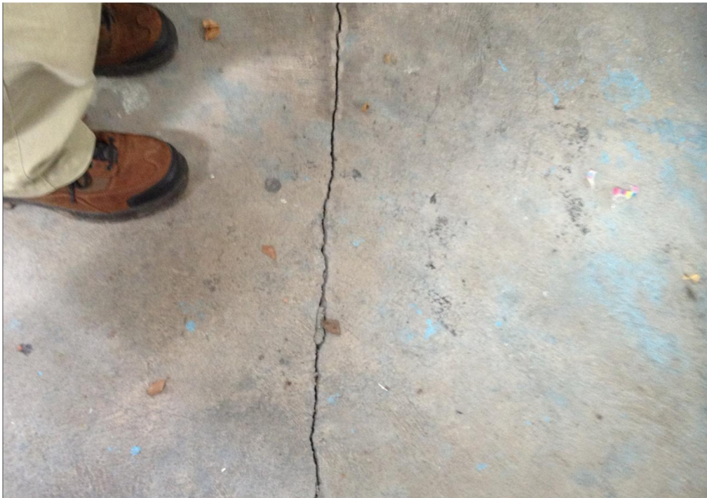
Photo 10: Ground slab in Men's Change Room. Damage Description: Cracking to ground slab.
