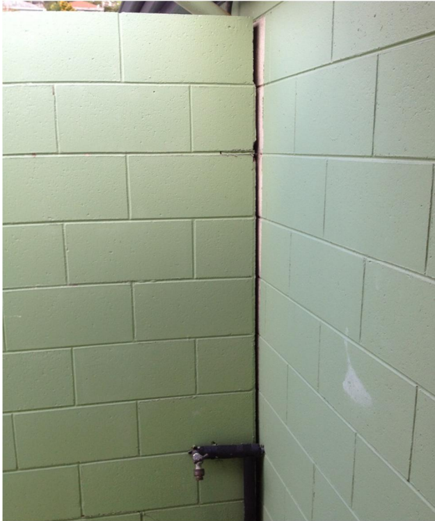
Photo 13: Privacy entrance wall to Disabled Bathroom (view from east).
