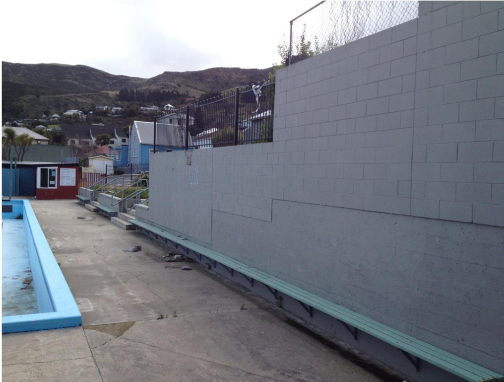
Photo 15: Concrete retaining wall and concrete masonry block fence to the north of the pool (view from south-east).
