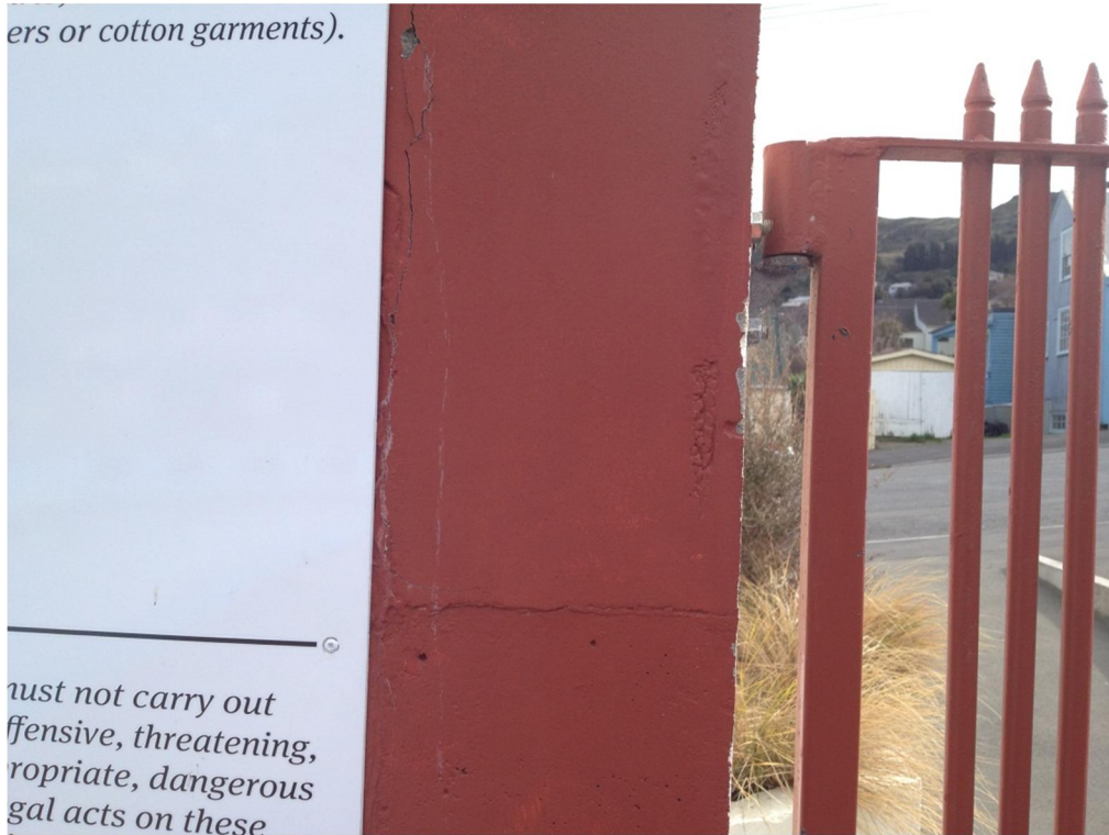
Photo 5: External masonry/rendering at office building. Damage Description: Cracking/spalling to external rendering.
