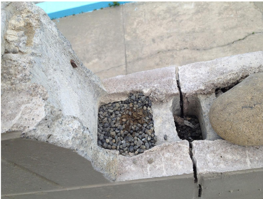
Photo 8: Concrete masonry fence to the north of the pool.
