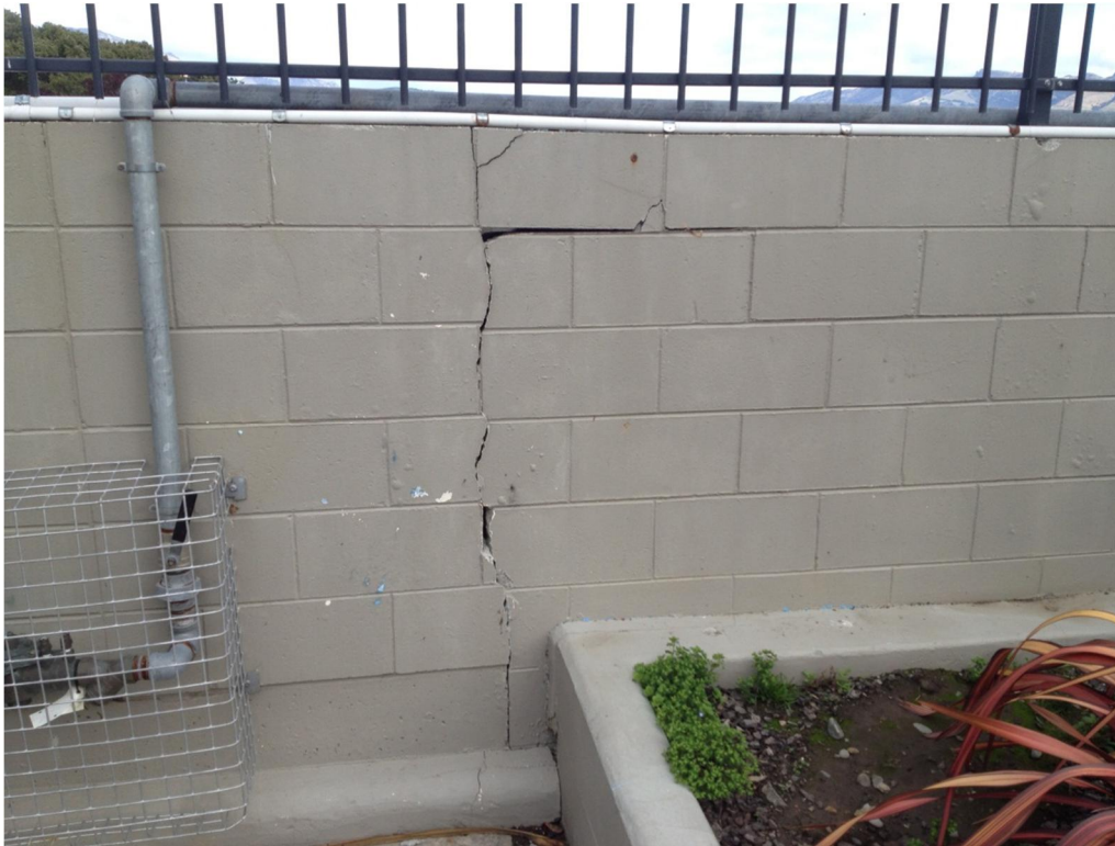
Photo 5: Adjacent concrete masonry block wall along driveway between Main Plant Room and Lean-to Shelter. The Main Plant Room is immediately to the left of this photo (view from north). Damage Description: Cracking and differential settlement of concrete masonry block wall.
