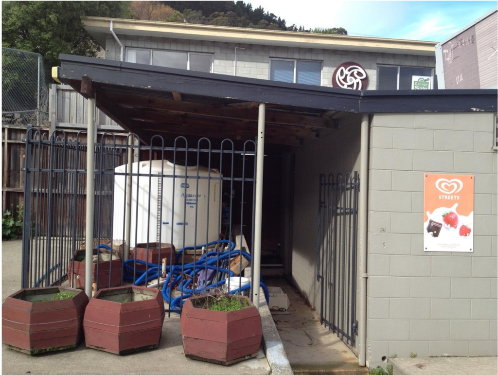
Photo 2: External view of Main Plant Room.
