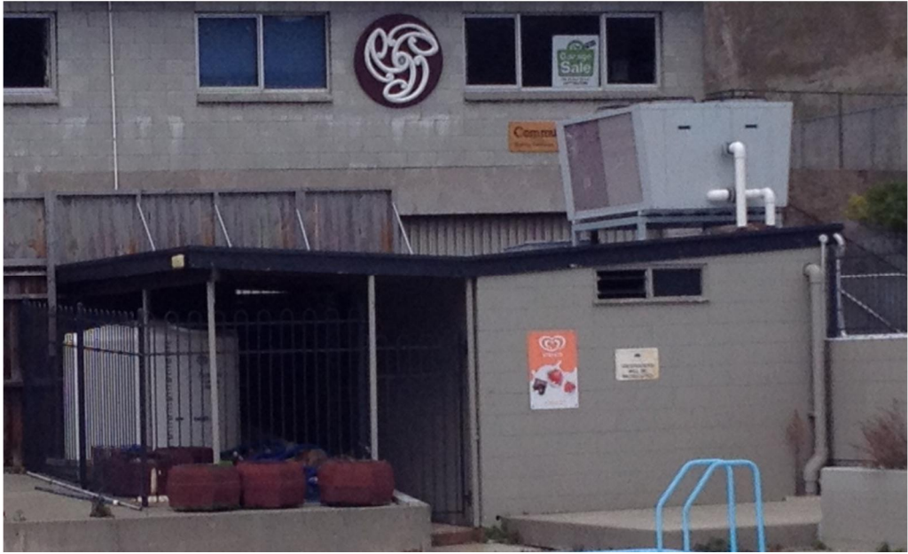
Photo 1: External view of Main Plant Room.
