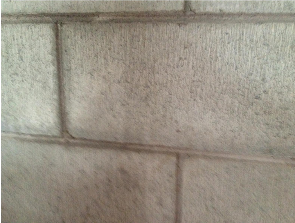
Photo 3: Internal concrete masonry block work.
