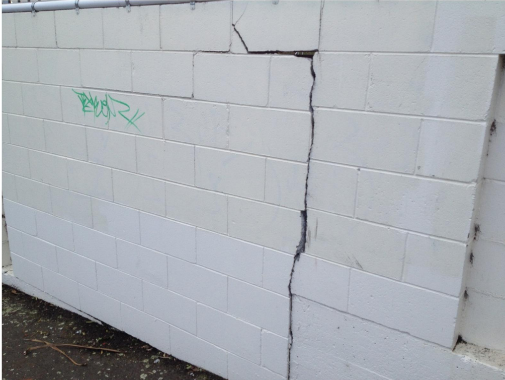
Photo 4: Adjacent concrete masonry block wall along driveway between Main Plant Room and Lean-to Shelter. The Main Plant Room is immediately to the right of this photo (view from south).
