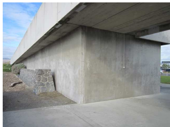
Northern eastern elevation of the New Brighton Pier - Toilets.
