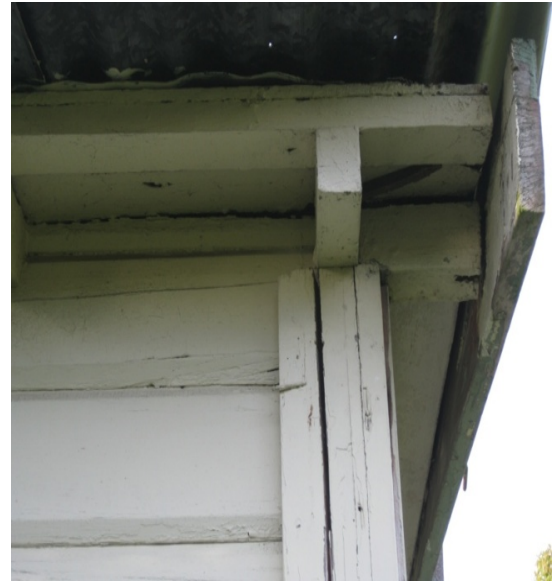
Photo 28: Longitudinal crack along timber element on southwest corner of building.
