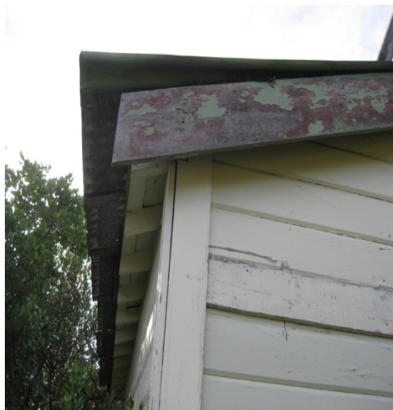
Photo 29: West soffit with corrugated metal roof sheeting above 80x50mm timber rafters at 450mm centres.
