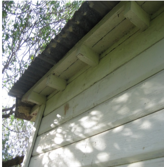
Photo 19: West soffit with timber elements and corrugated metal roof sheeting above.
