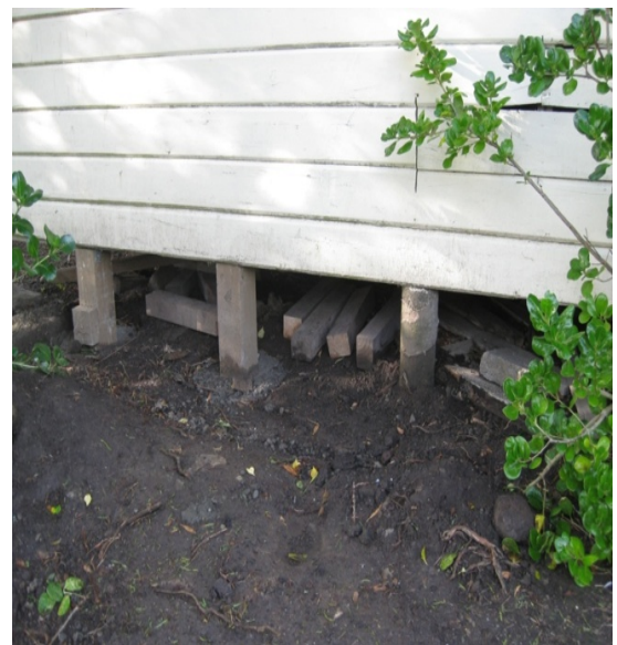
Photo 22: Two timber piles with a concrete pile on their right on the west side of the building are shown.
