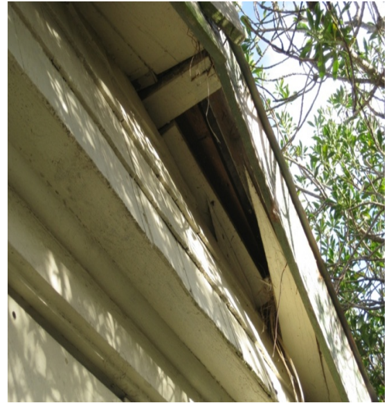
Photo 6: Missing timber elements on north soffit.
