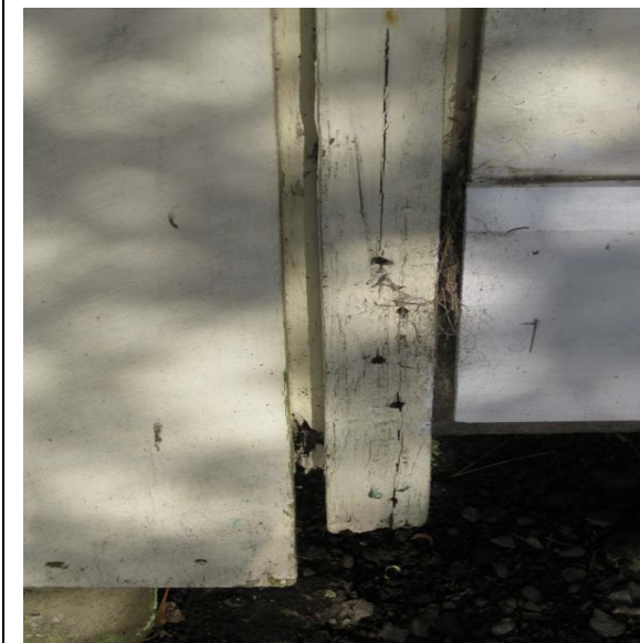
Photo 7: Longitudinal cracks in timber element on north wall.
