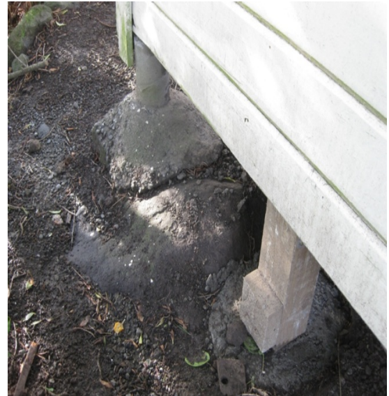
Photo 20: Northwest concrete pile and timber pile shown.
