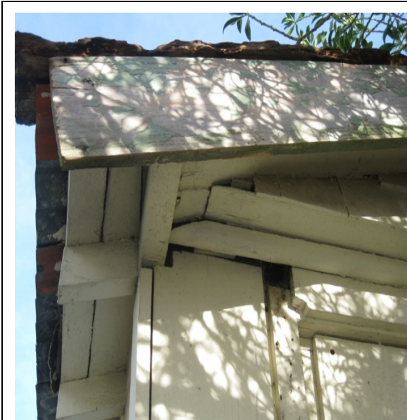
Photo 5: Gaps opening up between timber elements on north soffit.
