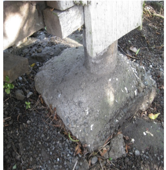
Photo 14: Concrete pile on northwest corner of building with 450mm square concrete footing exposed.
