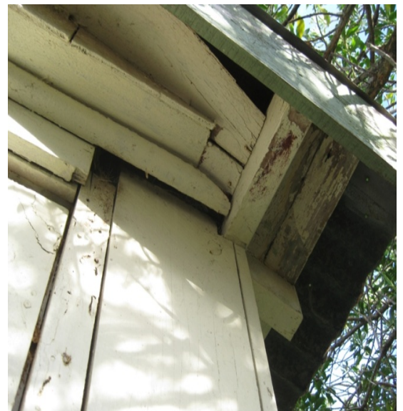
Photo 18: Gaps opening up between timber elements on north soffit.
