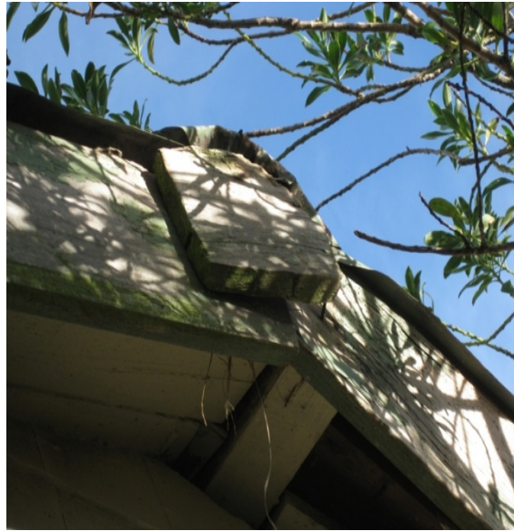
Photo 9: Loose timber element on north side of the building at roof level.
