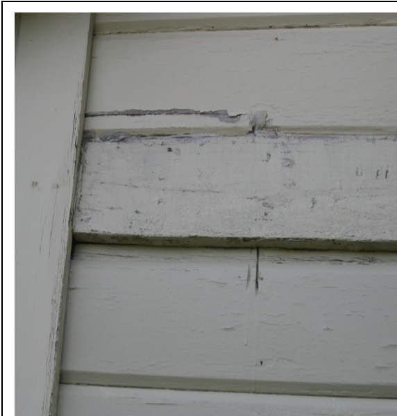
Photo 31: Longitudinal crack in timber weatherboard on south wall.
