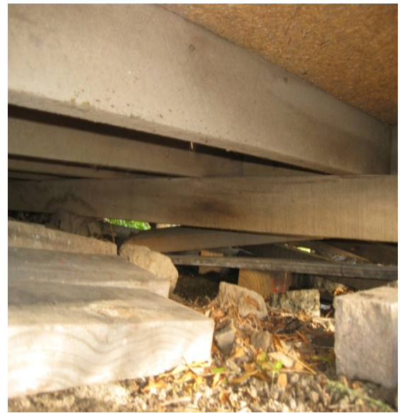
Photo 12: 150x50mm timber joists at 475mm centres spanning across the building with bearer at mid-span.
