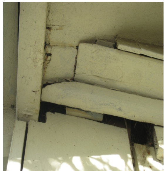
Photo 8: Gaps opening up between timber elements on north soffit.
