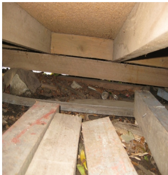
Photo 21: Timber joists on bearer at mid-span.
