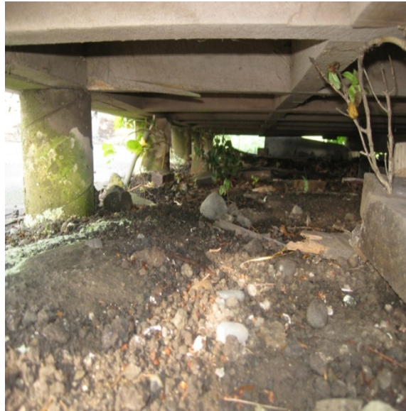
Photo 13: Concrete piles on east perimeter of building, with joists and 150x50mm nogs shown.
