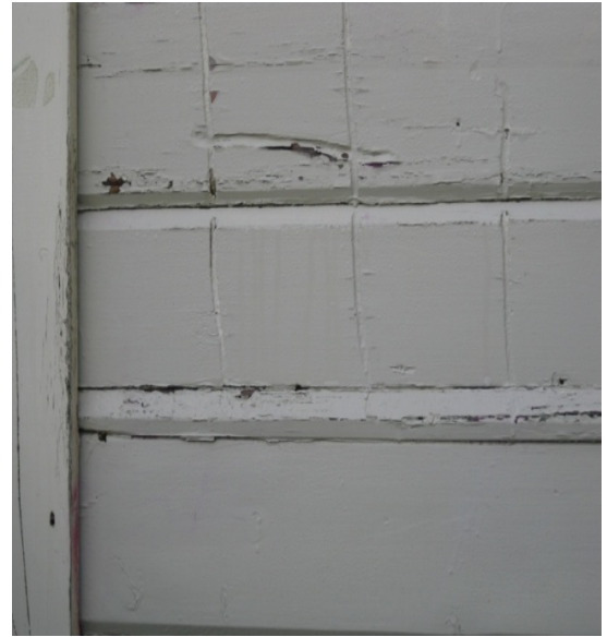
Photo 32: Longitudinal crack in timber weatherboard on south wall.
