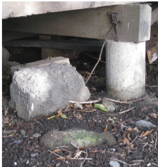
Photo 11: 150x50mm timber bearer spanning along the building at mid-span resting on concrete pile.
