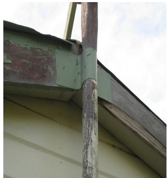
Photo 30: Metal plate support for timber post on south side of building.
