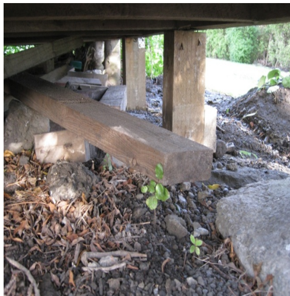
Photo 17: Two 130mm square timber piles in concrete footings replacing concrete piles on the west side.
