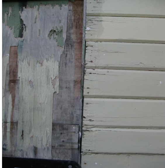
Photo 35: Longitudinal cracking in timber weatherboards at connections on south wall of building by entrance.
