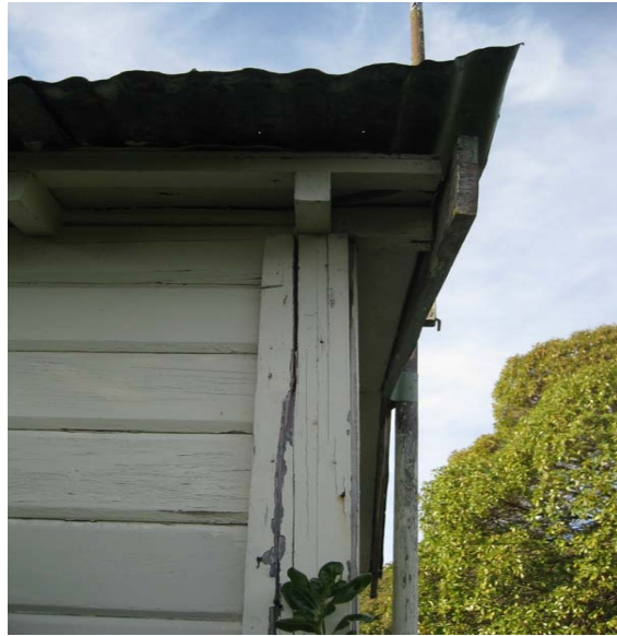
Photo 27: Longitudinal crack along timber element on southwest corner of building.
