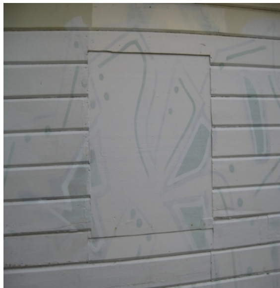
Photo 37: Covered opening on east wall.
