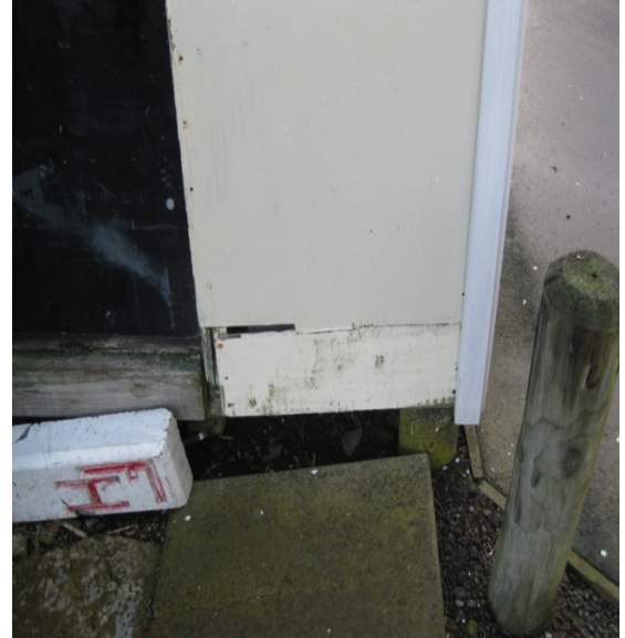
Photo 36: Plasterboard cladding on south wall, east of the entrance.
