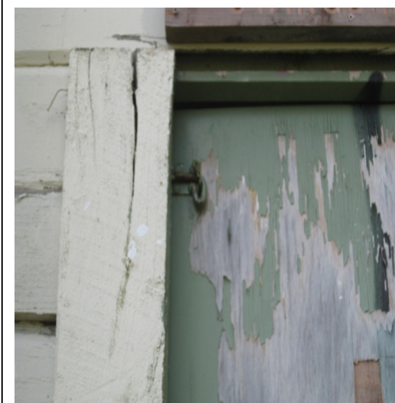
Photo 33: Longitudinal crack in timber element on south wall.
