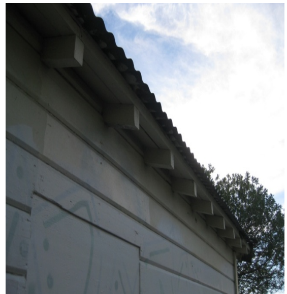
Photo 38: East soffit with corrugated metal roof sheeting above 80x50mm timber rafters at 450mm centres.
