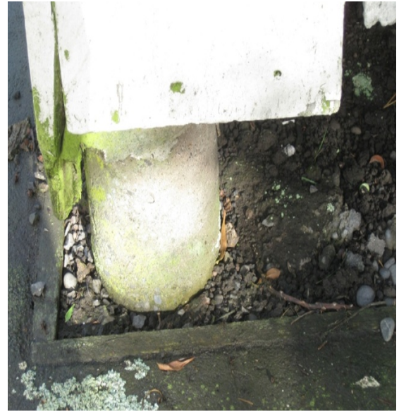
Photo 10: 150mm diameter concrete pile on northeast corner of building.
