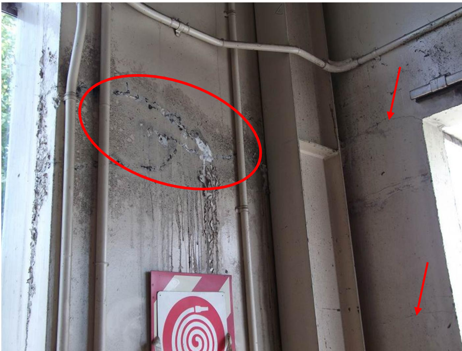
Photo 4: Cracks to concrete walls
