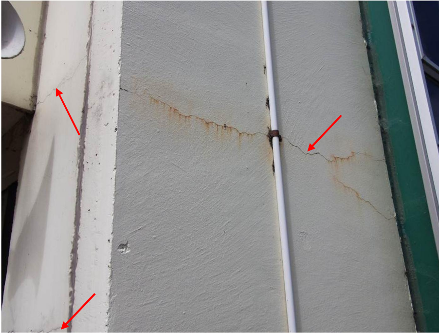
Photo 5: Typical cracking to concrete walls
