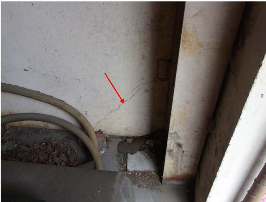
Photo 6: Typical cracking to concrete walls
