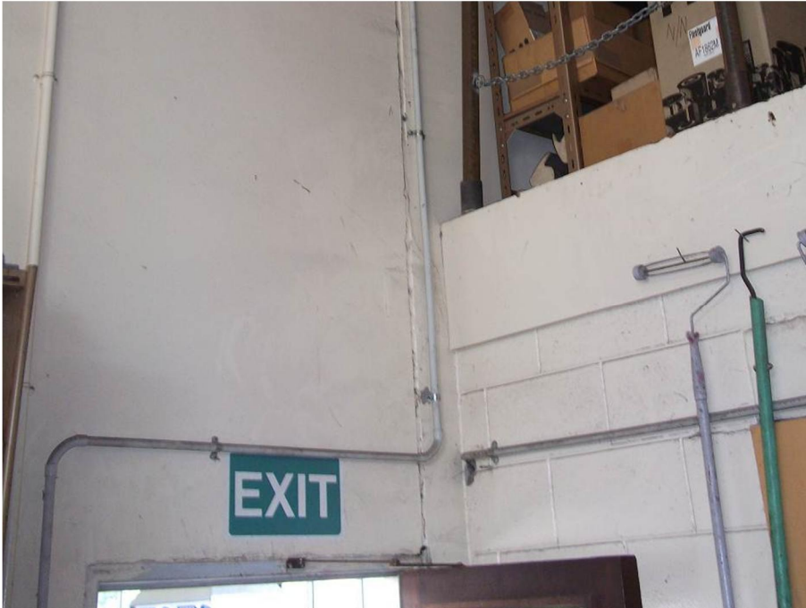
Photo 3: Typical cracking to vertical walls joints
