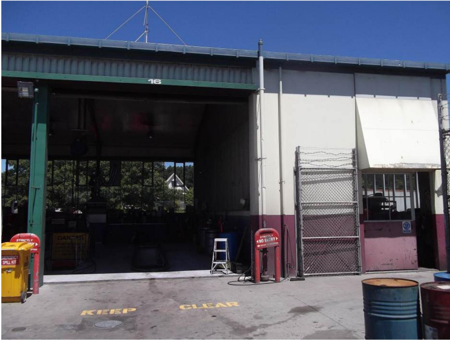
Photo 1: External view of Tyre Bay
