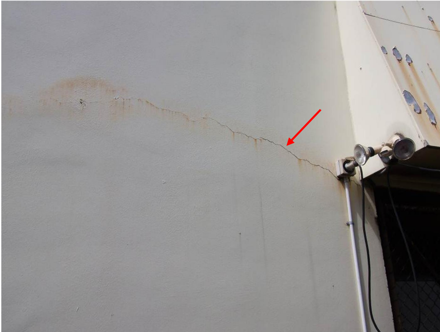
Photo 7: Typical cracking to concrete shear walls
