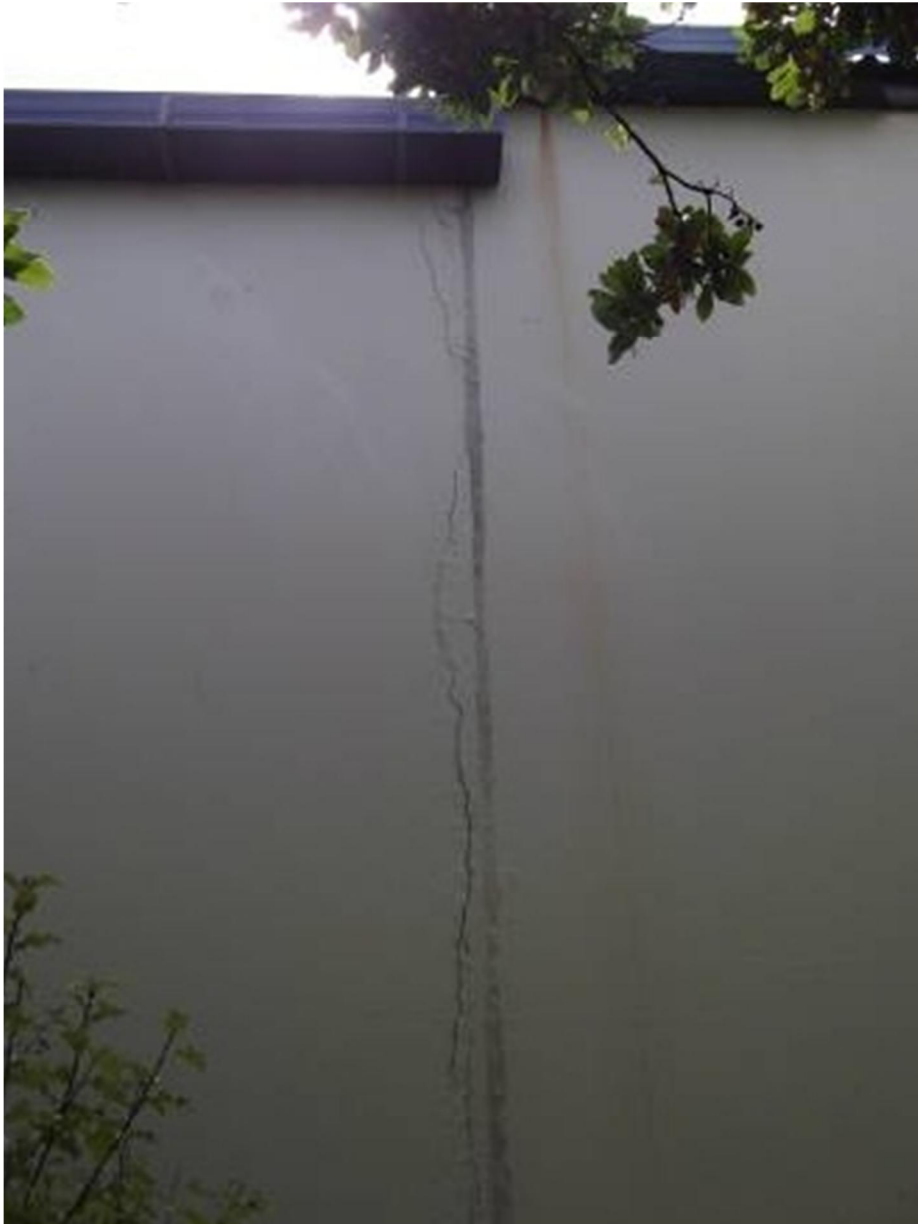
Photo 9: Cracking to concrete wall panel
