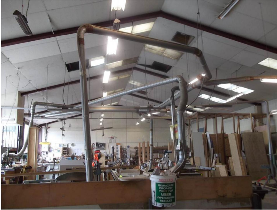
Photo 5: Interior view of Building Services Workshop
