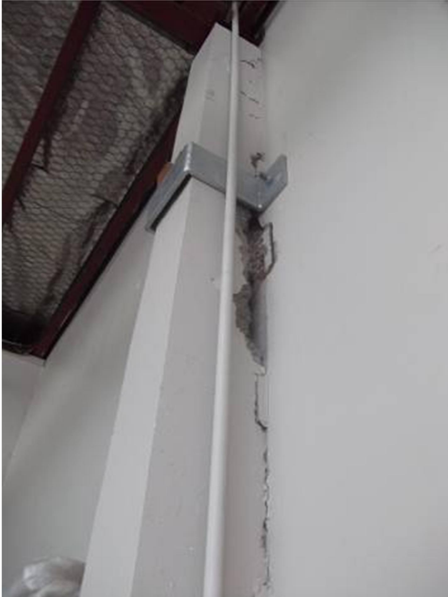
Photo 7: Damage to column encasement
