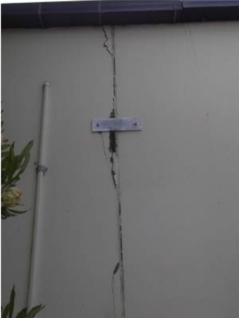
Photo 8: Damage to wall on other side of Photo 7.
