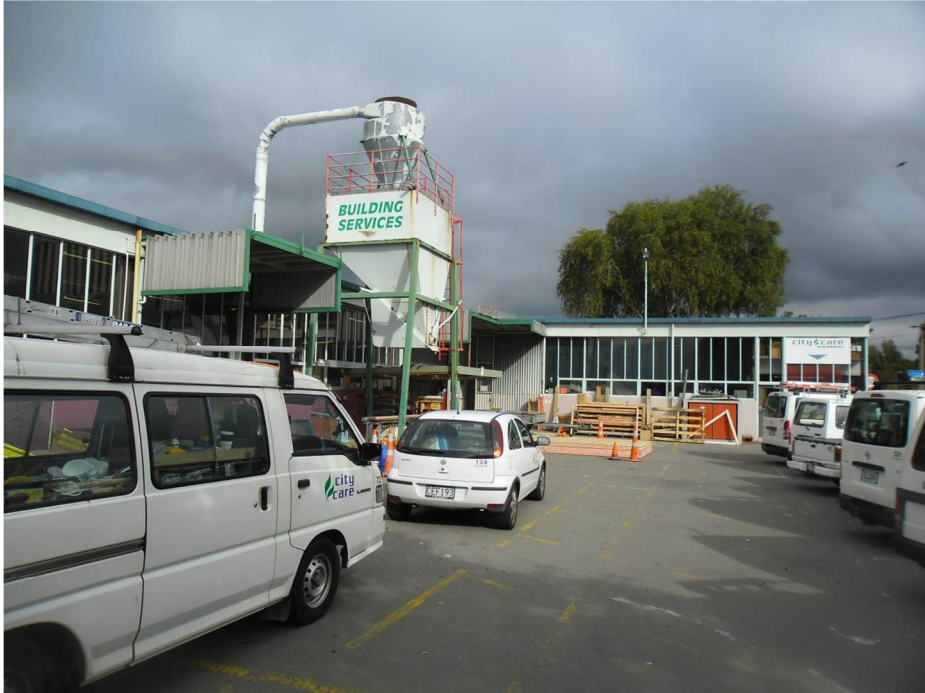
Photo 1: Exterior view of Sign Shop and Building Services Workshop (North-west elevation)
