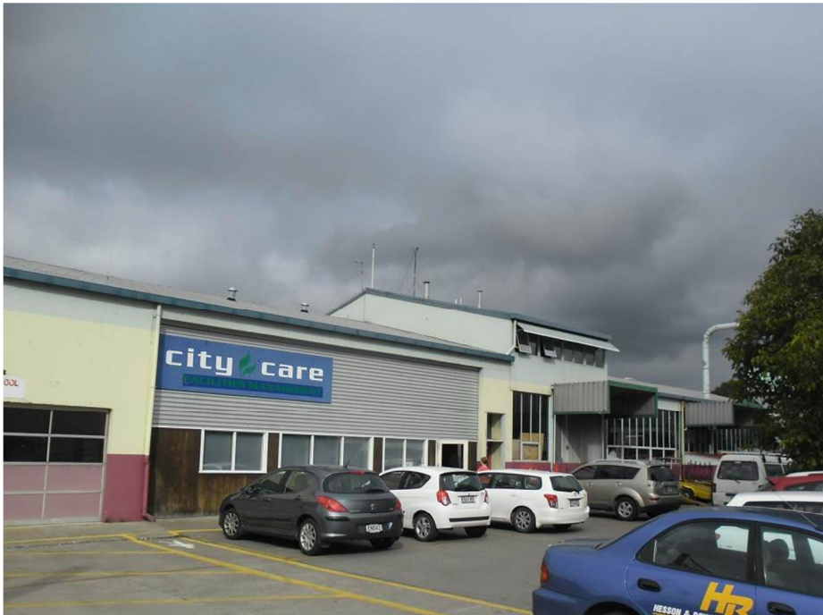
Photo 2: Exterior view of Facilities Management (North elevation)
