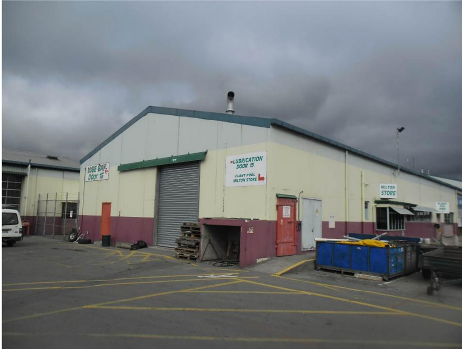
Photo 3: Exterior view of Hire Pool / Storage / Weed Spraying areas (North-east elevation)
