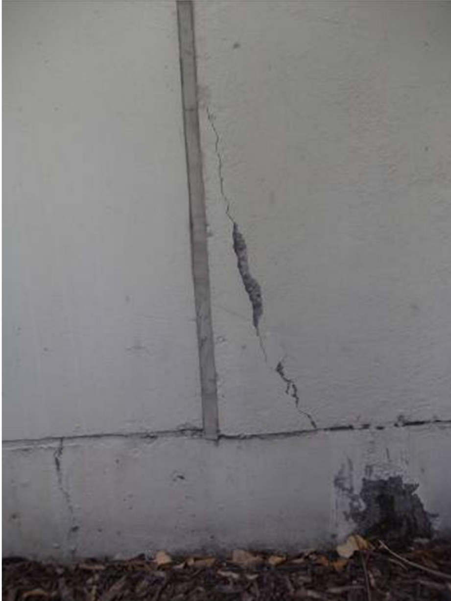
Photo 10: Typical cracking to concrete wall panel
