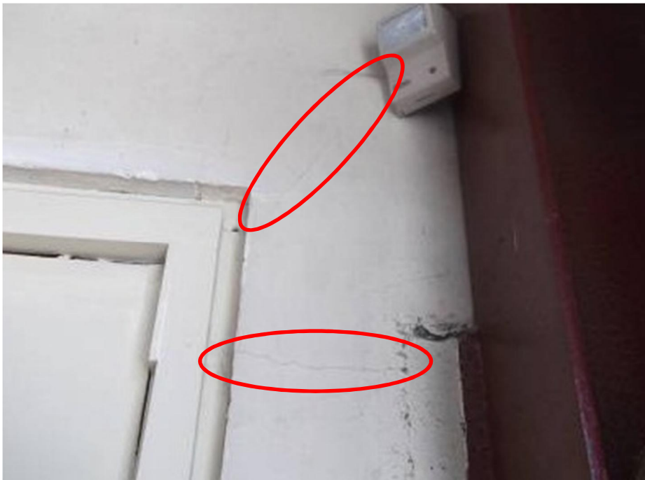
Photo 14: Cracking to concrete wall
