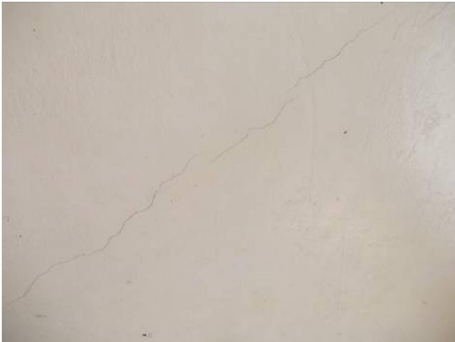
Photo 12: Cracking to concrete wall
