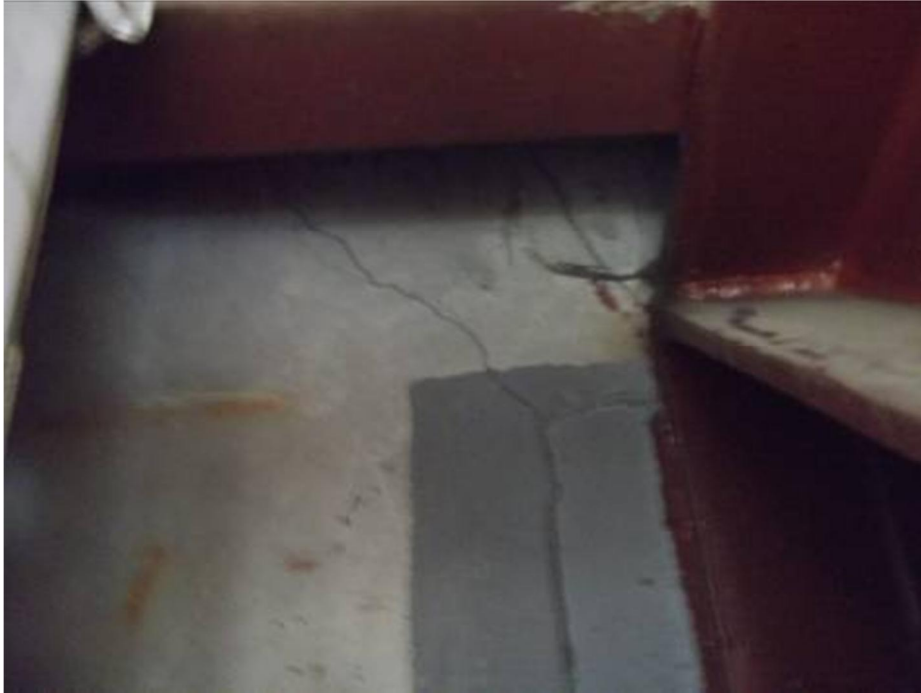
Photo 11: Typical cracking to concrete wall panel
