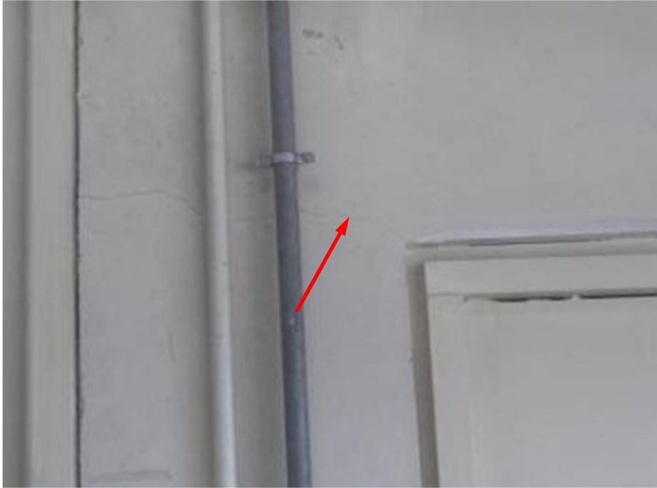
Photo 13: Cracking to concrete wall
