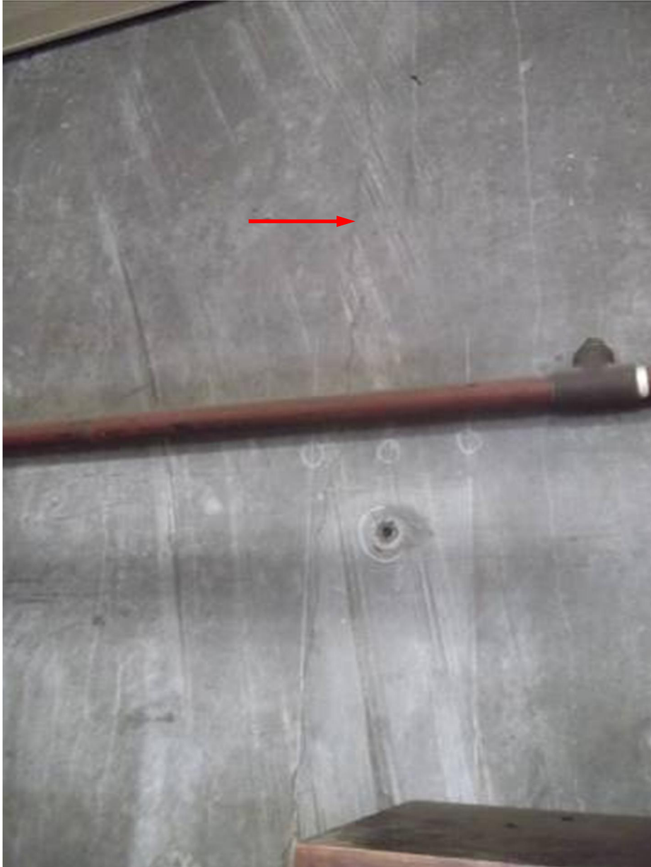
Photo 15: Cracking to concrete wall
