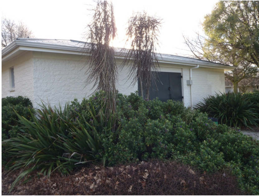
Photo 3: View of the rear of the building
