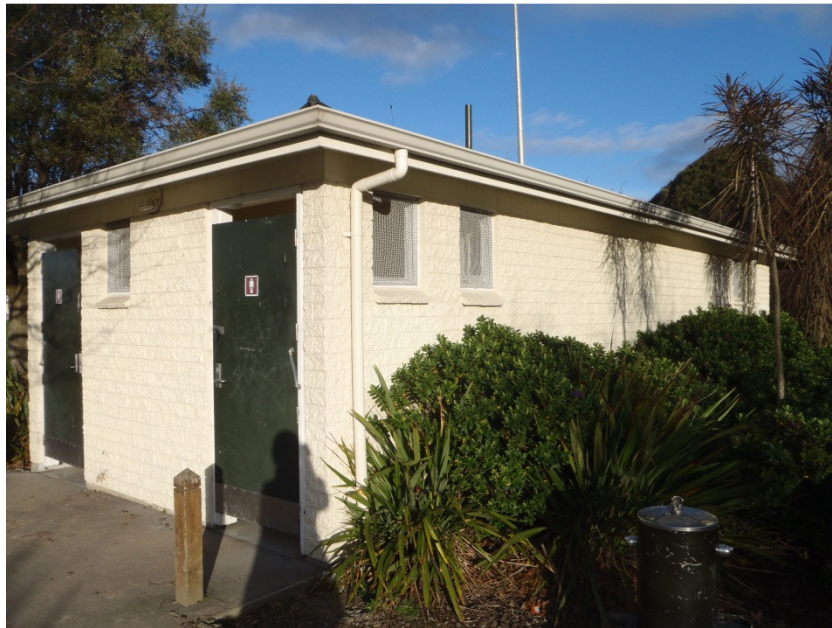
Photo 1: View of the front of the building
